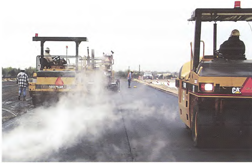
Construction crews working on an airport runway.
