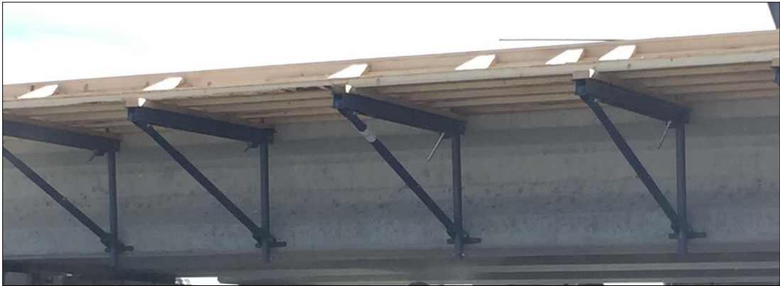
(b) Forming of the overhang portion of the deck
