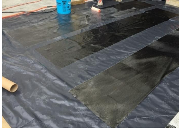
(l) Saturating the CFRP with Sikadur 300
