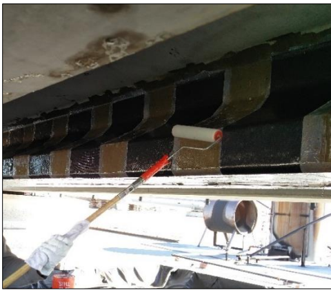
(a) Application of Sikadur 300
