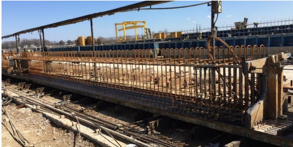
Figure 4-1 Strands and reinforcements cage
