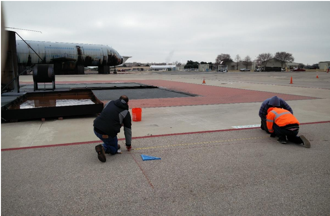
Figure 4-11 Construction layout and staking survey
