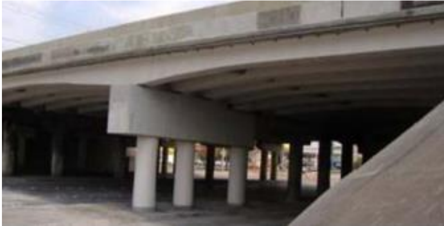
Figure 1-5 SH183 bridge over Macarthur Boulevard after FRP repair (Sika Corporation)
