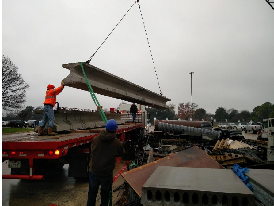
(a) Transportation of the support girders from CELAB to the fire test center
