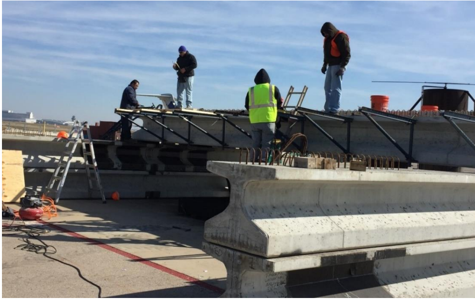
(a) Installation of hangers
