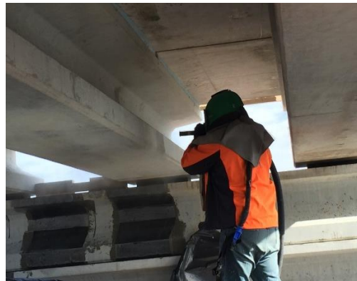
(c) Sandblasting unit (left) and operation (right)
