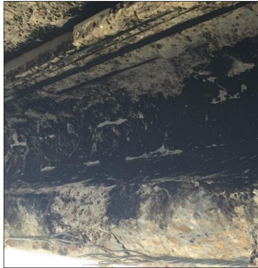
(a) Concrete hanging on the broken strand (b) broken strand
