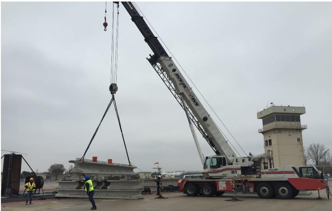
(d) Setting of the girders on the support
