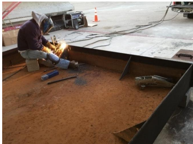
Figure 5-6 Welding of additional stiffeners
