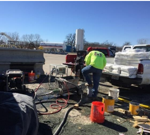
(c) spraying unit(left) and mixing of Sikacrete-213F (right)
