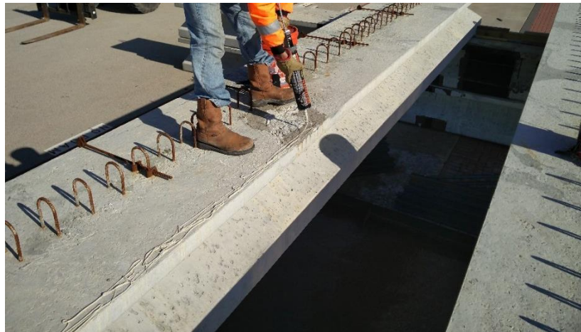
(a) Spreading of epoxy on the edge of the girder
