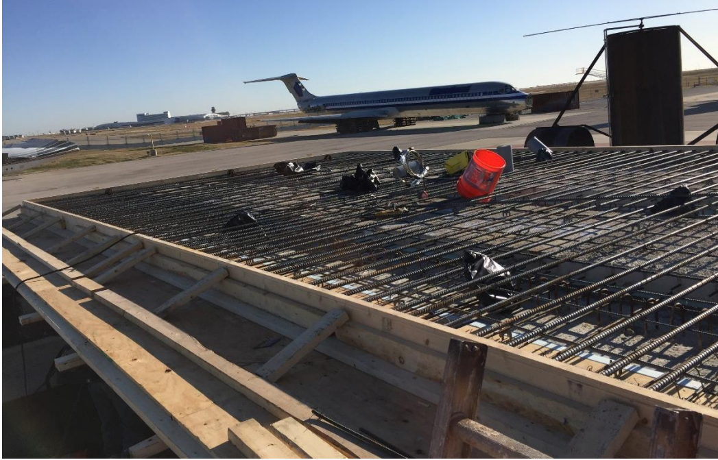
(c) Deck reinforcement
