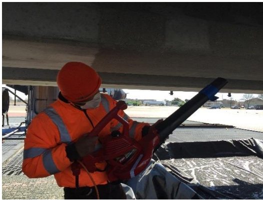
(h) Pressurized dust removal
