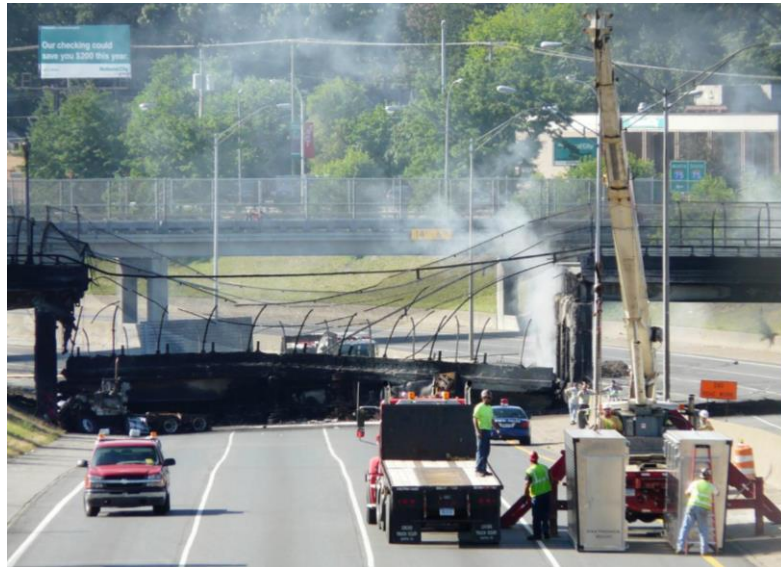
Figure 2-1 The collapsed Hazel Park Bridge near Detroit, Michigan (Wojdyla 2009)
