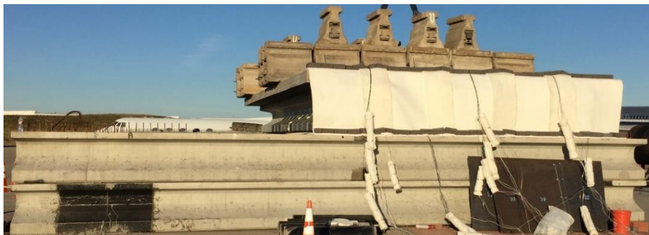
(b) Opening between girders after placing the ceramic blanket
