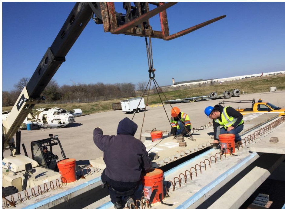
(c) Placing of precast deck panels
