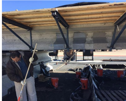
(k) Applying Sikadur-330 on the concrete
