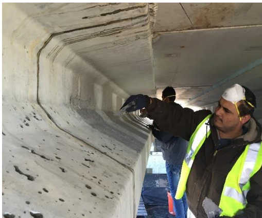
(j) Patching of voids using Sikadur 30
