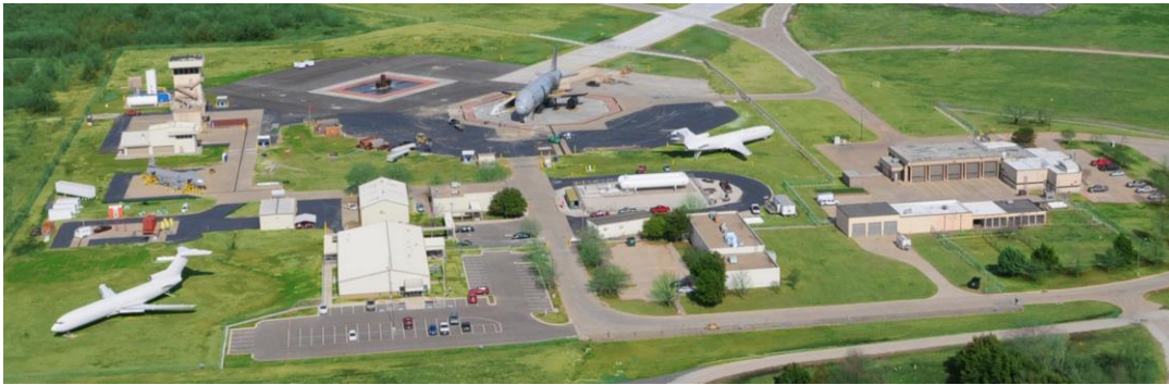
Figure 4-8 The Dallas/Fort Worth International Airport's Fire Training Research Center
