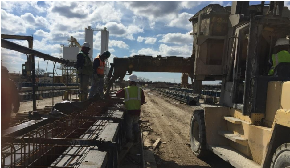
Figure 4-3 Concrete casting of girders
