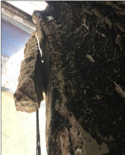
(a) Concrete hanging on the broken strand (b) broken strand
