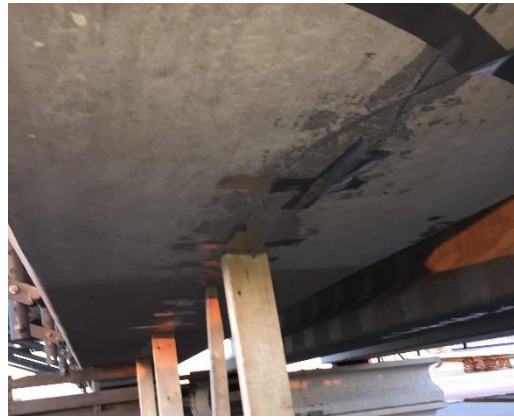
(g) Installed thermocouple
