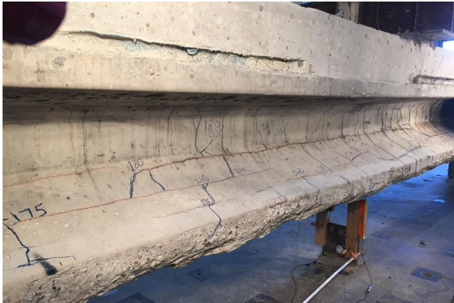
Figure 6-33 Cracks formed during fire and residual strength test
