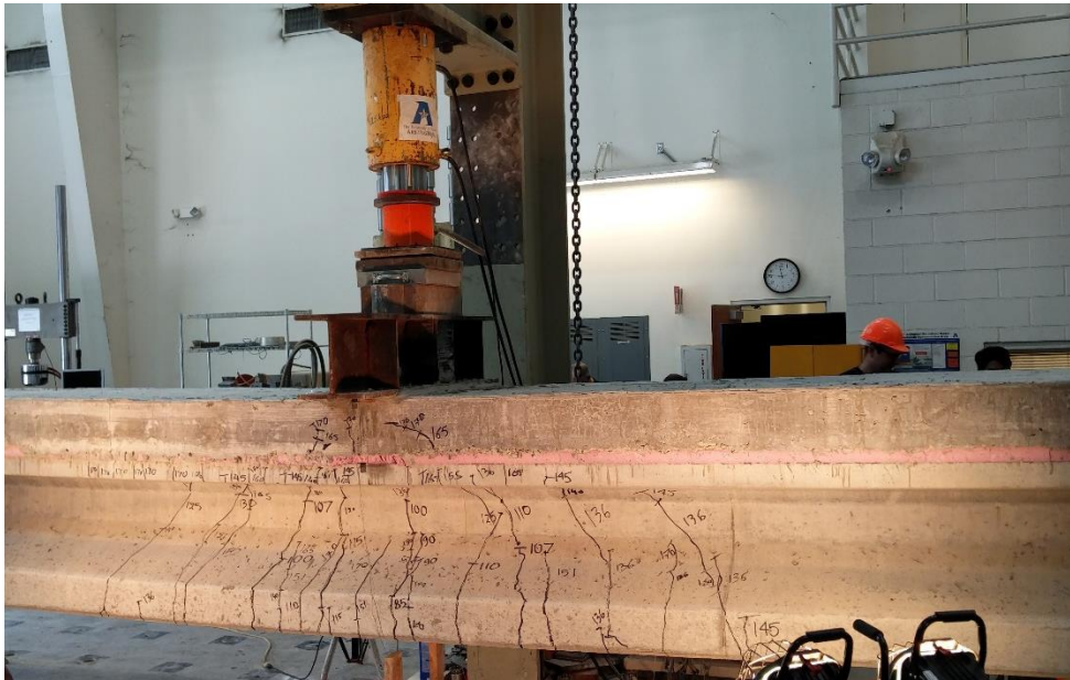
Figure 6-41 Crack pattern of control girder
