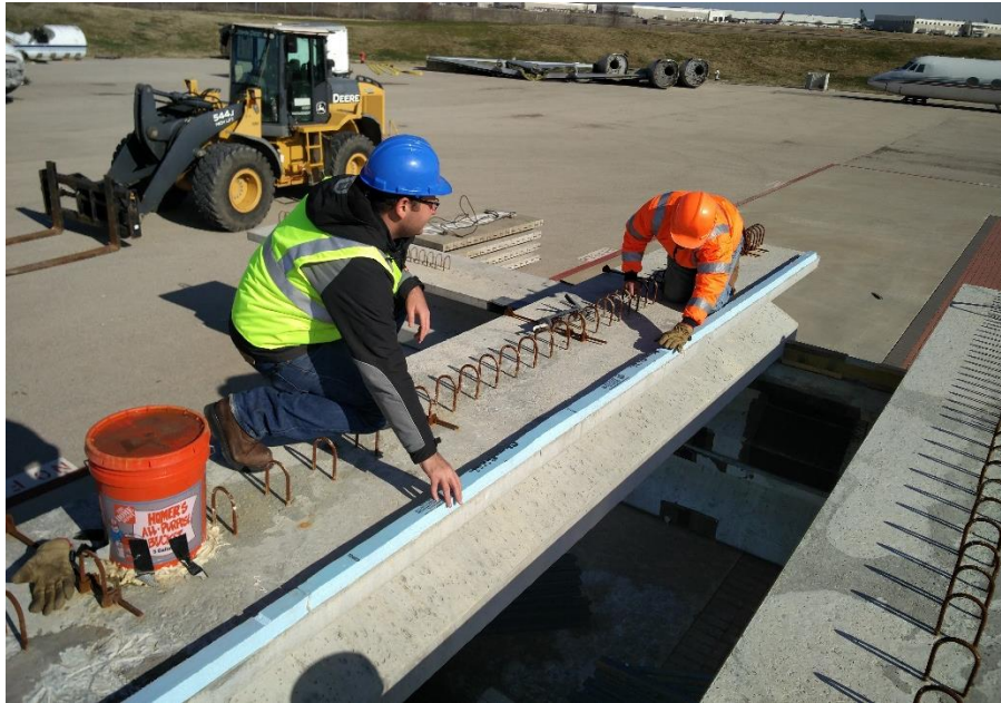
(b) Placing of bedding strip
