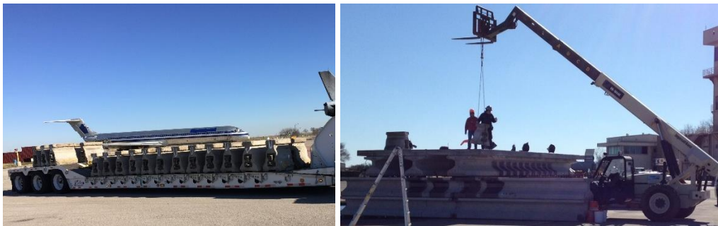
Figure 5-2 Loading of zipper barriers
