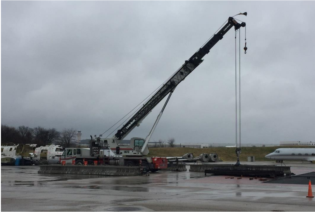
(C) Setting of the support girders to the ground
