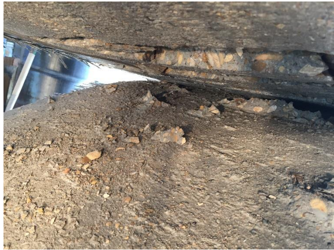
(b) small chunks of concrete on the debonded FRP
