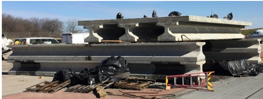
(a) Opening between girders before placing the ceramic blanket
