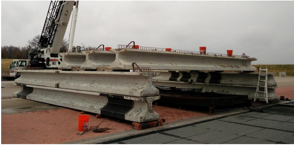
(e) Supports and girders after placement
