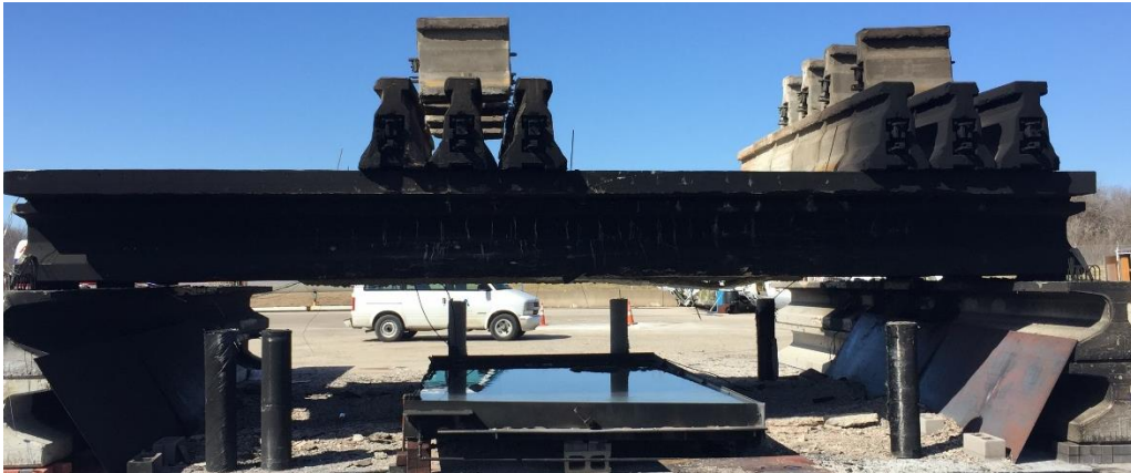
Figure 5-53 Girder-3 covered with soot
