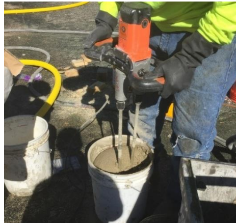
(c) spraying unit(left) and mixing of Sikacrete-213F (right)
