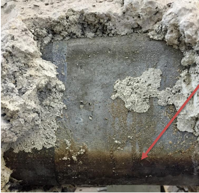
Figure 5-27 Smoke on the concrete underlying the fireproofing
