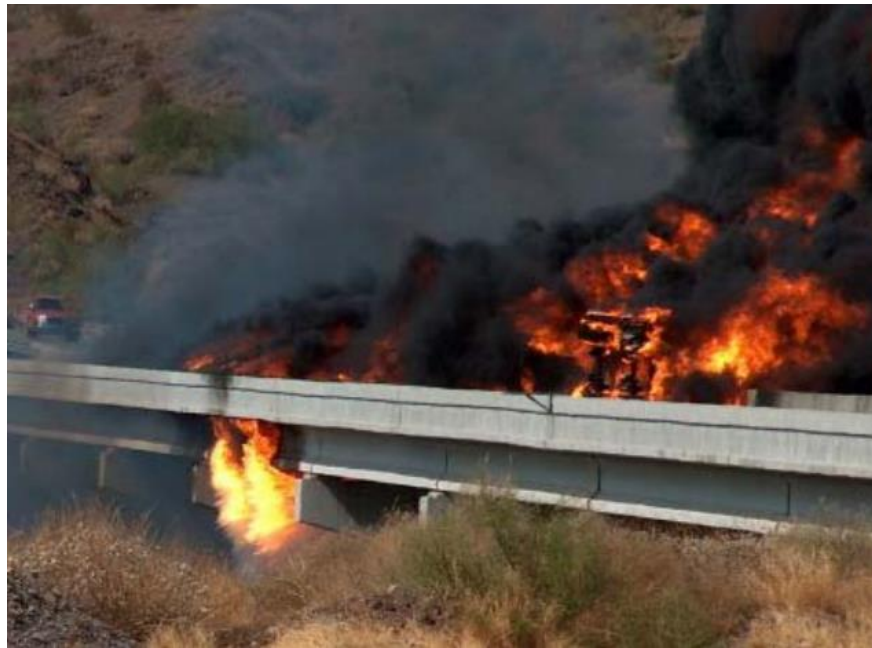
Figure 2-3 Bill Williams River Bridge fire (Marth et al. 2007)
