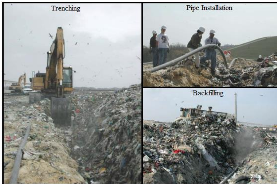
Figure 2.6 Construction of the horizontal trench (Townsend, T., 2008)
