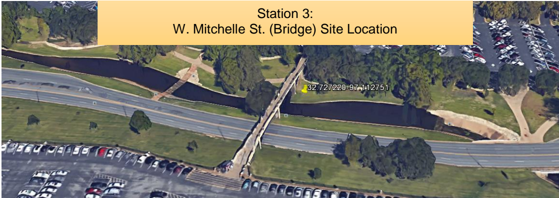
Figure 3-4 Aerial View of W. Michelle St. (Bridge) Site Location of Station 3
