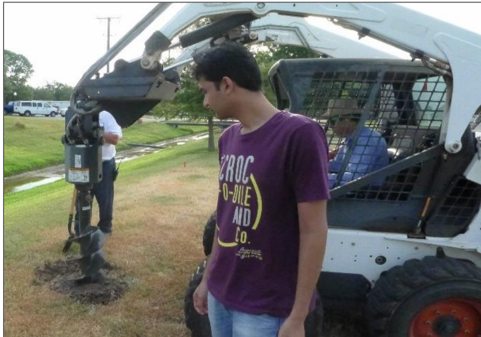
Figure 3-35 Rotatory Drill Auger Excavator employed for excavation
