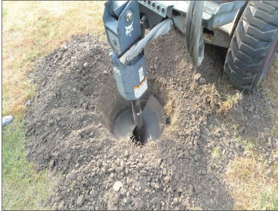
Figure 3-36 Soil Excavation using Rotatory Drill Auger Excavator
