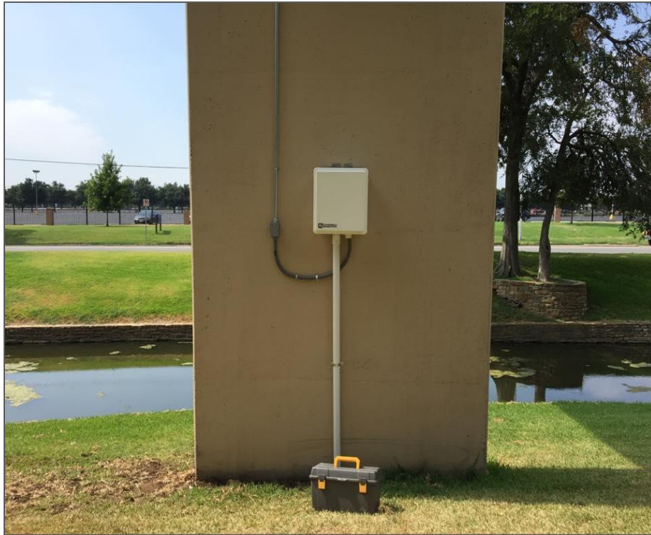
Figure 3-51 The whole assembly for the TDR installation and measurement is complete.
