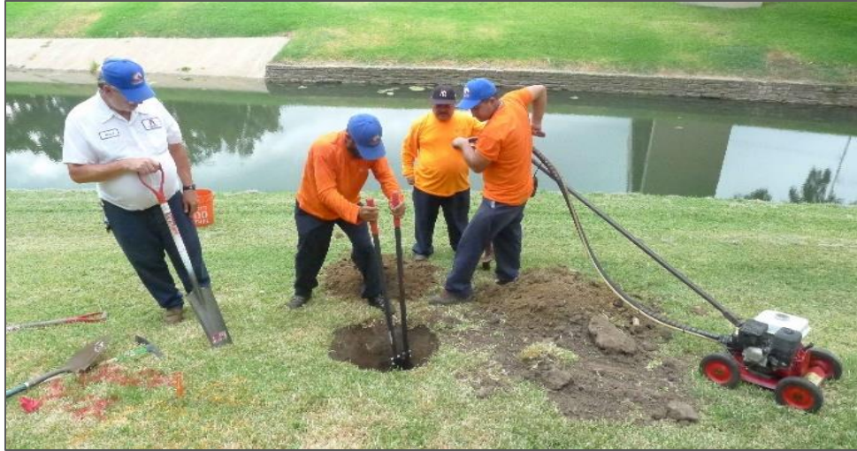
Figure 3-38 Hand Augers and Auger Drills operated by DG in sloping ground
