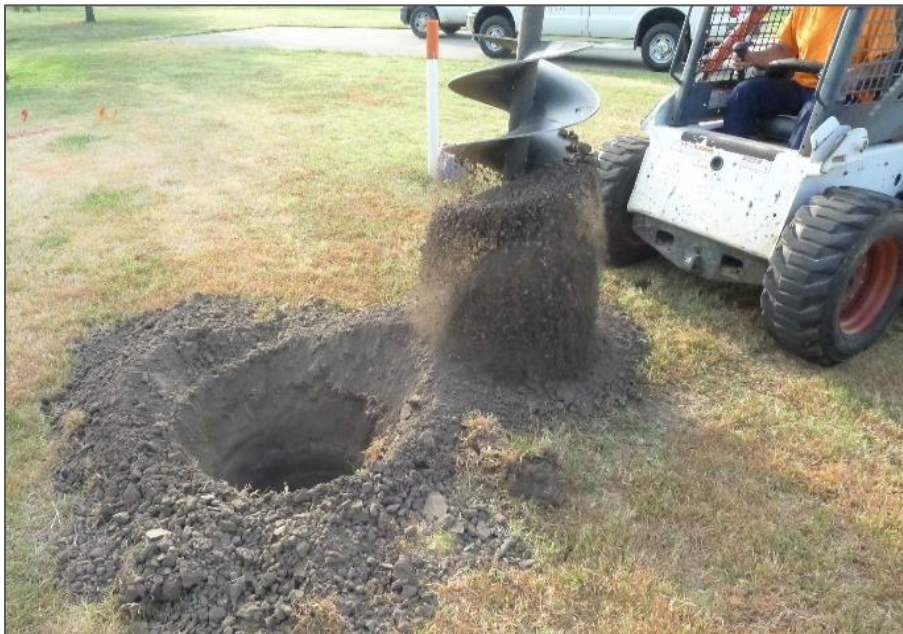
Figure 3-37 Soil Excavation using Rotatory Drill Auger Excavator
