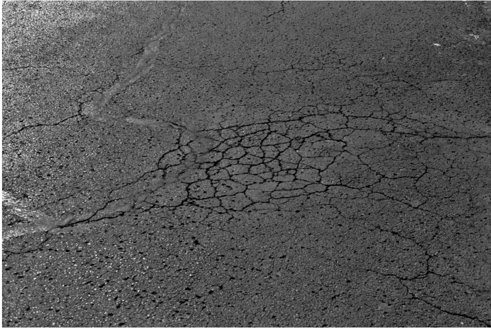
Figure 1-1 Alligator Cracking (Asphalt Institute, 2016)
