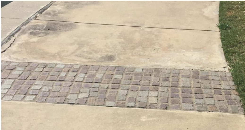
Figure 4-23 Brick and Concrete Paving 2
