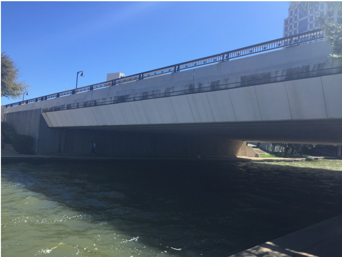
Figure 4-26 Bridge over Lake Carolyn
