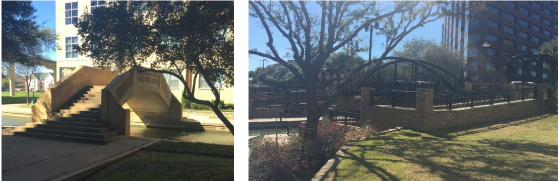
Figure 4-25 Bridge over the Mandalay Canal
