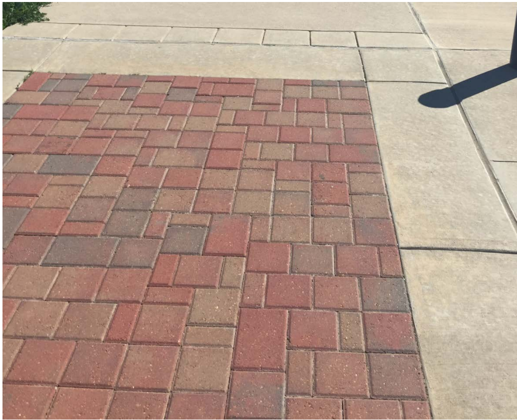
Figure 4-22 Brick and Concrete Paving
