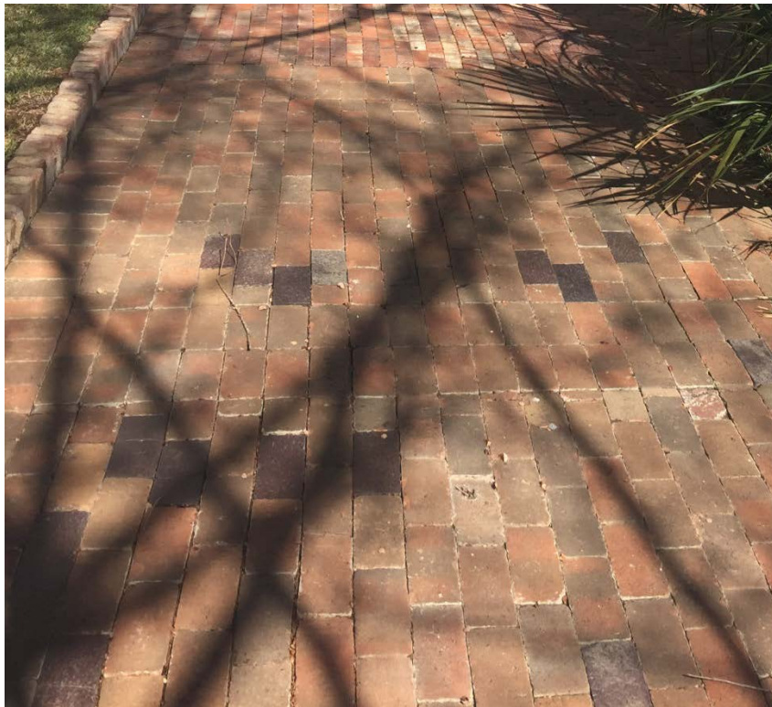
Figure 4-20 Red Brick Paving
