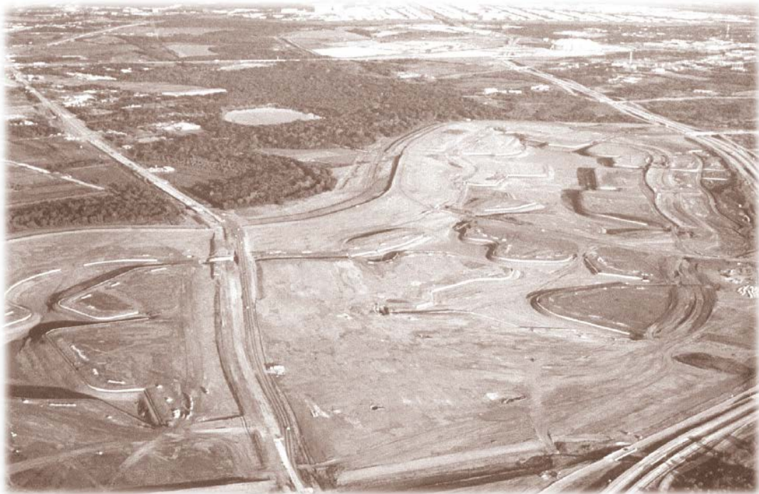
Lake Carolyn during the initial phase of excavation.
