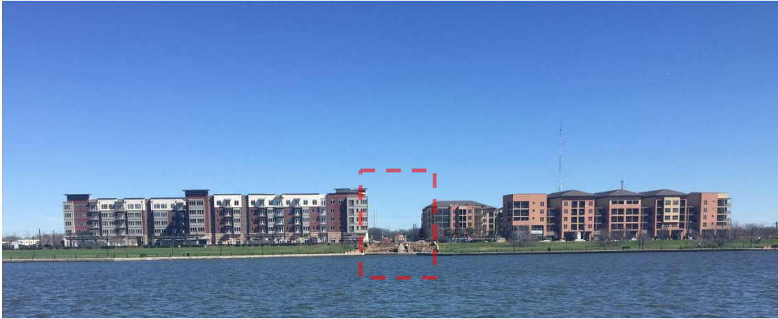
Figure 4-10 Buildings Framing the View
