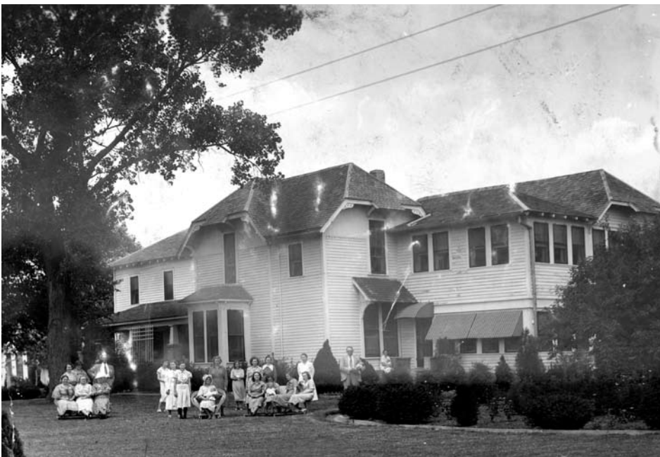
The historic main Rest Cottage building. The facility stood amidst 70 acres of gardens and hay pastures that produced fruit, vegetables, milk and beef for consumption on site.
