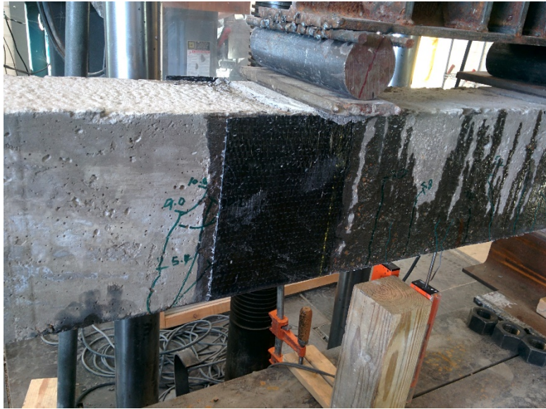
Figure 34 Crack pattern for strengthened beam with U-Wrap
