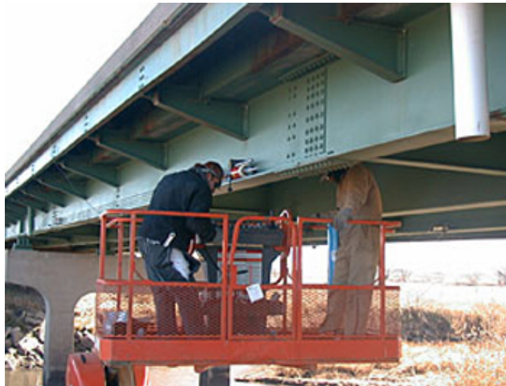
Figure 2: Strengthening of Steel Bridge
