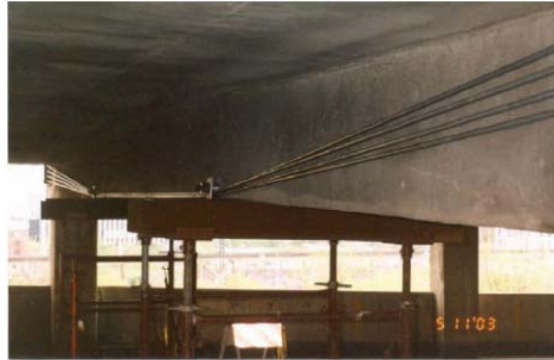
Figure 9: External Post-tensioning
