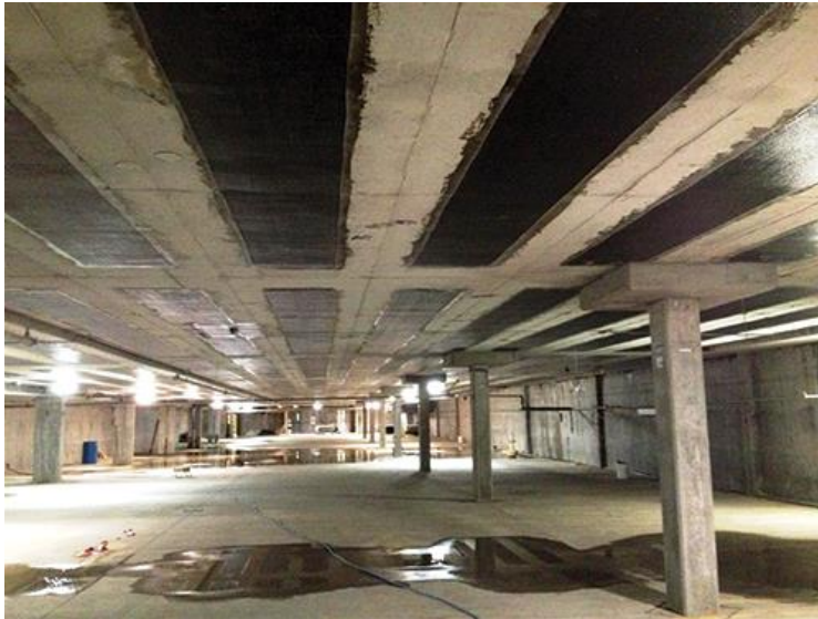
Figure 3: V-Wrap composite sheeting
