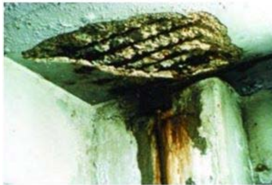
Figure 8: Corrosion
