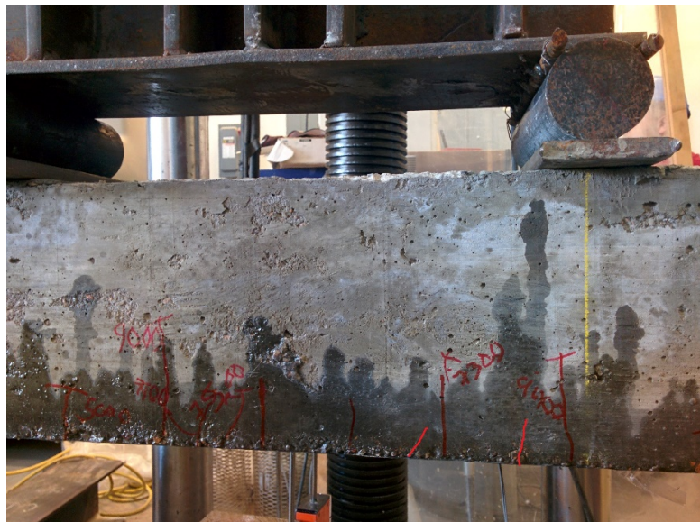
Figure 33 Crack pattern for Strengthened beam with anchor bolt
