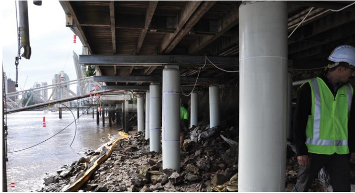
Figure 1: Strengthening of Piles using FRP
