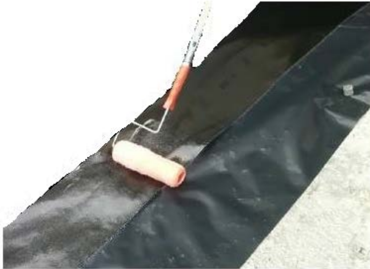
Figure 21: Saturate the FRP sheet
