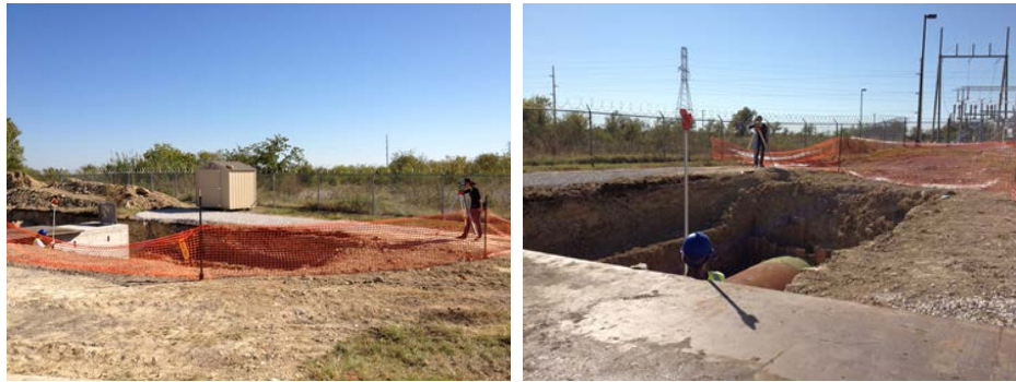
Figure 4-9 Surveying was conducted in order to obtain the exact trench configuration
