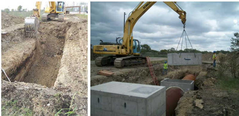
Figure 4-7 The excavated trench, installed pipes, and manholes
