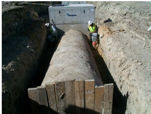
Figure 4-13 Compaction and backfilling of the select fill for the first pipe
