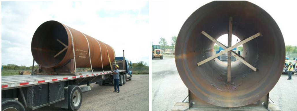
Figure 2-6 Stulls were installed in the manufacturer's plant to prevent excessive deformation
