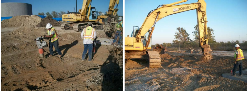
Figure 4-17 Final surface of the trench after completion of the backfilling
