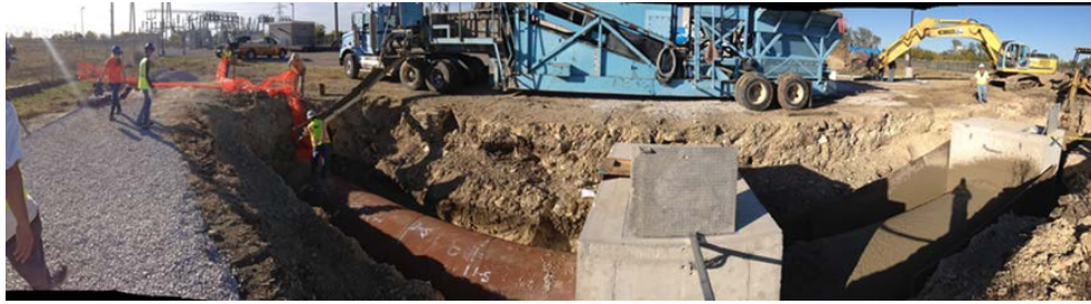
Figure 4-11 Preparation and casting of CLSM (panorama view)
