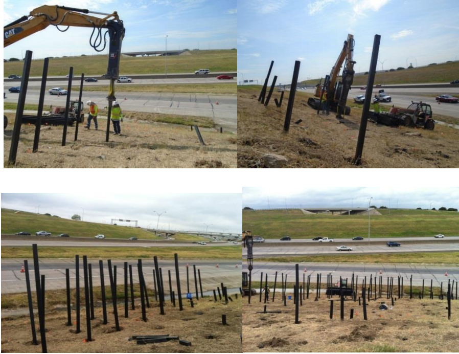
Figure 4-12 RPP Instillation at SH 183 Slope
