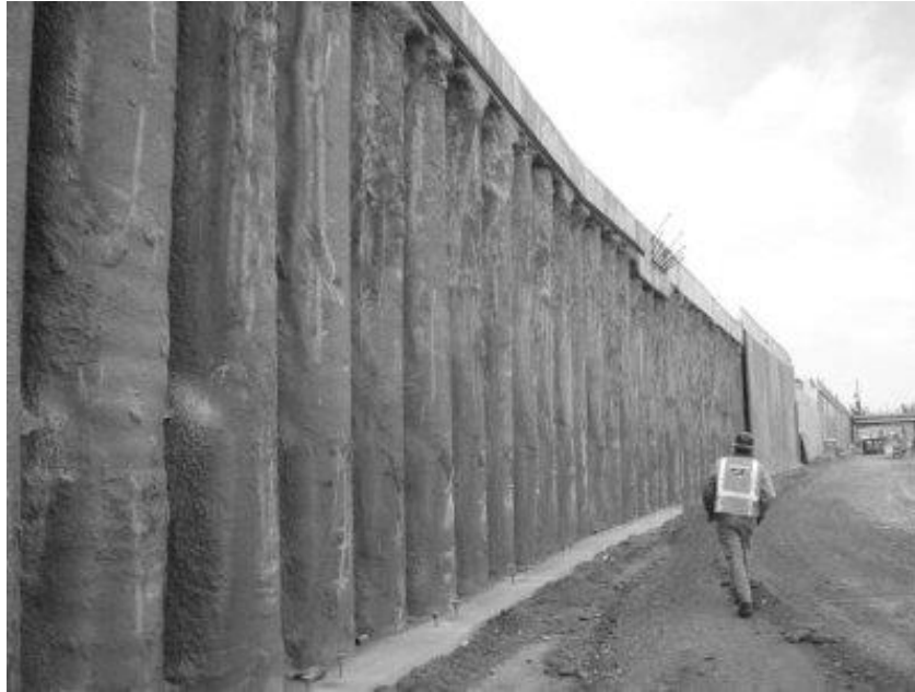
Figure 2-9 Construction of drilled shaft retaining wall. (Source fhwa.dot.gov)
