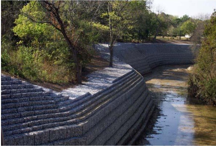
Figure 2-6 Gabion wall used to prevent erosion control in Desoto, Texas
