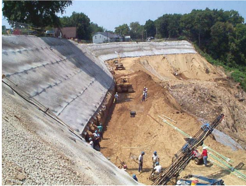
Figure 2-10 Soil nail after instillation (Source Wordpress.com)
