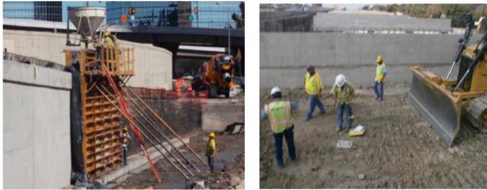
Figure 2-7 Cast in place wall placement and subgrade preparation (Quintanar, 2014)
