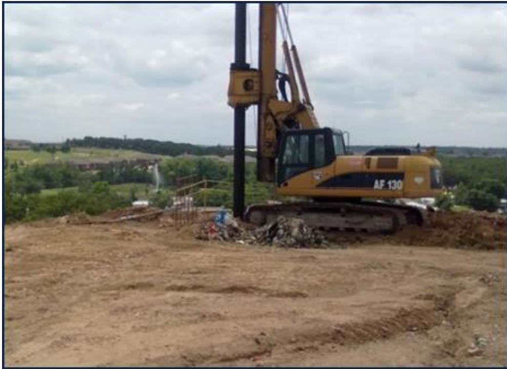
Figure 3-3 Landfilled MSW collection with AF 130 Hydraulic Drill Rig
