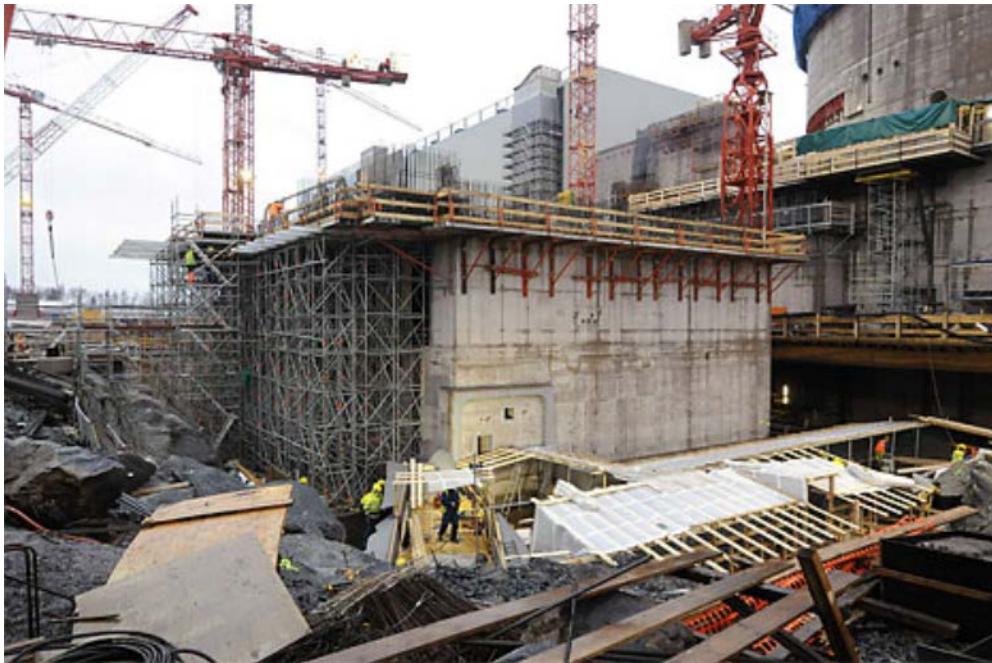
Figure 2-18 Shear wall in a nuclear reactor, Olkiluoto, Finland
