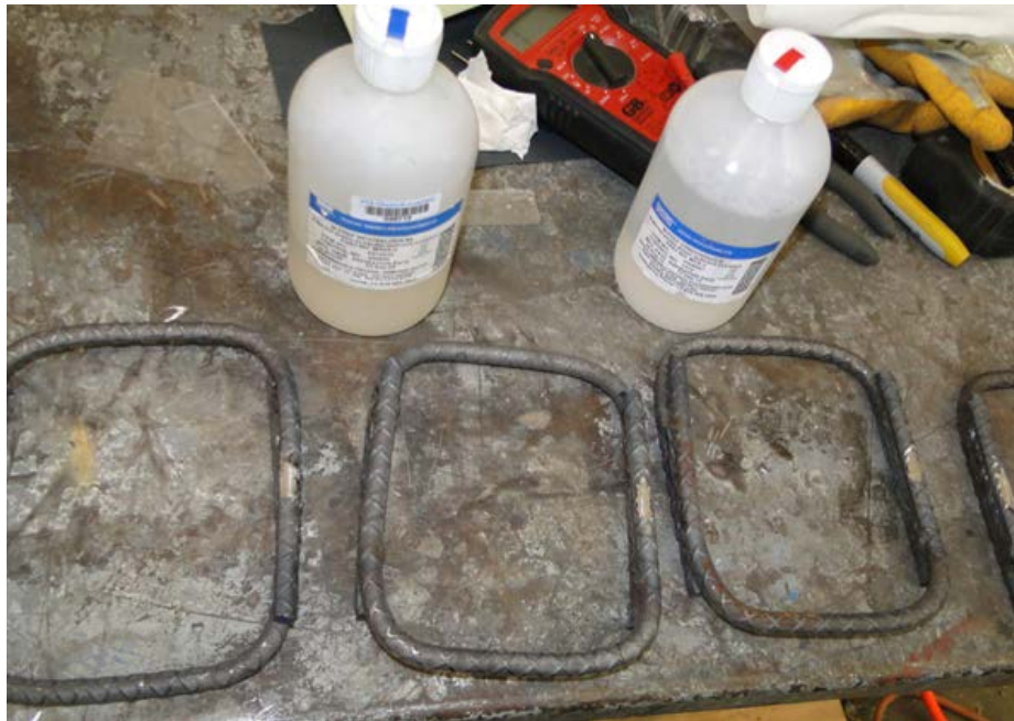
a) Smooth and clean the surface of the rebars
