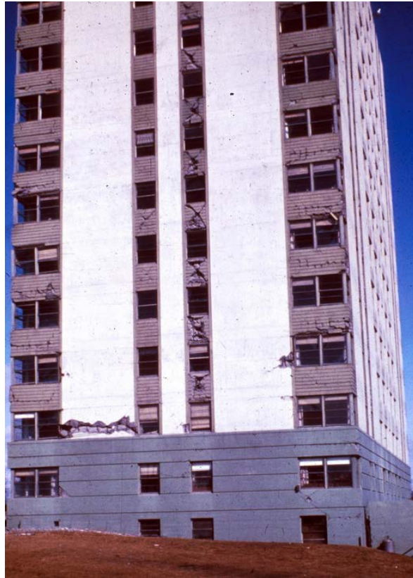
Figure 1-3 Diagram showing failure of conventional coupling beam during Alaska Earthquake (United States Geological Survey (1964))
