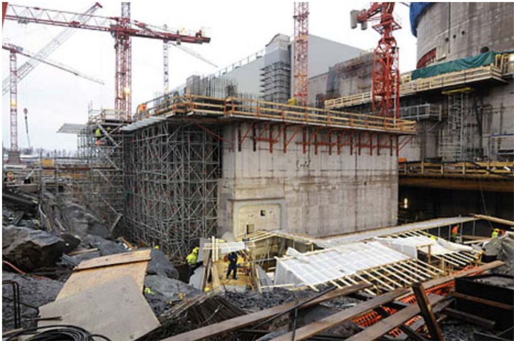
Figure 1-6 Shear wall in a nuclear reactor, Olkiluoto, Finland
