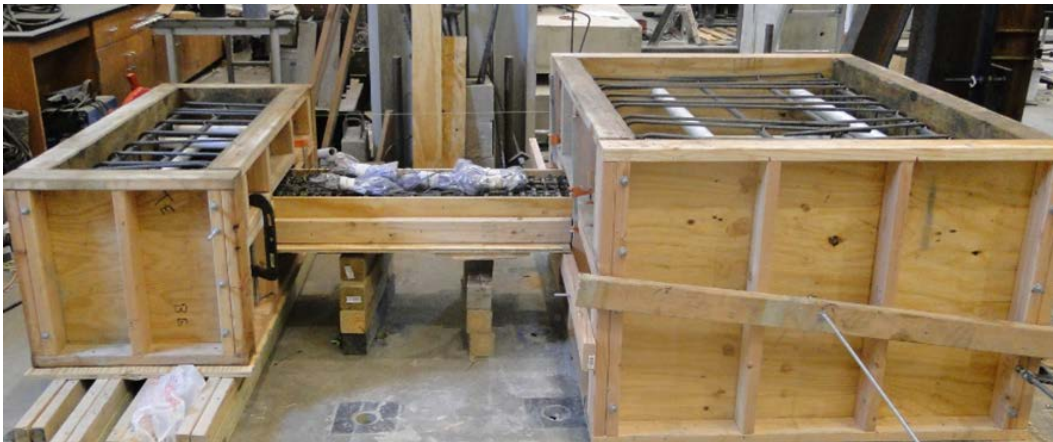
a) Construction Of half scale coupling beam
