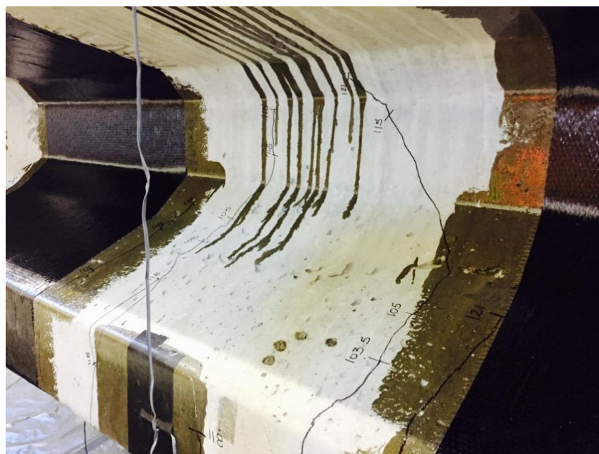
Figure 6-11 -Observed cracks due to loading GF1
