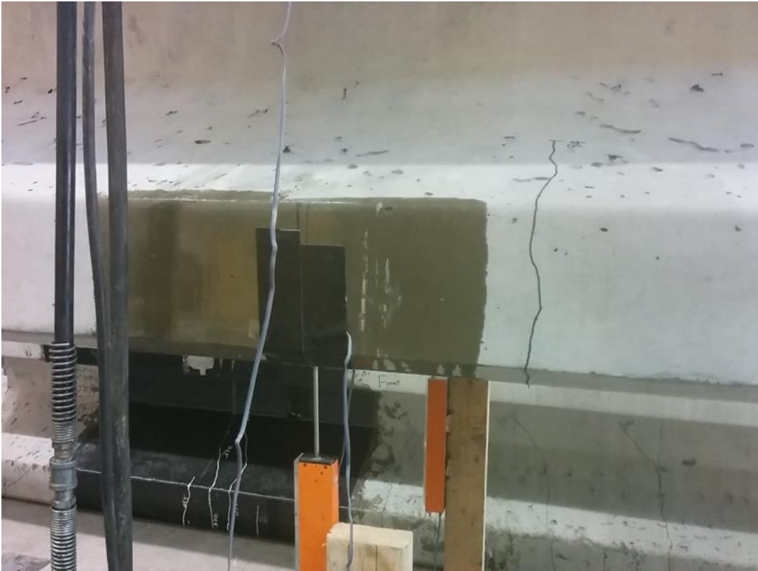
Figure 6-1- Observed first crack at 94 kips
