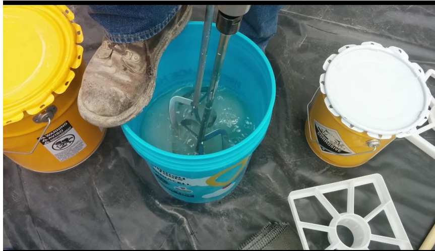
Figure 4-6- Mixing of epoxy
