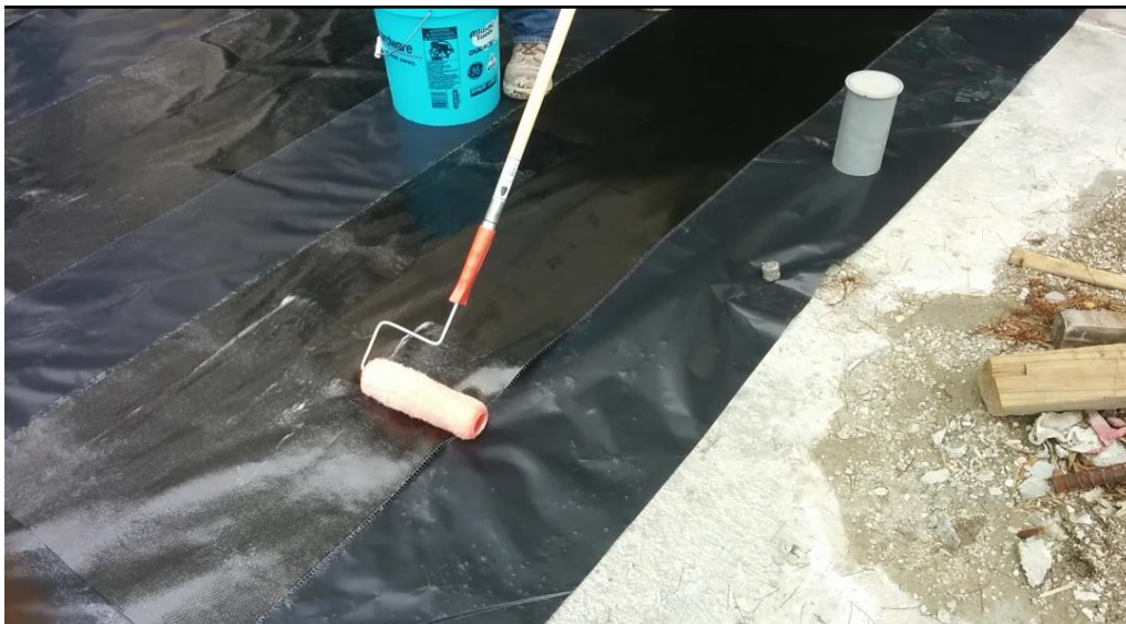
Figure 4-8 – Applying Epoxy on FRP
