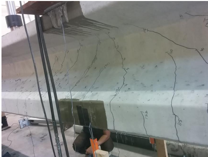
Figure 6-9 - Observed cracks due to loading at first force drop GC
