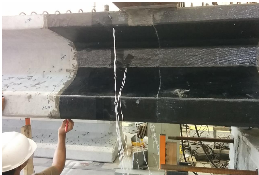
Figure 6-20 – Observed cracks due to loading GS1
