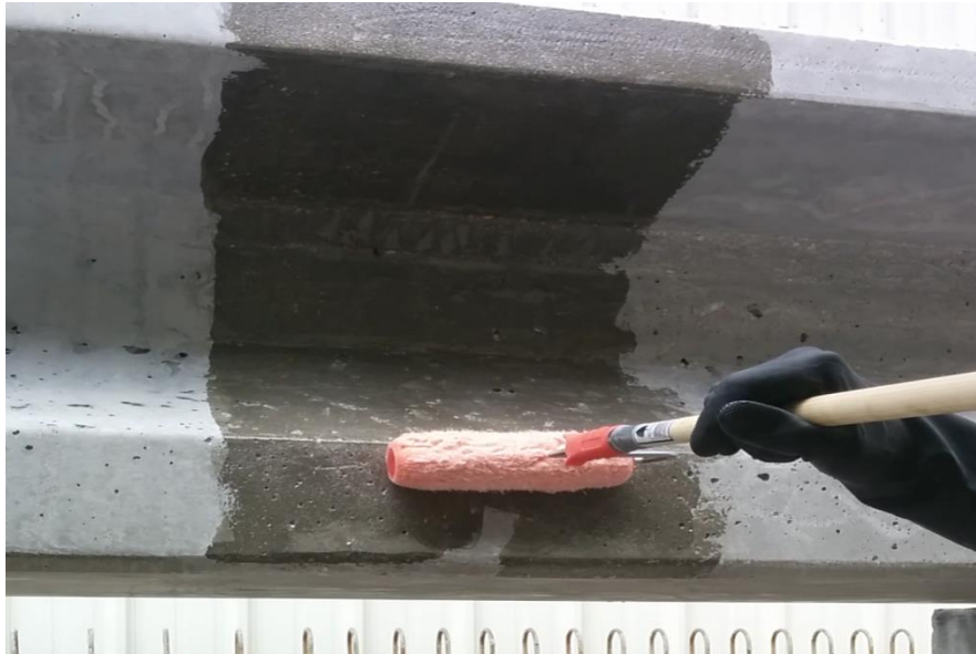
Figure 4-7- Application of epoxy to girders
