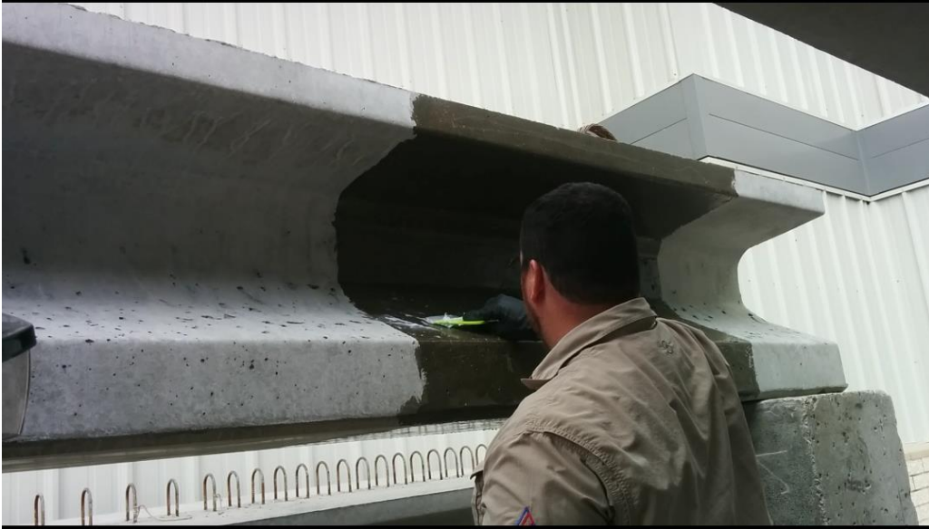
Figure 4-9 – Applying thick paste of Epoxy with Silica
