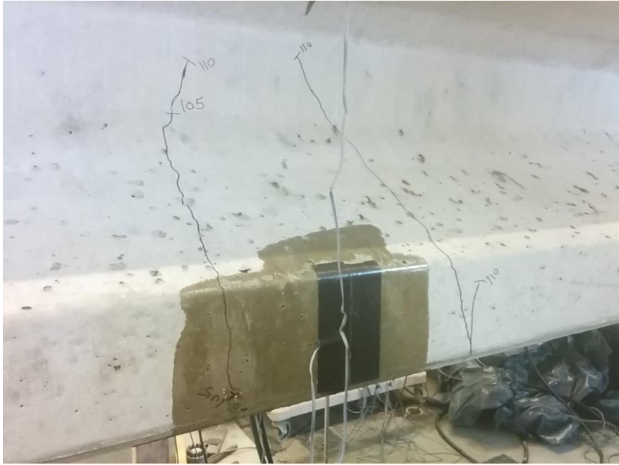
Figure 6-4 - Observed cracks due to loading GC
