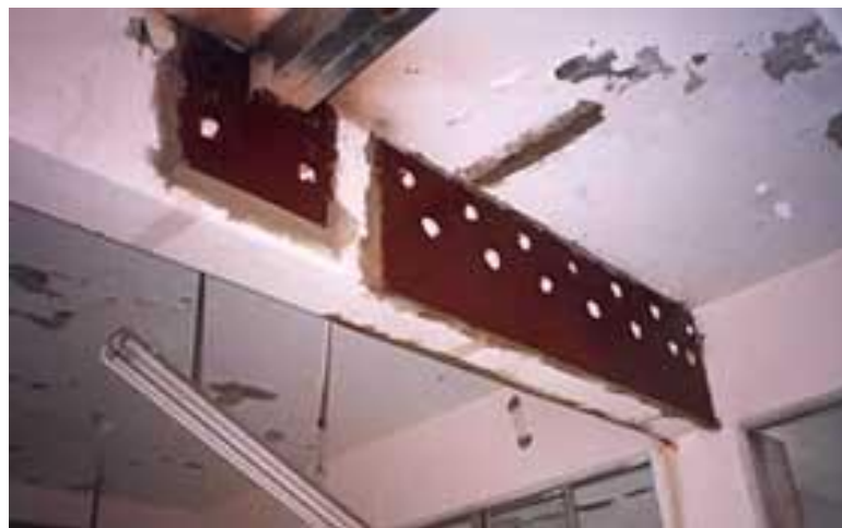
Figure 1-2 externally bonded steel plates ( www.chemcosystems.com )
