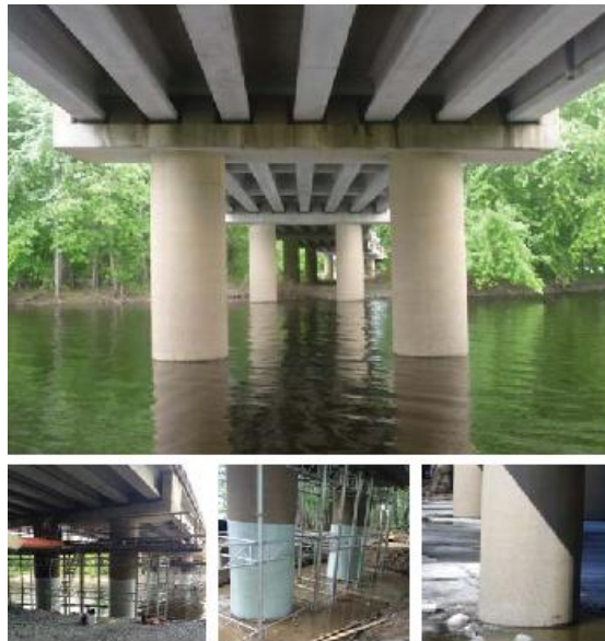
Figure 1-5 Nashwaak River Bridge in Fredericton, New Brunswick, Canada
