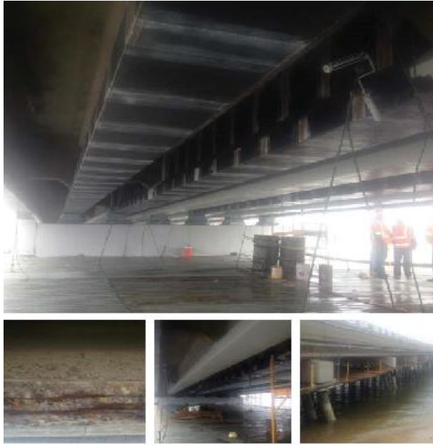
Figure 1-4 JFK bridge over Risley Channel in Atlantic country, New Jersey
