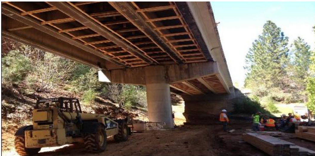
Figure 1-7 FRP girder strengthening for Caltrans big oak side hill viaduct
