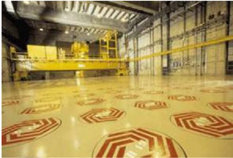
Figure 2-17 Storage hall for vitrified waste at La Hague
