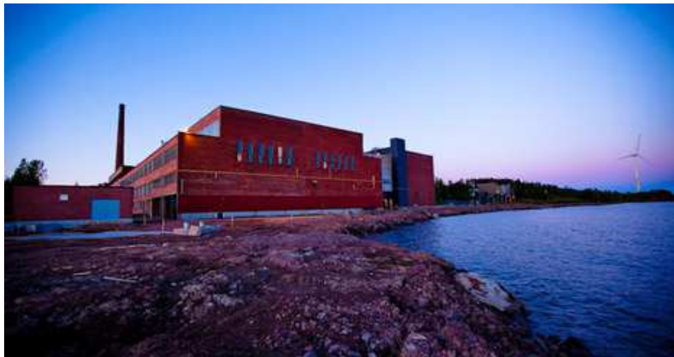
Figure 2.3 Google's Hamina Data Center cooled by sea water
