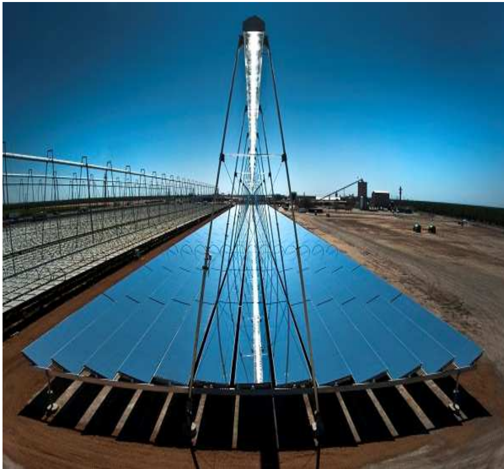
Figure 2.9 Linear Fresnel Reflector
