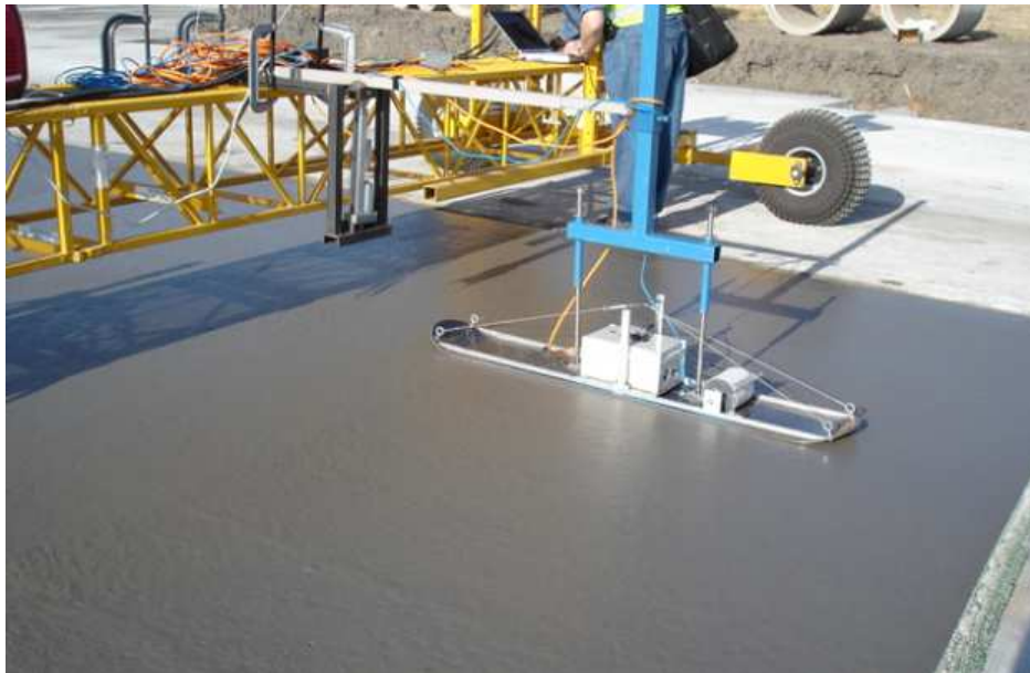
Figure 1-1 Sliding Profiler over wet concrete surface
