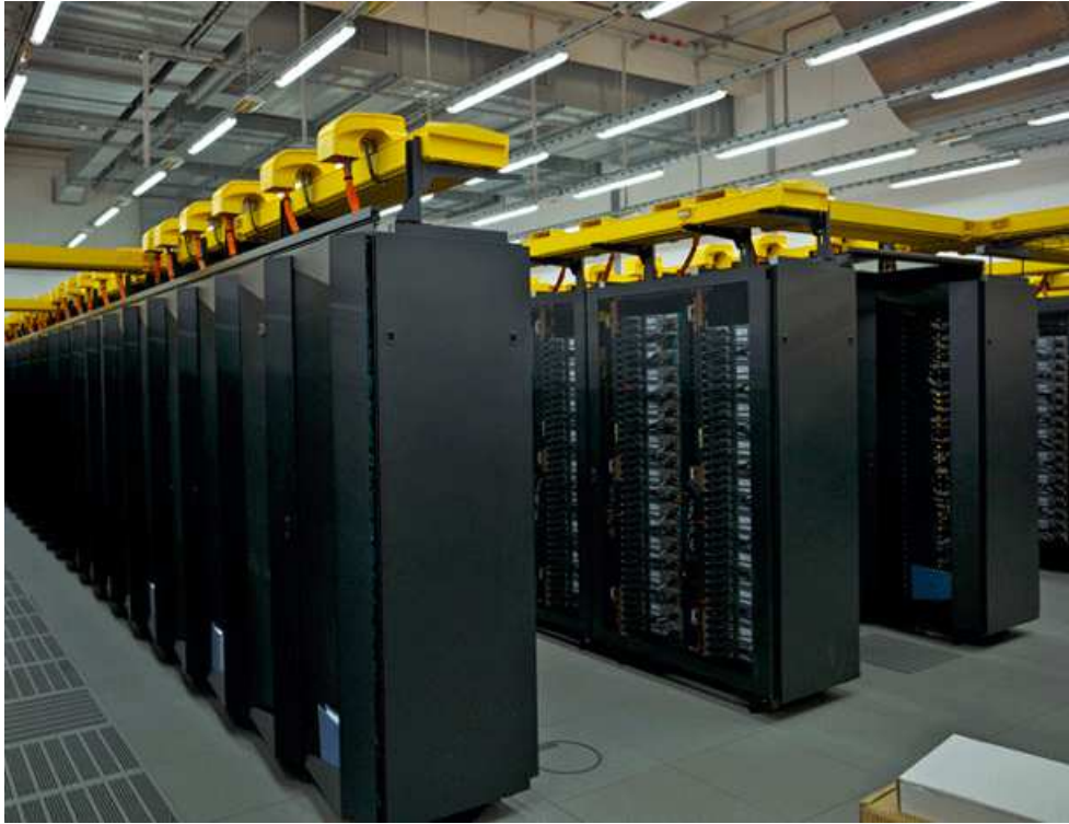
Figure 1.2. Liquid-based Cooling at IBM.
