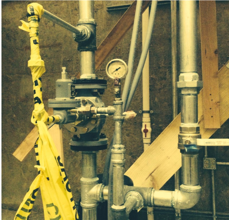
Figure 4.3 Back-Flow Pressure Valve
