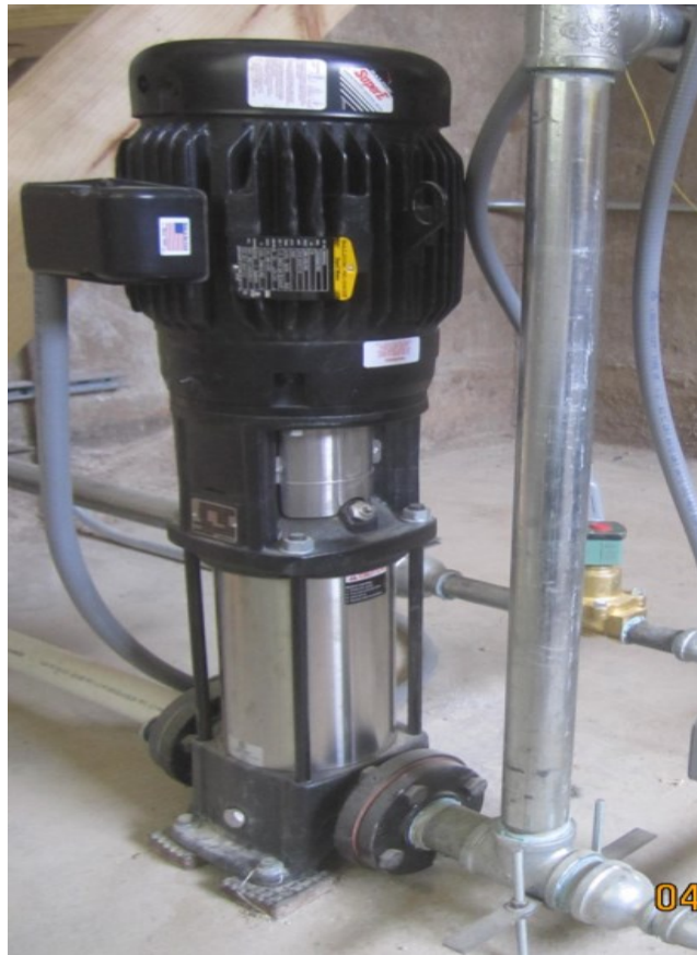
Figure 4.8 Multi-Stage Centrifugal Pump (10 HP)
