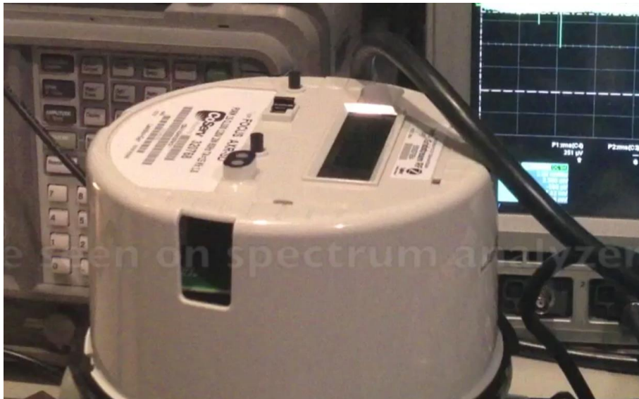
Figure 5-2 A screen capture from a video recording of evidence of GFCI tripping due to RF interference of a Smart Meter. Here, it can be seen that the wires being used to power the GFCI off of the Smart Meter are put in a circular fashion. It was found that this increased tripping events, and is possibly acting as an antenna.
