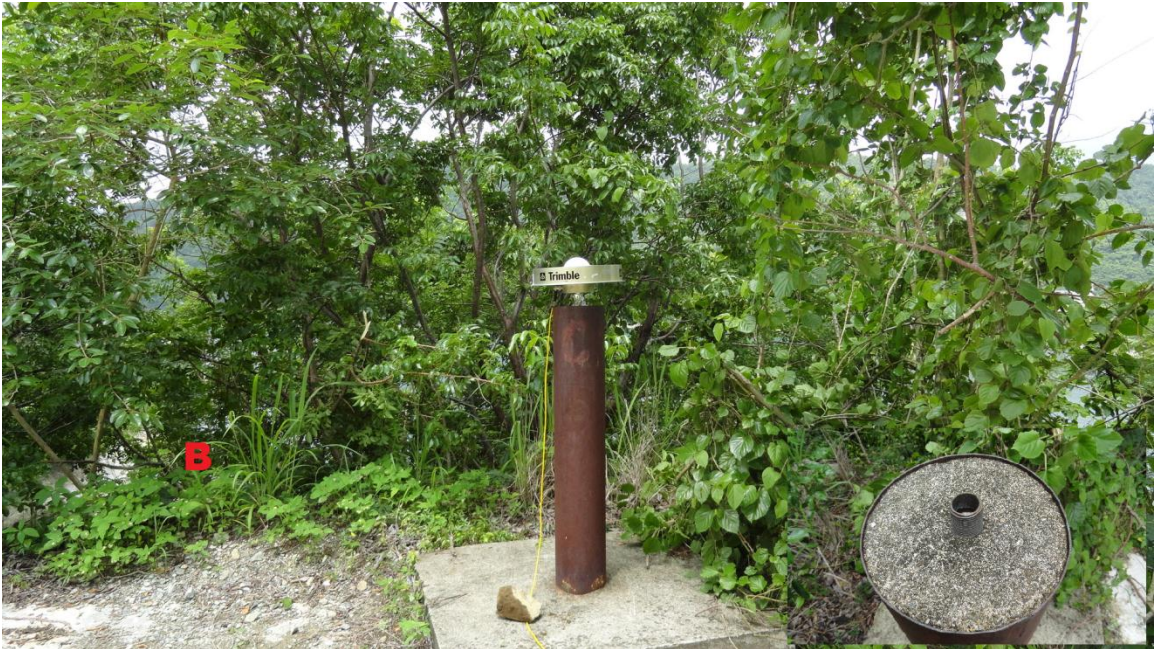
Figure A5. Photographs of site CCM5-PONCE acquired during June 2011. (A) Photoview of the site with solar power backup connected to the receiver facing northwest. (B) Photoview facing west while the inset photo shows the hole without an antenna. Note: This pipe will allow you to insert a 1" diameter brass antenna mount.
