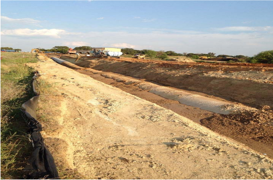
Figure 3- 6 CLSM around the Pipeline in the Prove-out Section
