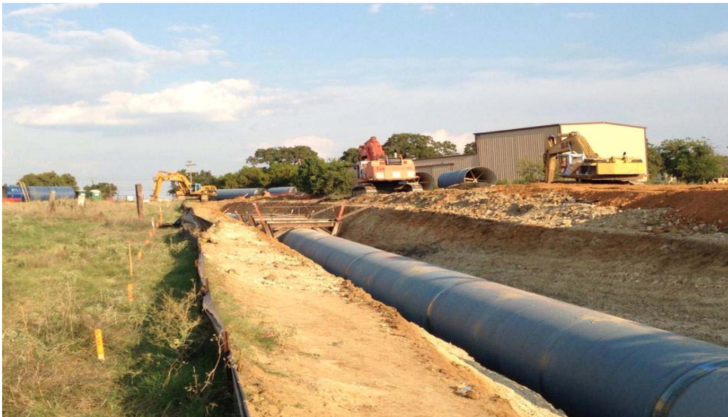
Figure 3- 5 Installation of the Pipeline in the Prove-out Section
