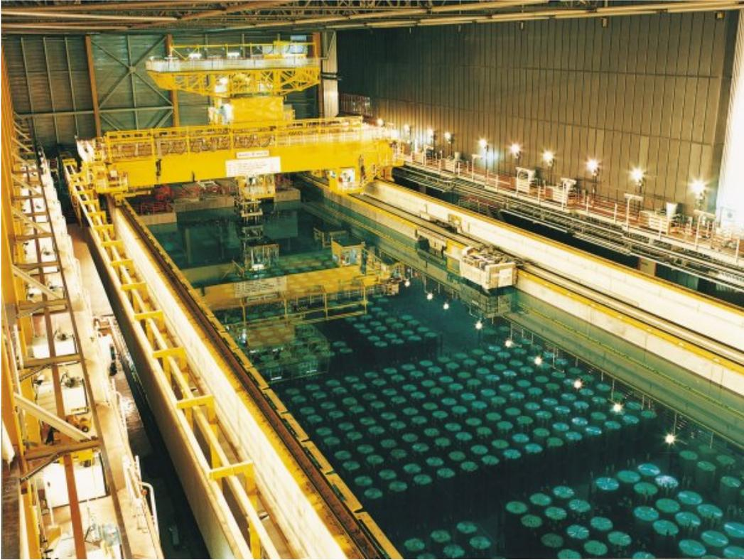
Figure 4: Storage pond for used fuel at the Thermal Oxide Reprocessing Plant at the UK's Sellafield site. (Sellafield Ltd)<sup>18</sup>
