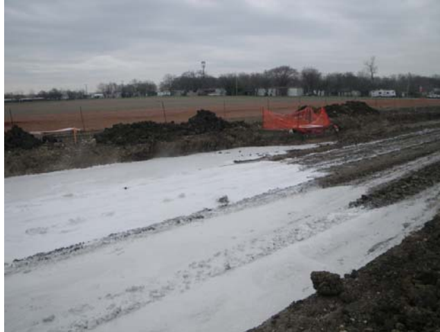
Figure 6.2 Lot 13 Lime Slurry Placement
