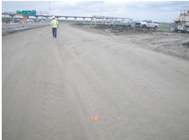
Figure 6.5 Finished Lot Compacted and Curing
