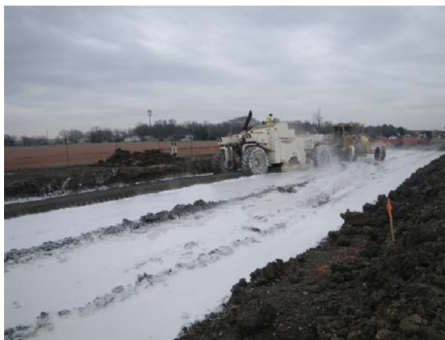
Figure 6.3 Lot 13 Mixing with Rotary Mixer
