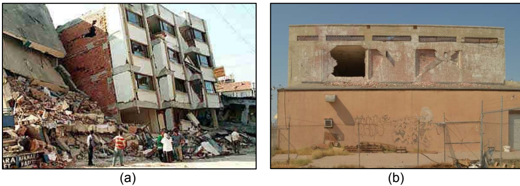
Figure 1.1 Examples of damaged buildings with RC frames and masonry infill panels. (a) Izmit, Turkey and (b) California, US.
