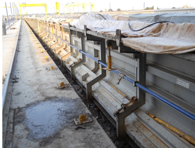
Figure 2.27: Girder line view with wet mat.
