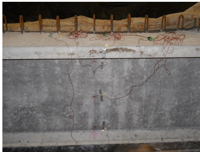
Figure 3.6: Strain gauges on the girder.
