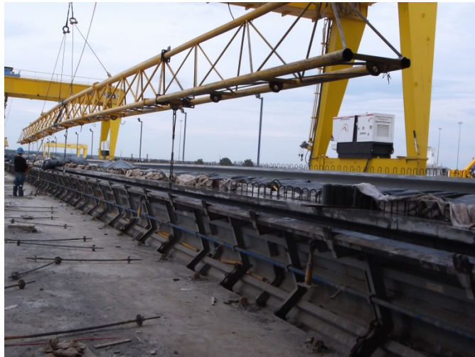
Figure 2.28: Crane opening girder mold.
