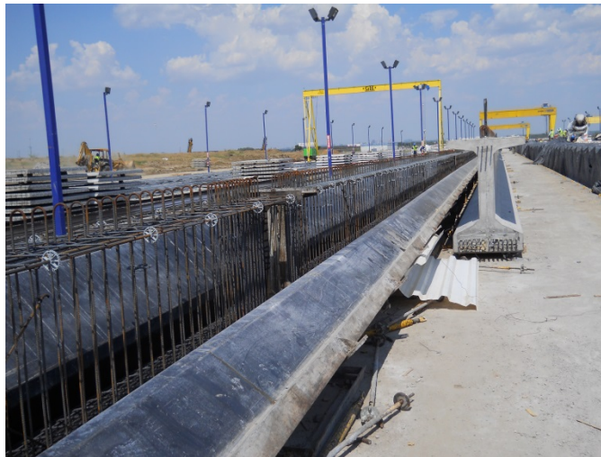
Figure 2.13: Reinforced steel after being placed in the casting bed.
