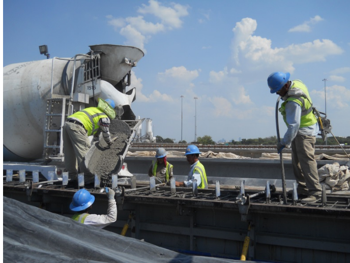
Figure 2.22: Concrete pour over the girder and concrete vibration.
