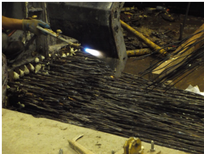
Figure 2.34: View of strands after being cut.
