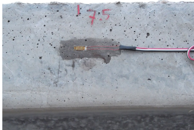
Figure 3.2: Strain gauge attached to the girder.
