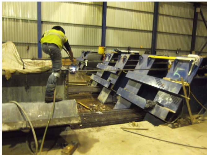
Figure 2.30: Worker flame cutting the top strands of girder.
