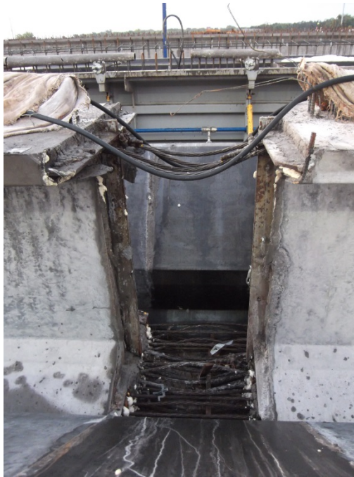
Figure 2.35: View between girders after cutting the strands.
