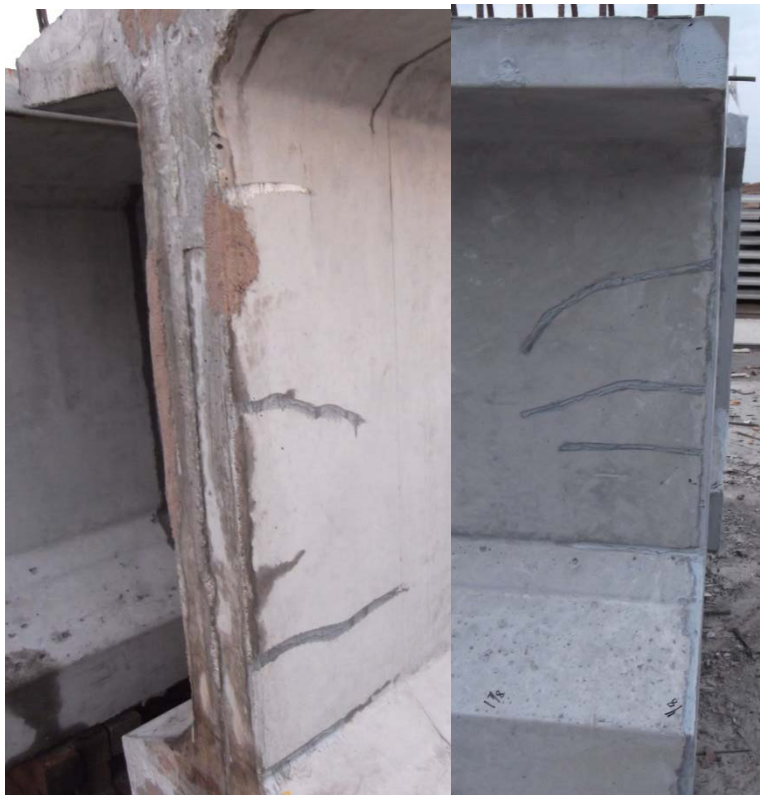
Figure 3.8: Microcraks at girder end.
