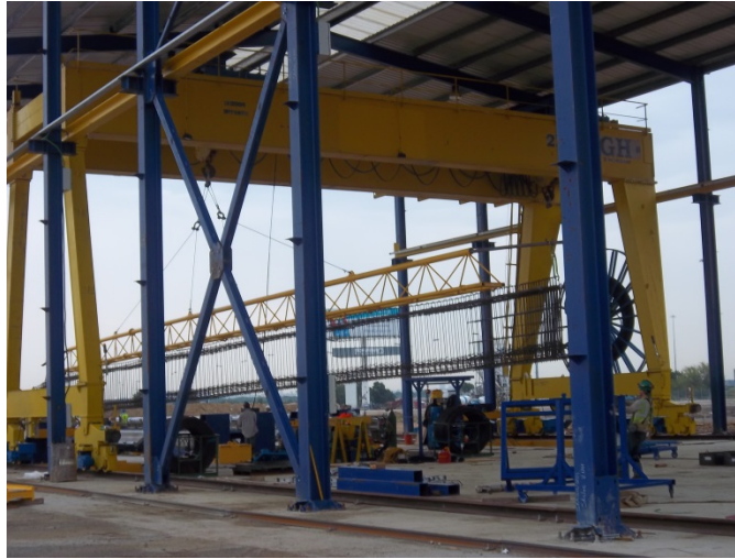
Figure 2.14: Girder reinforcement being moved to the casting bed.
