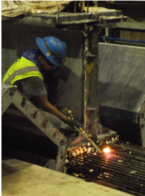
Figure 2.33: Worker flaming cut the bottom strands
