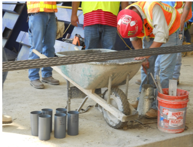
Figure 2.23: Worker realizing slump test.
