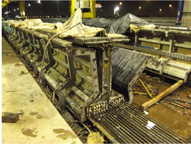
Figure 2.29: Girder mold partially opened.
