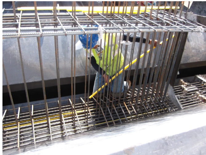
Figure 2.21: Worker placing the plastic sleeve to debond the strand.
