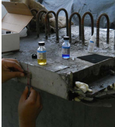
Figure 3.1: Coat protection over the strain gauge.
