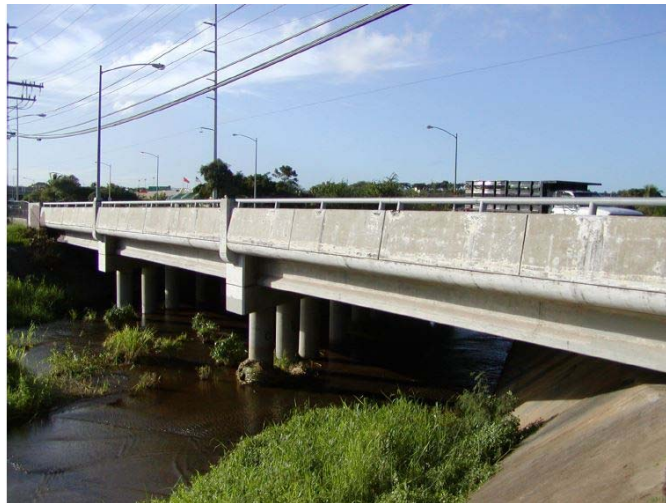
Figure 2-1 Elevation of Typical AASHTO-Type Girder Bridge
