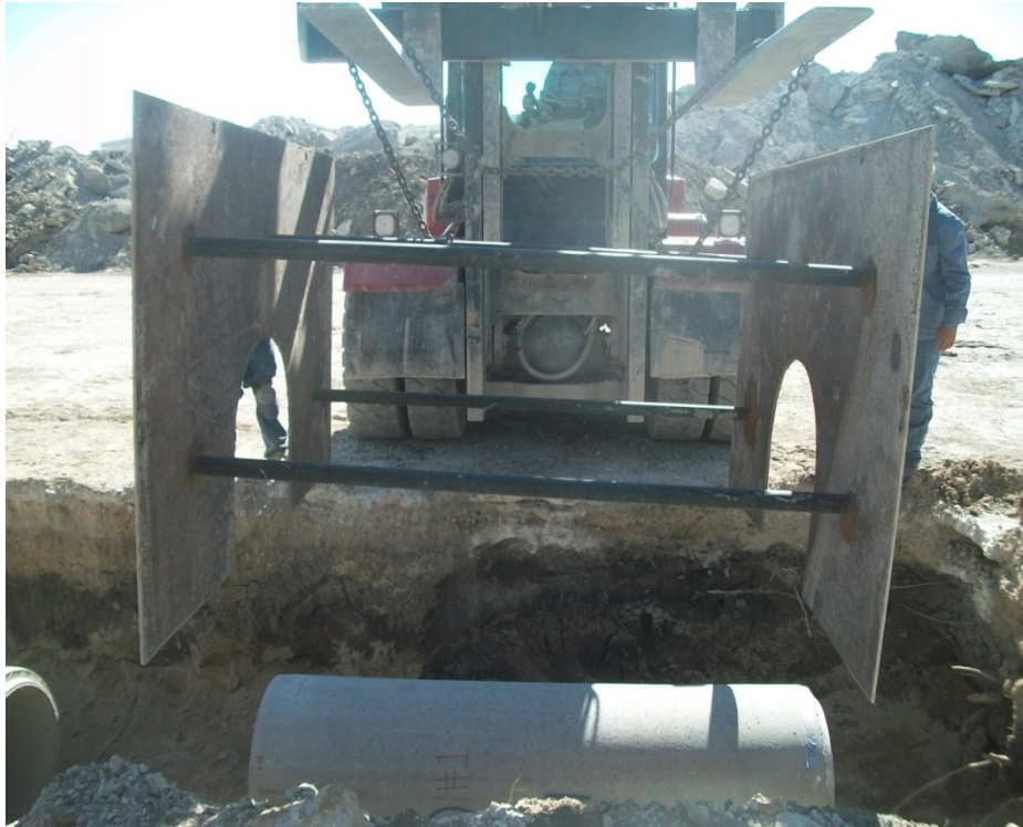
Figure A-13 Photograph for placing of steel capping-step 2
