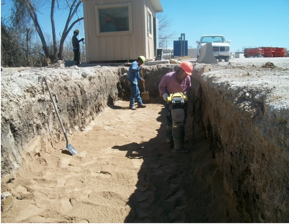
Figure A-7 Photograph of compaction of bedding
