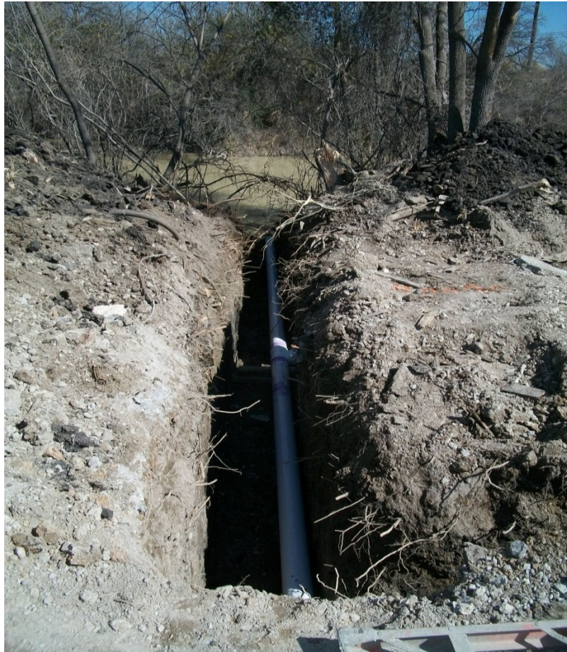
Figure A-3 Photograph of drainage installation
