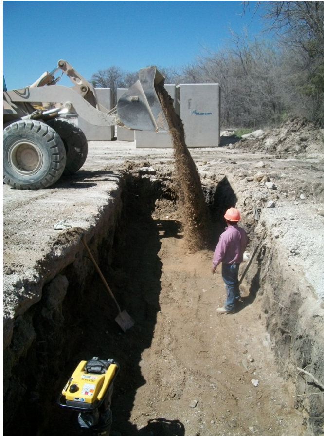
Figure A-6 Photograph of pouring of sand for bedding
