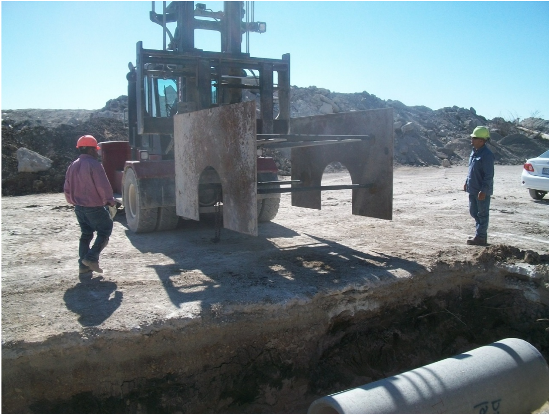
Figure A-12 Photograph for placing of steel capping-step 1
