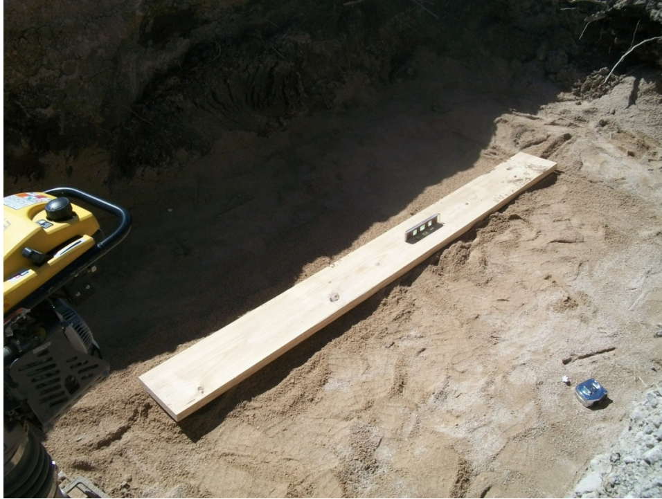
Figure A-8 Photograph of leveling check for bedding
