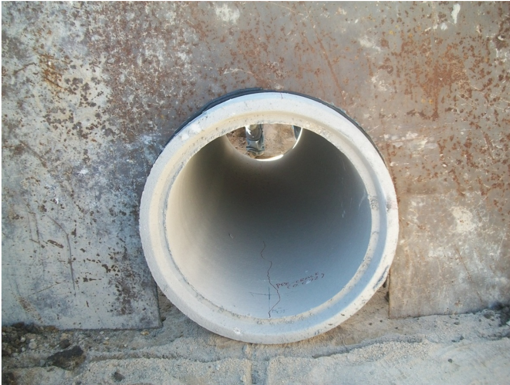
Figure A-15 Photograph of rubber strip and steel capping installed
