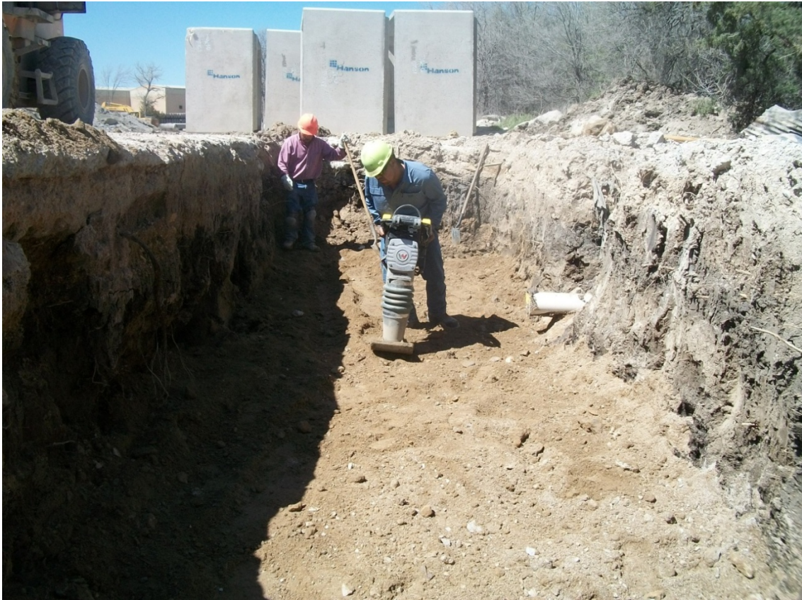
Figure A-5 Photograph of initial compaction of trench
