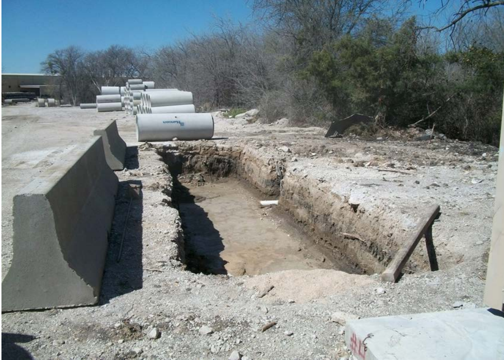
Figure A-1 Photograph of trench excavated
