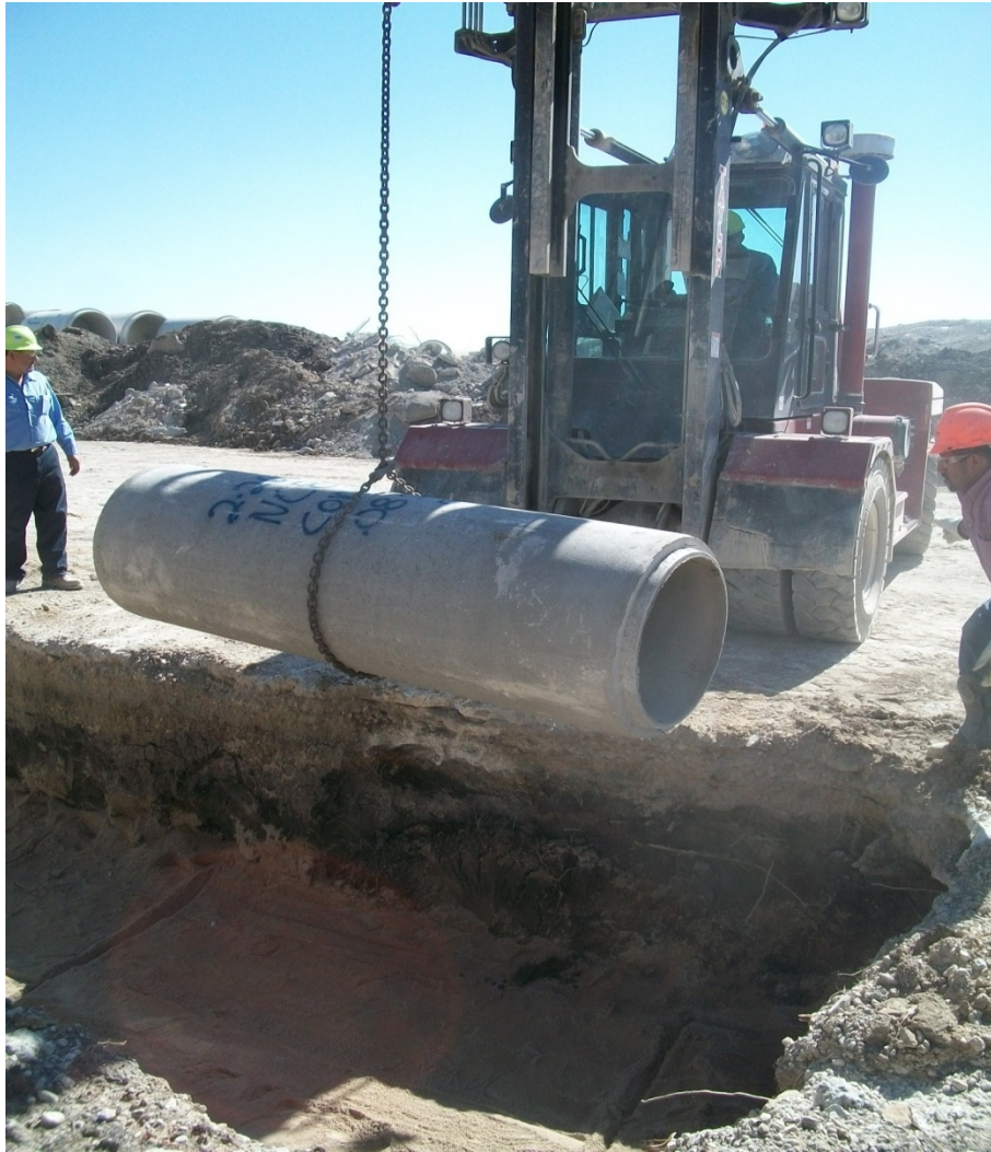
Figure A-10 Photograph of pipe being placed
