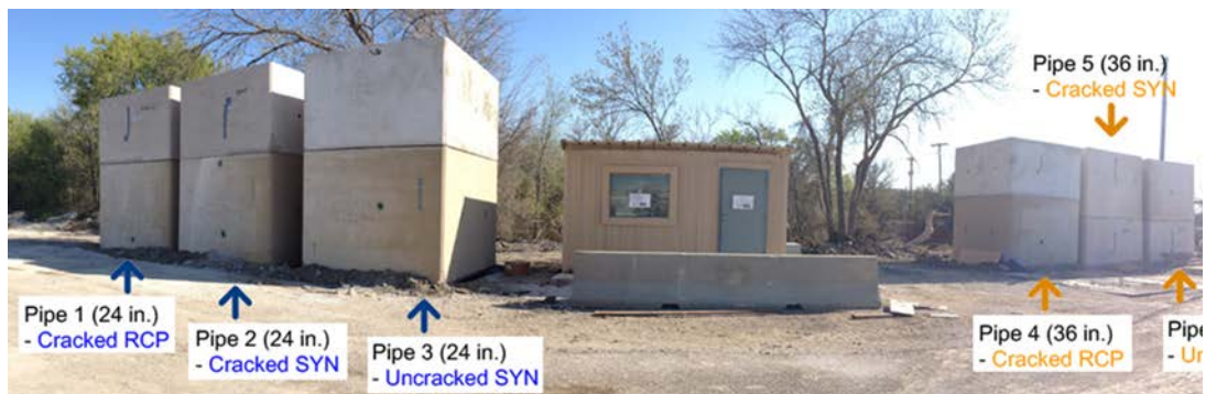
Figure 2-21 Final set-up for long-term monitoring
