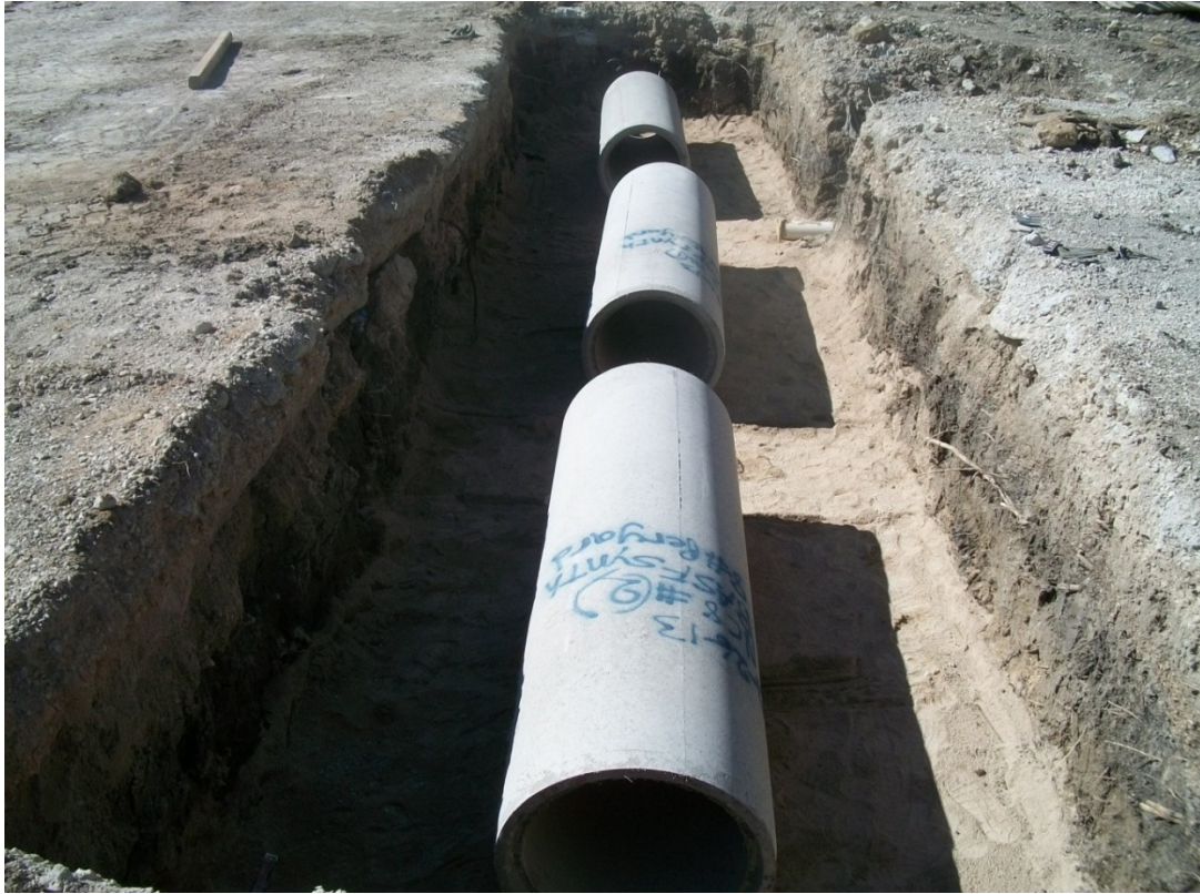
Figure A-11 Photograph of all three pipes placed in trench
