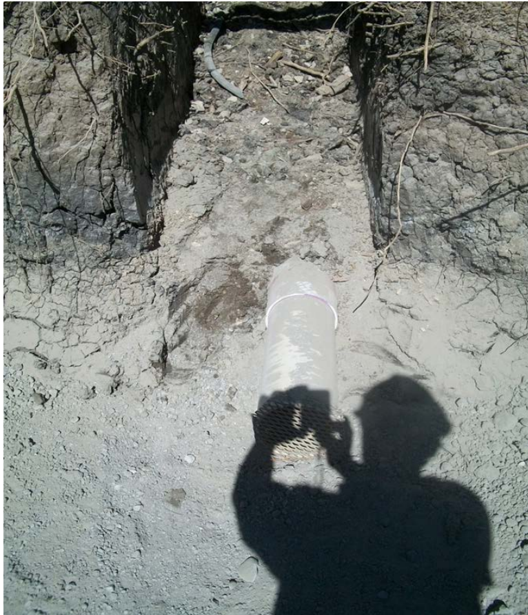
Figure A-2 Photograph of Trench excavated for drainage system
