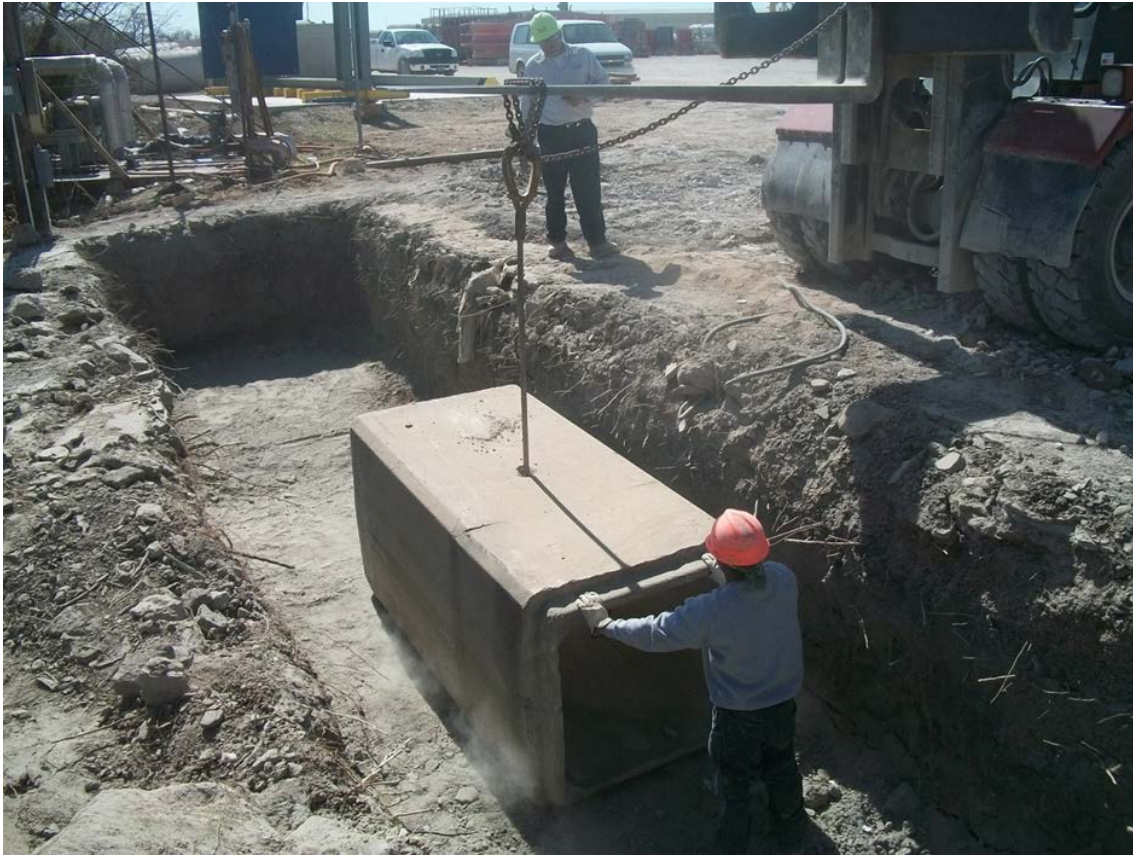
Figure A-4 Photograph of rough compaction of initial trench
