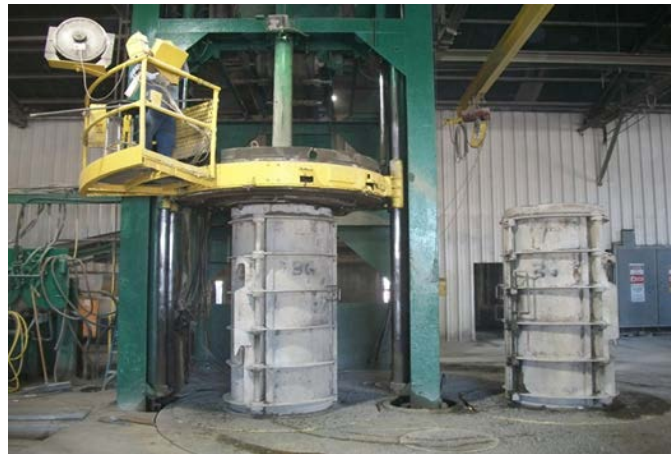
Figure 1-7 Photograph of Packerhead Equipment at Hanson Facility
