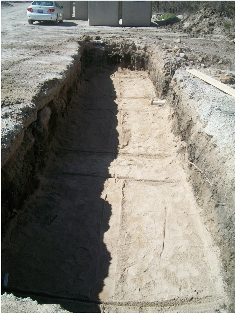
Figure A-9 Photograph of bedding marked for pipe placement
