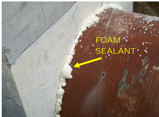
Figure 2 - 16 Connection of the pipe and the vault
