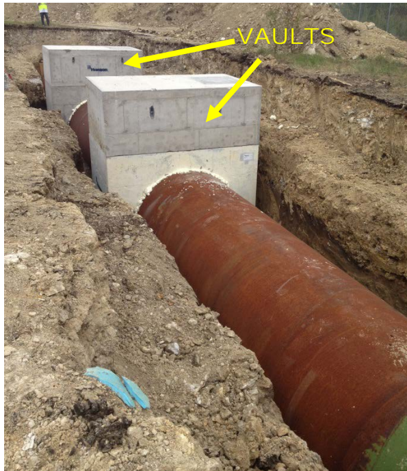
Figure 2 - 15 Overview of the trench
