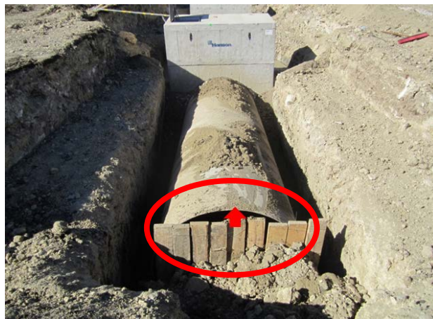
Figure 2 - 29 Pipe 1 after flotation
