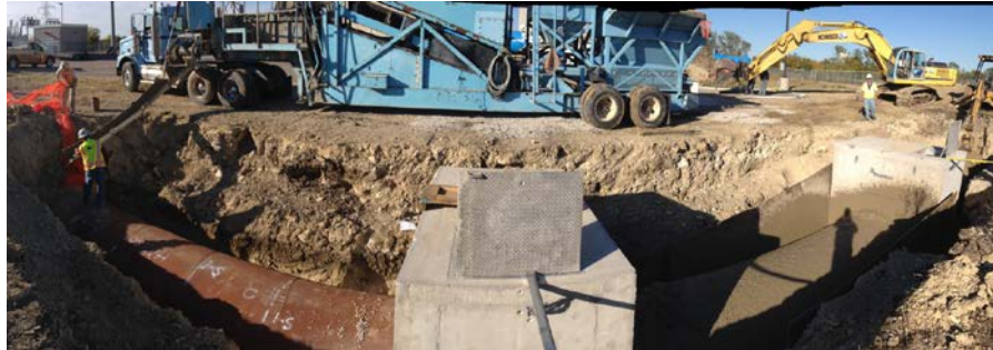
Figure 2 - 28 CLSM placing overview
