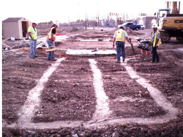
Figure 2 - 35 Soil layer surface after compaction
