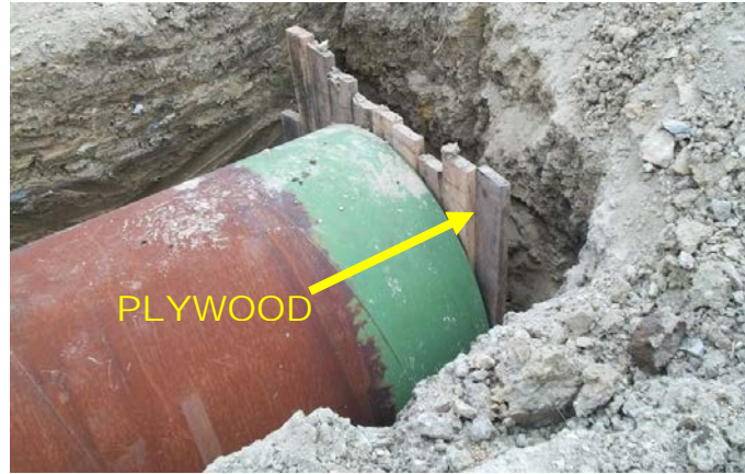
Figure 2 - 17 Pipe end closed with plywood
