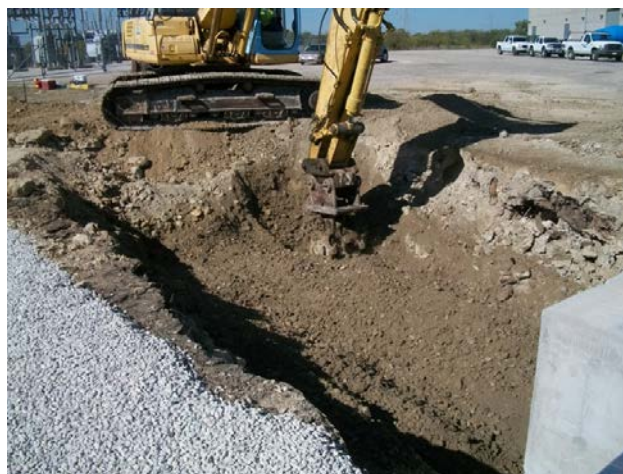
Figure 2 - 33 Compaction of the first backfilling layer
