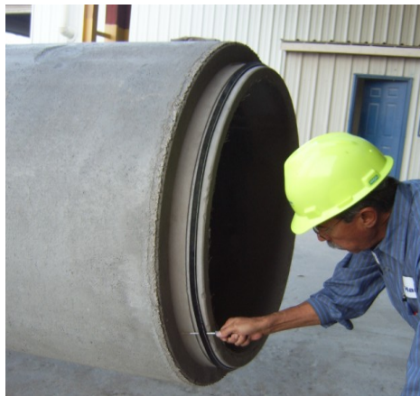
Figure 2-12 Equalizing the gasket for pipe installation
