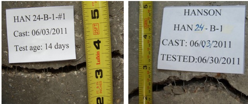
Figure B- 52 Typical crack opening for 24 in. (600 mm) SFRCP at 5% deformation
