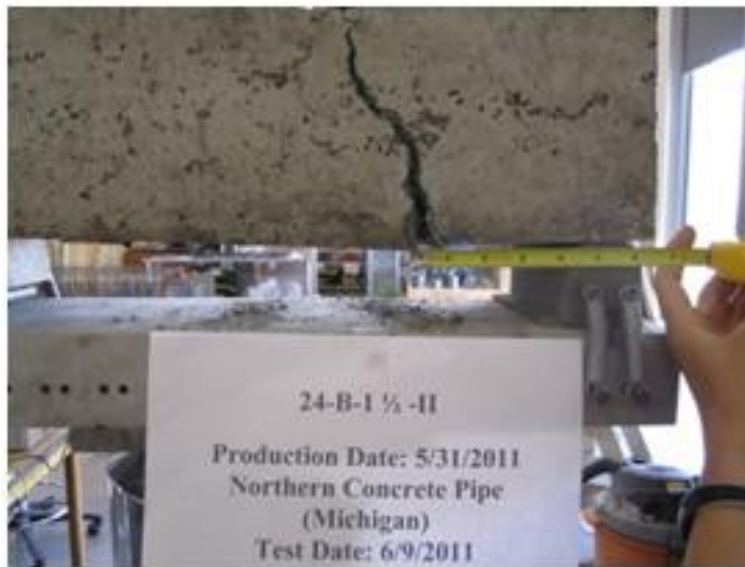
Figure D- 40 Crack pattern for NCP24-8-B-0.5-T1-BM
