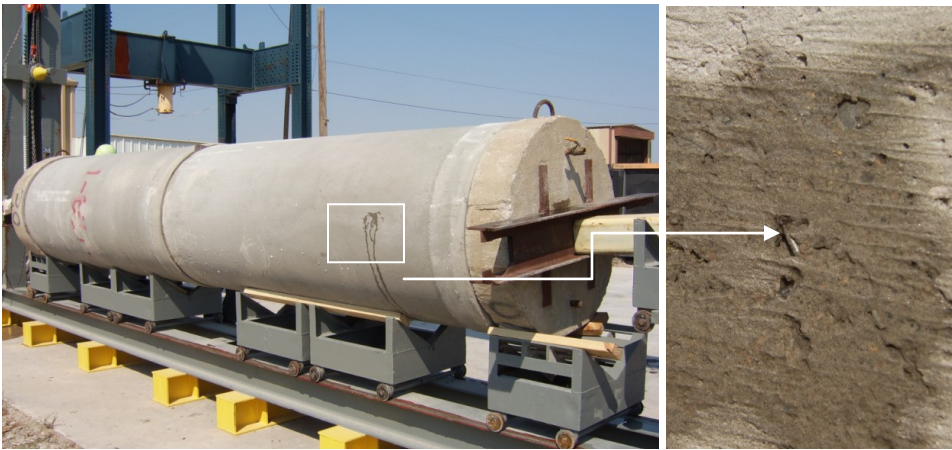
Figure B- 55 Specimen 1 for HAN-30-C-0.33 SFRCP minor seepage from a pinhole
