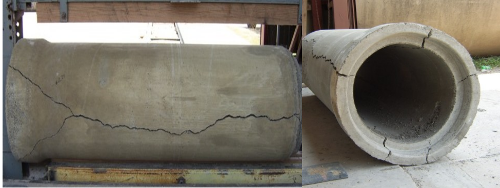
Figure 2-20 Typical crack pattern for SFRCP with bell
