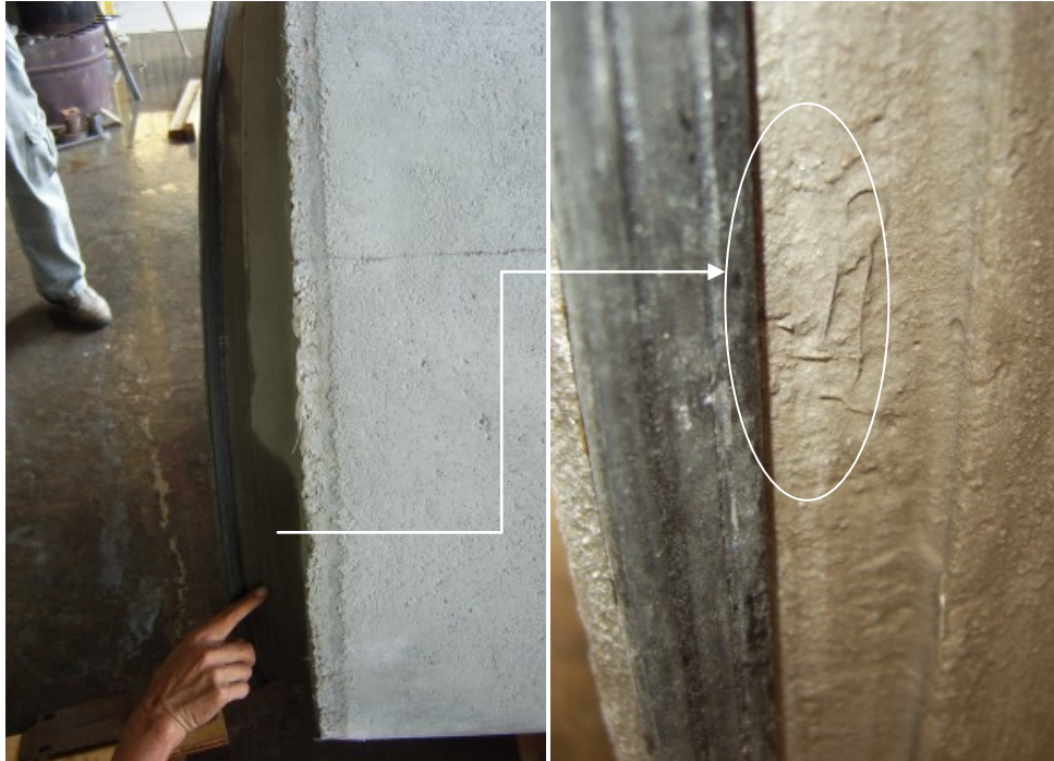
Figure B- 58 Specimen 4 for HAN-36-C-0.83 joint leaking location
