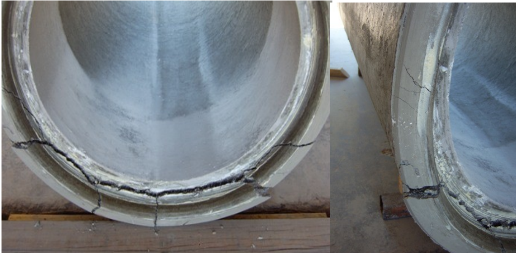
Figure B- 60 Specimen #1 joint shear joint failure pattern
