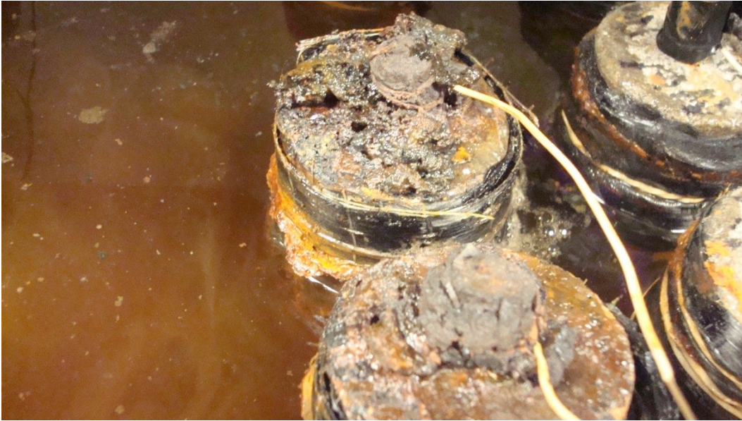
Figure 4-6 Localized Corrosion at the Concrete-Rebar Interface
