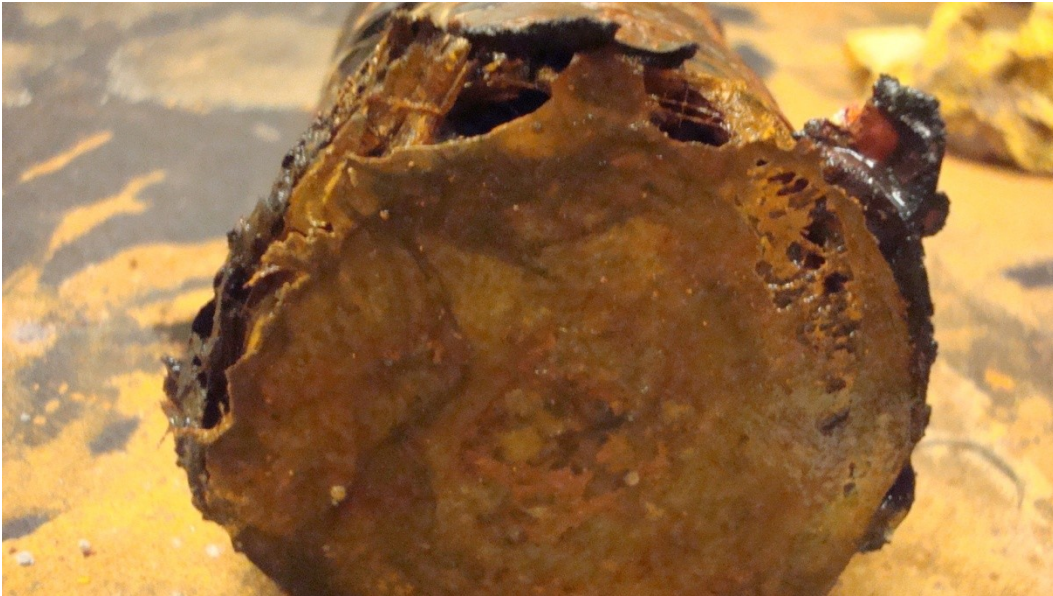
Figure 4-4 Debonding of the FRP from the substrate
