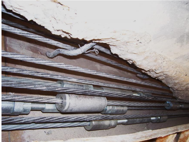
Figure 1-3 Spliced Strands
