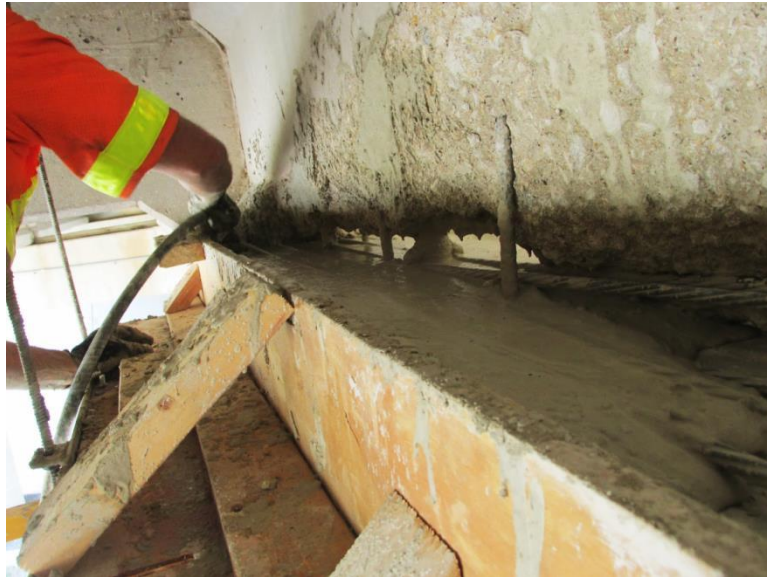
Figure 1-6 Consolidation
