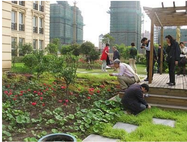
Figure 2.5 Intensive Green Roof (Winter Street Architects, 2010)
