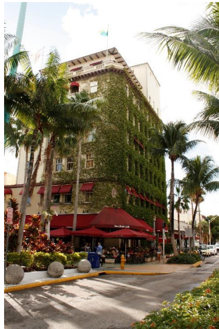
Figure 2.1 Example of Traditional Green Façade, Miami, Florida (Ozdil, 2013)
