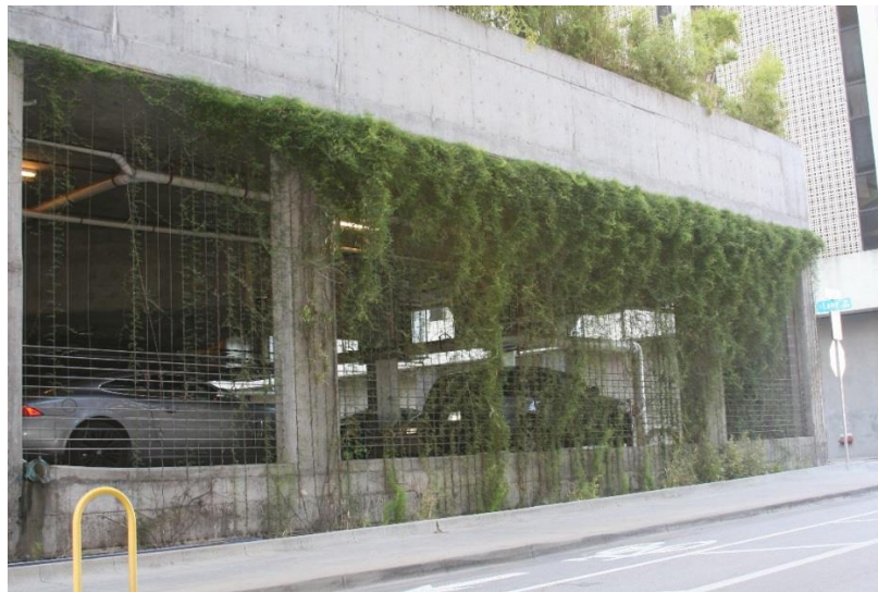
Figure 3.12 Green Wall at 1514 Commerce Street, Dallas, TX.
