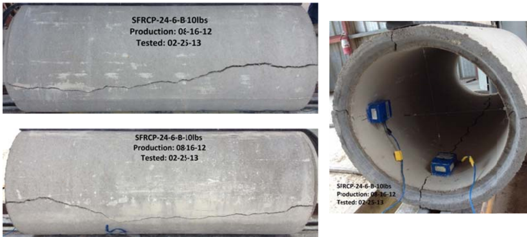
Figure B-40 Crack propagation for SFCP-24-6-B-10lbs steel
