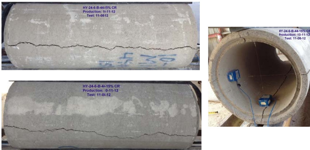
Figure B-101 Crack propagation for HYCP-24-6-B-44lbs steel-15%rubber
