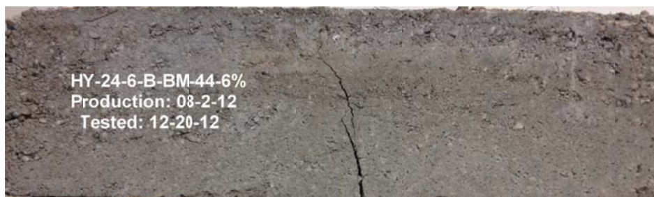
Figure C-8 Photograph of Crack for HY-24-6-BM-44lbs-6%
