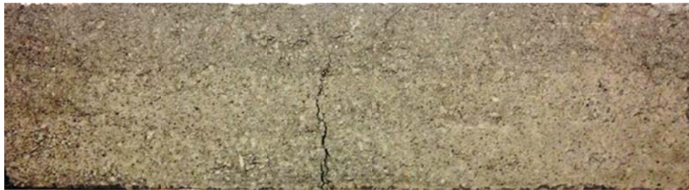
Figure 4-4 The photograph of most frequent failure type for Flexural Beam Specimens
