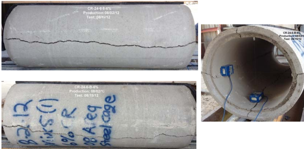
Figure B-16 Crack propagation for CRCP-24-6-B-6%rubber
