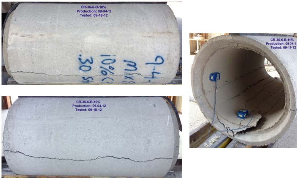
Figure B-66 Crack propagation for CRCP-36-6-B-10%rubber
