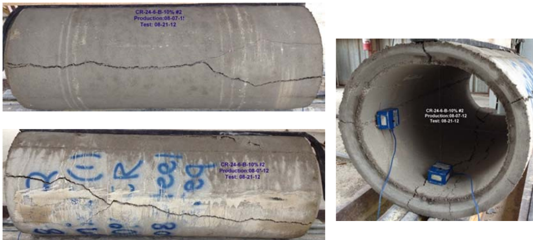
Figure B-32 Crack propagation for CRCP-24-6-10%rubber
