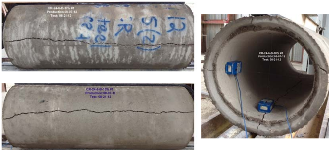
Figure B-30 Crack propagation for CRCP-24-6-10%rubber
