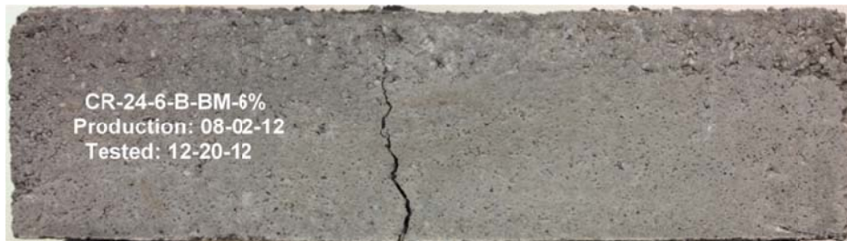
Figure C-10 Photograph of Crack for CR-24-6-BM-6%
