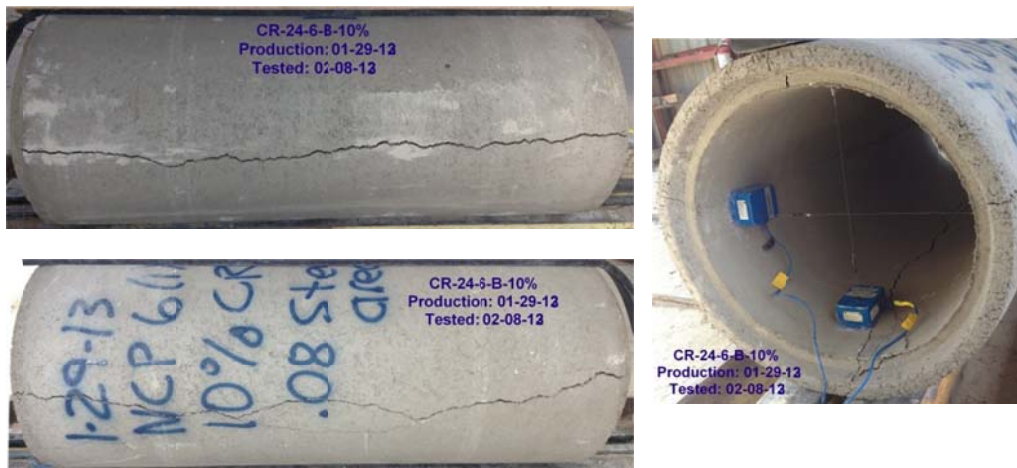
Figure B-130 Crack propagation for CRCP-24-6-10%rubber
