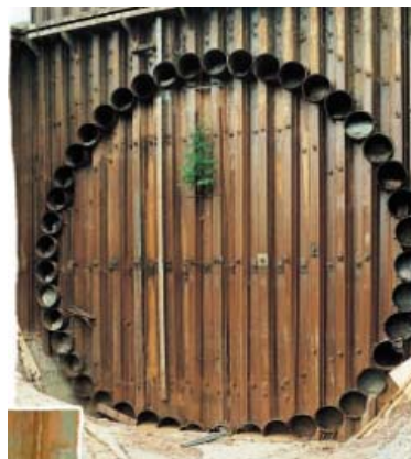
Figure 2-8 Pipe Roofing Project in Germany (Tracto-Technik, 2004)
