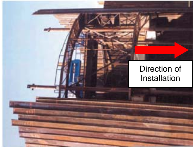
Figure 3-1 Metal Sheet Piles Tilted Horizontally (ArcelorMittal, 2008)
