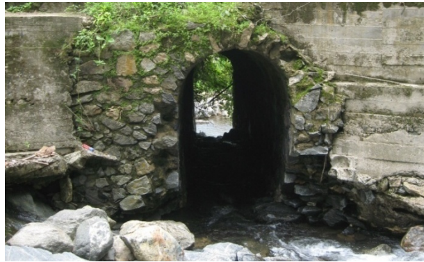
Figure 2-4 Stone Masonry Culvert in Mexico
