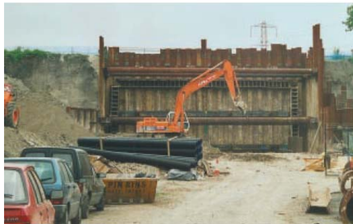
Figure 2-9 Jobsite of the Special "I" Beam Ramming Project (Tracto-Technik, 2004)
