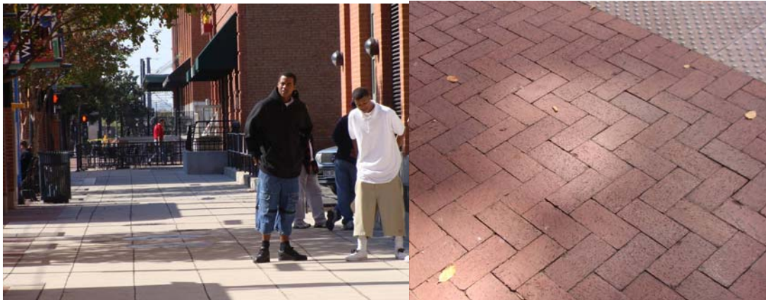
Figure 4.24 Surface Material along the West End Segment
