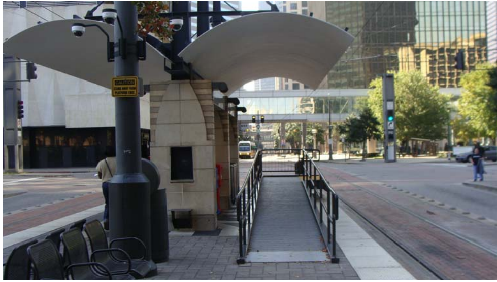
Figure 4.52 Boarding Ramp at Pearl Station
