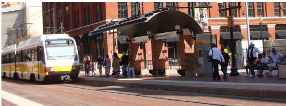
Figure 4.50 Overhead Structure at West End Station
