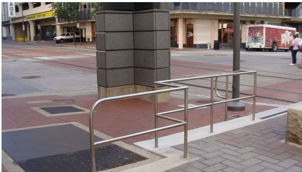
Figure 4.53 Curb Ramps at the St. Paul Segment
