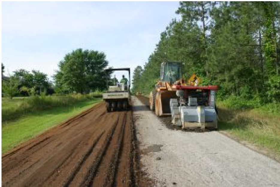
Figure 2.9 Full Depth Reclamation Process (Source: http://www.asphaltzipper.com/img/full_depth_reclamation3.jpg )
