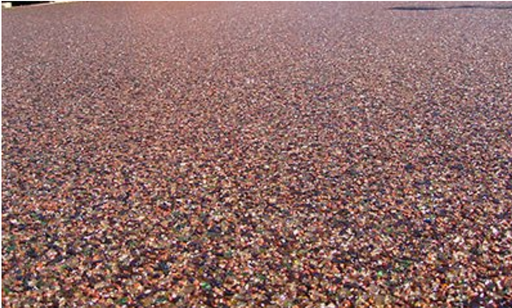
Figure 2.2 Recycled Glass Driveway (Source: http://swamplot.com/wp-content/uploads/2009/01/filterpave-cordell.jpg )
