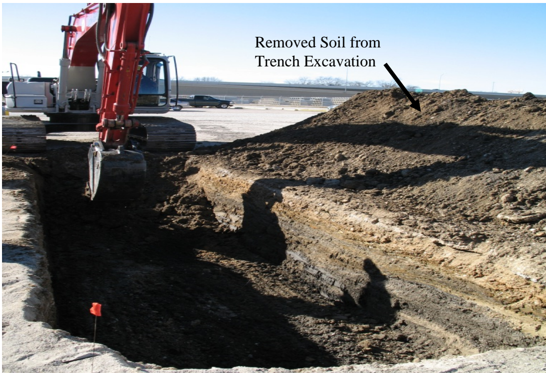
Figure 2.8 Accomplished trench excavation.
