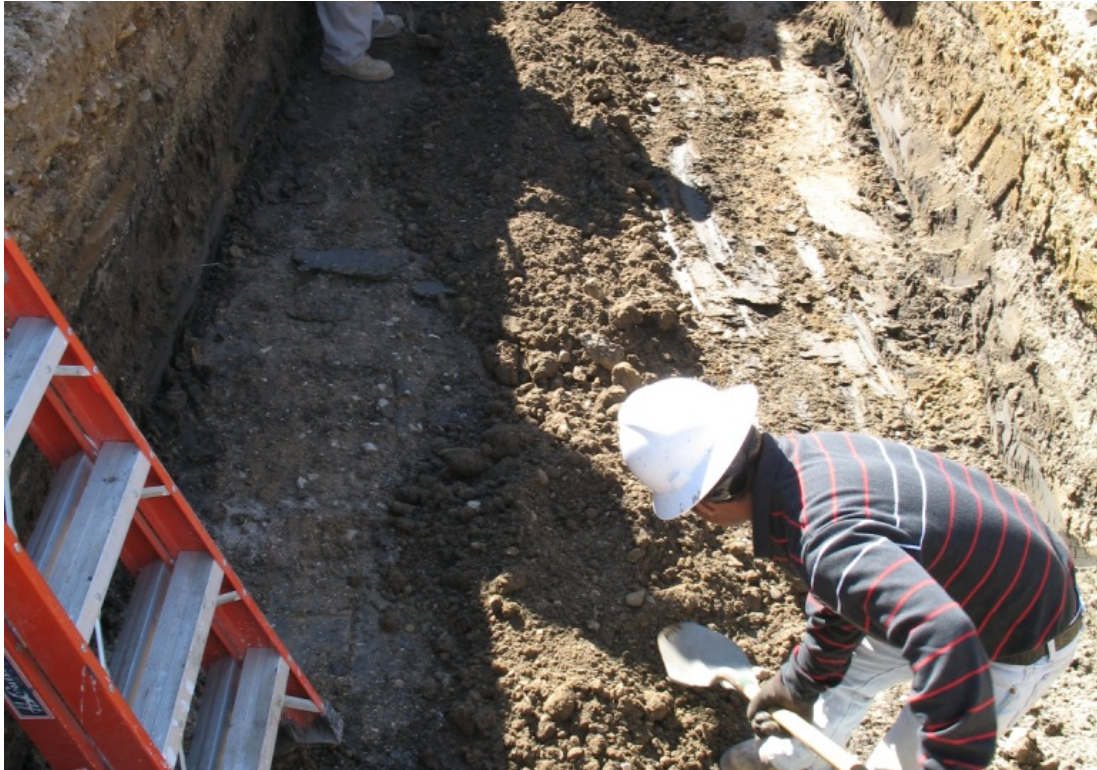
Figure 2.9 Bedding zone preparation.
