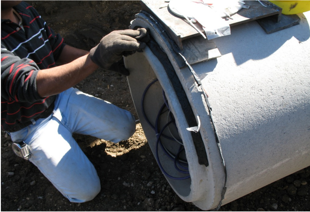
Figure 2.11 Sealing work at the pipe joint.
