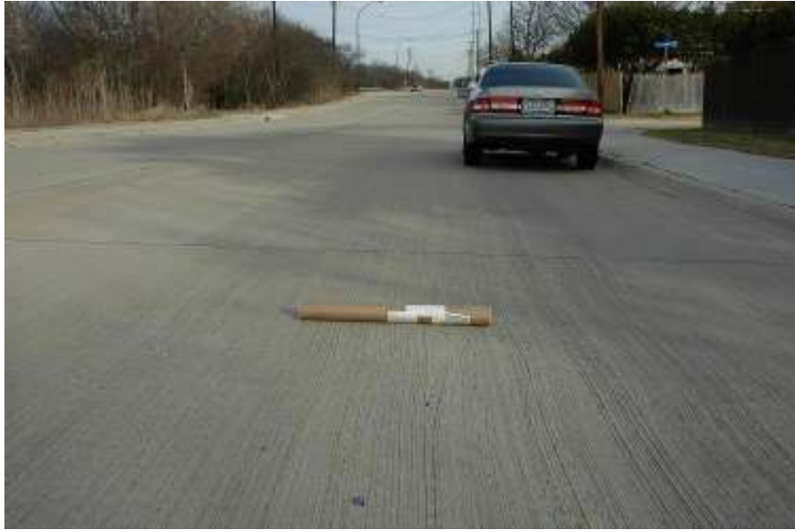
Figure A1 Current Condition of Harwood Road (Cement Treated Section).
