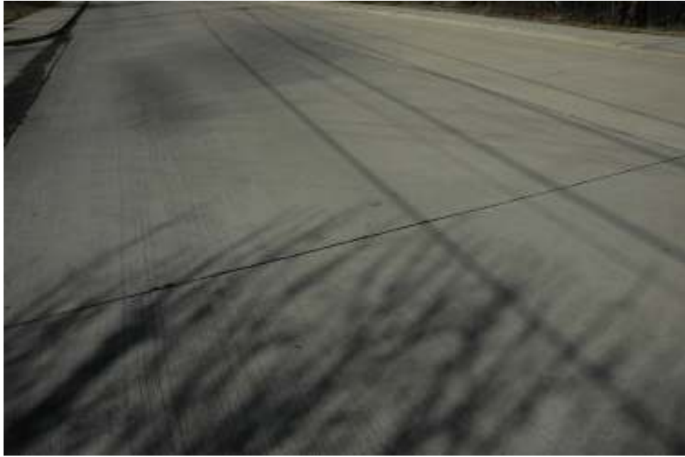
Figure A3 Current Condition of Harwood Road (GGBFS Treated Section).
