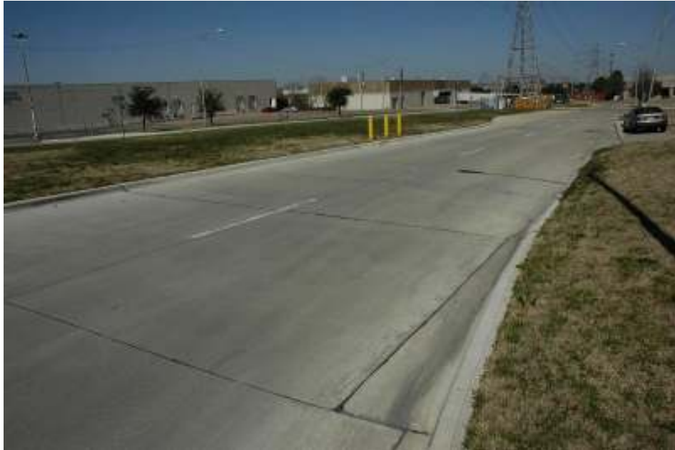
Figure B1 Current Condition of International Parkway.
