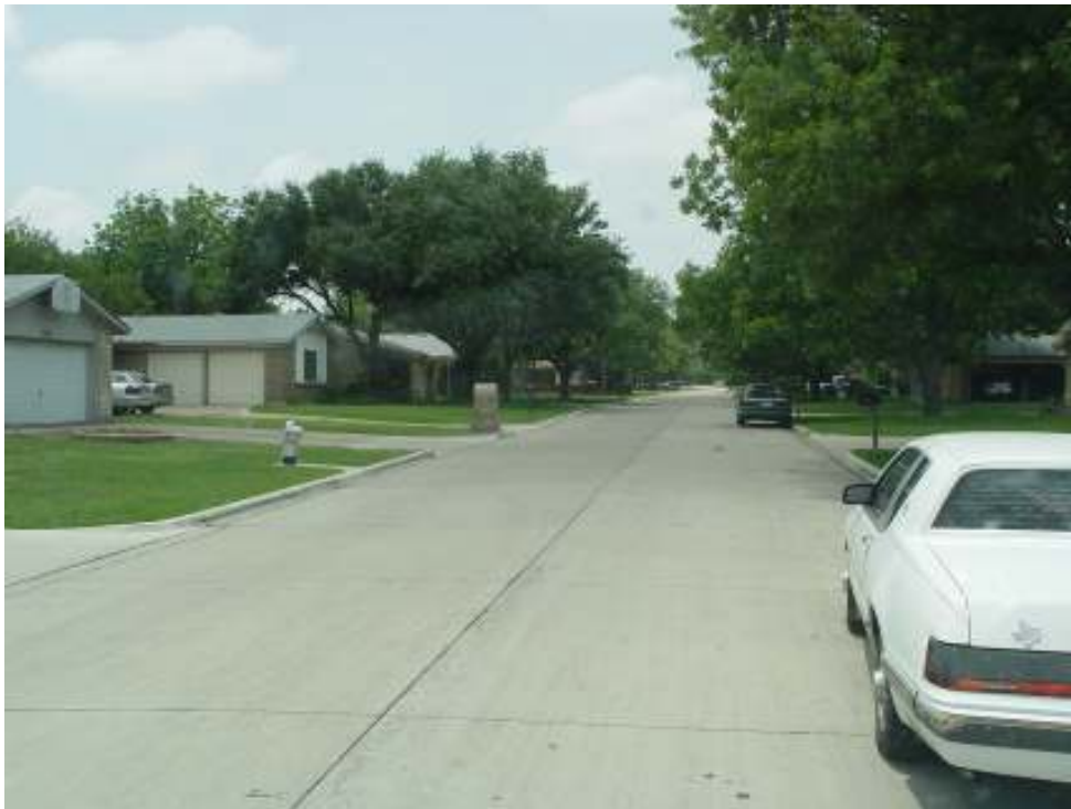
Figure 6.37 Current Condition of Southmoor Drive (Continue).
