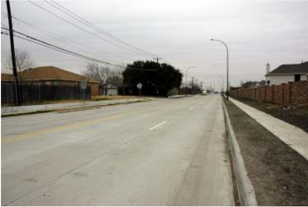
Figure B3 Current Condition of Southeast Parkway.
