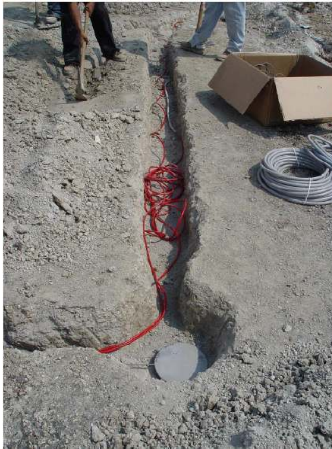
Figure 5.8 Placements of Pressure Cells (Pillappa, 2005).
