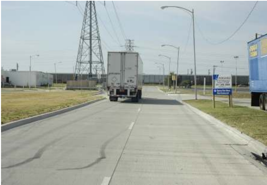
Figure 6.32 Heavy Traffic Load at International Parkway.
