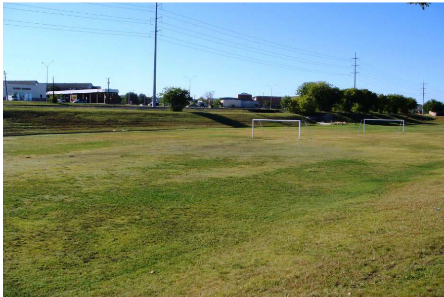
Figure 2.17: Detention basin doubling as a recreational playing field in Fort Worth, Texas (Voight, 2008)
