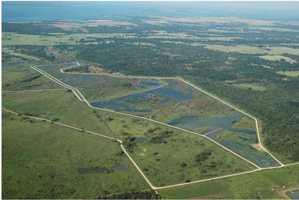
Figure 2.19: Aerial perspective of Tarrant Regional Water District’s George W. Shannon Wetlands Water Recycling Facility (field scale phase) along Richland-Chambers Reservoir near Corsicana, Texas (photograph courtesy of Alan Plummer Associates, Inc., 2005)
