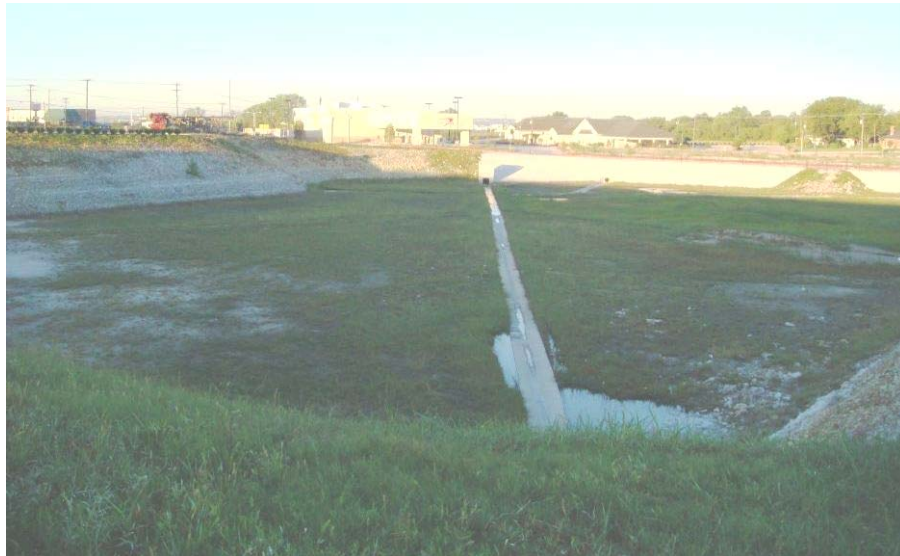
Figure 2.15: Detention basin system for a large box retail development in Fort Worth, Texas (Voight, 2008)
