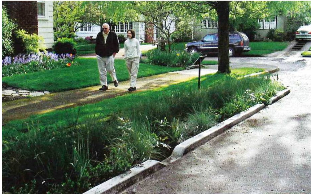
Figure 2.35: Curb extension located on Northeast Siskiyou Street in Portland, Oregon (Kays, 2006)
