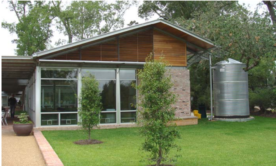
Figure 2.37: Rainwater collection storage tank at the Shangri La Botanical Gardens (Voight. 2008)
