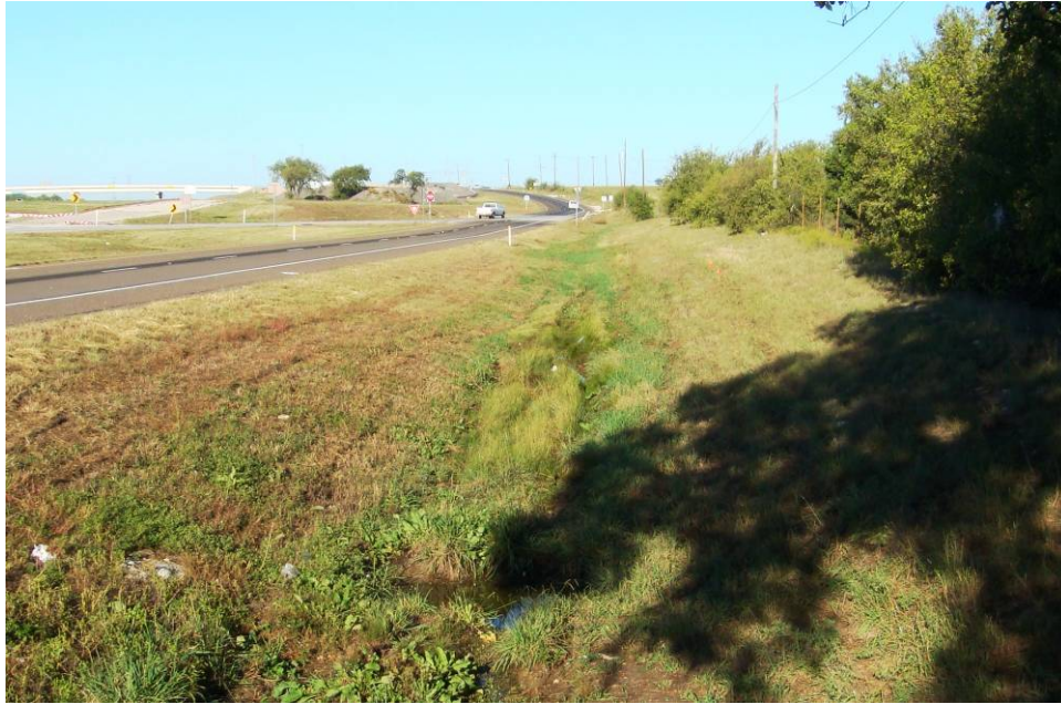
Figure 2.22: Vegetated swale with wetland type vegetation ( Eleocharis spp. ) (Voight, 2008)
