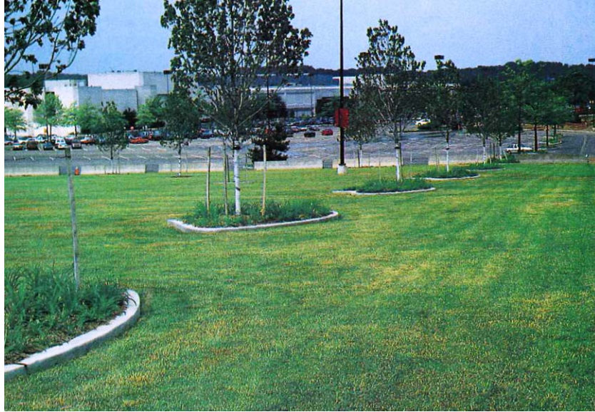
Figure 2.25: Reinforced stabilized turf in an overflow parking area (Thompson, 1996)
