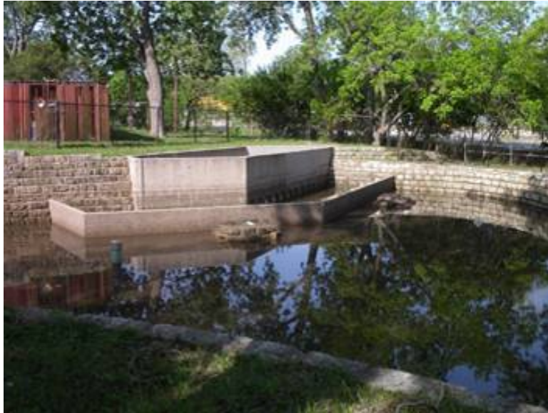
Figure 2.30: City of Austin, Texas' Gillis Park Sedimentation/Filtration Pond (City of Austin, 2008)
