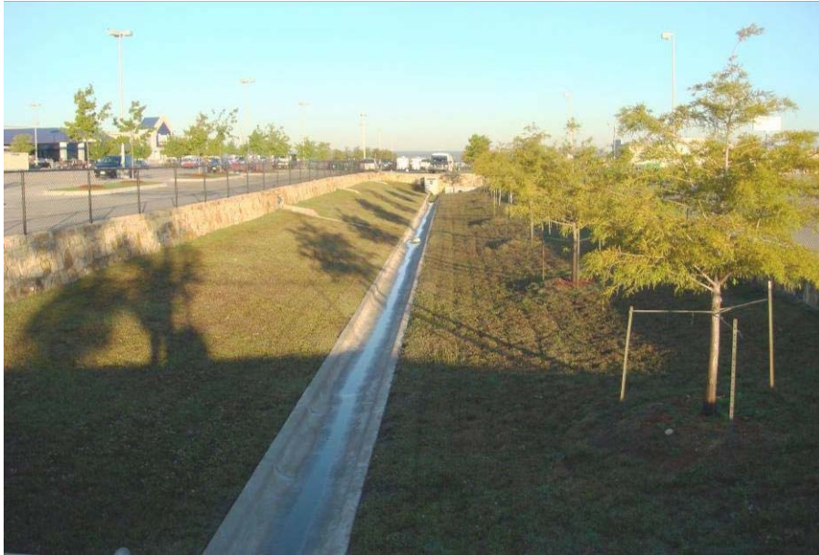
Figure 2.16: Detention system for a retail strip center in Fort Worth, Texas (Voight, 2008)
