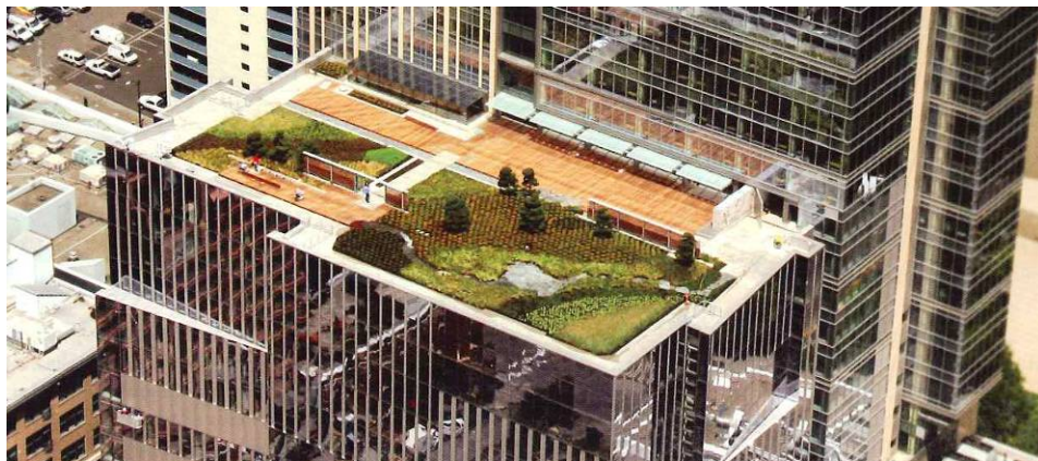
Figure 2.41: Roof garden atop Washington Mutual's (Chase Bank) headquarters in Seattle, Washington (McIntyre, 2007a)
