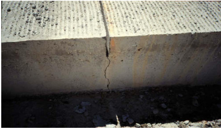
Figure 2.5: Aggregate Interlock
