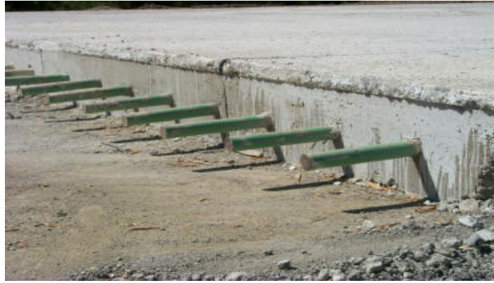
Figure 2.6: Dowel bar in place
