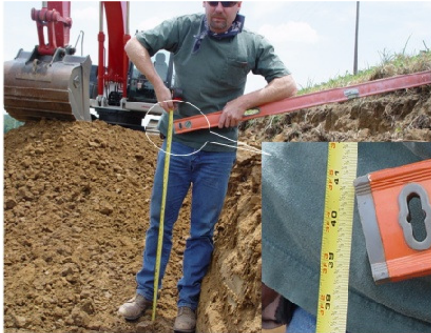
Figure 4.8 Depth of excavation near top of berm
