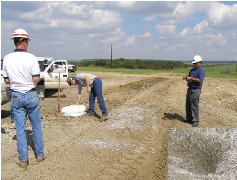
Figure 4.28 Spreading of fibers on soil in Zone 3 and Zone 4 (Inset: Observation pit)
