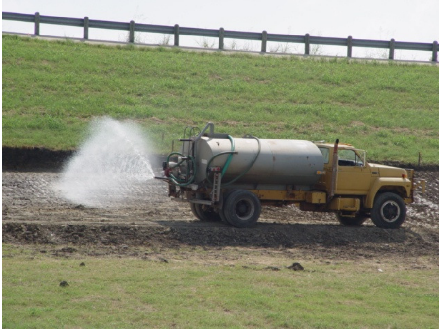
Figure 4.22 Watering of test sections
