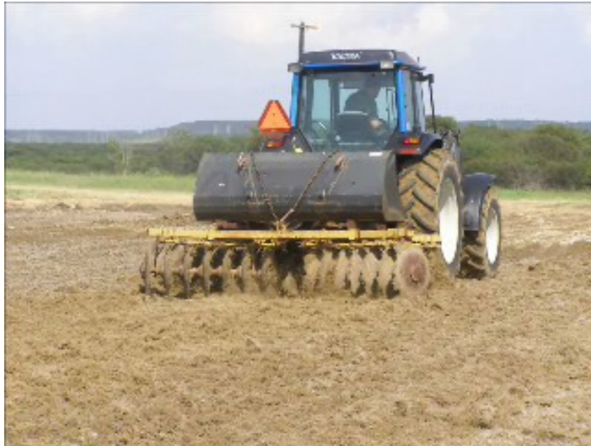
Figure 4.19 Mixing of fibers with lime soil mix
