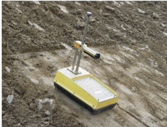
Figure 4.29 Nuclear gage for compaction quality control
