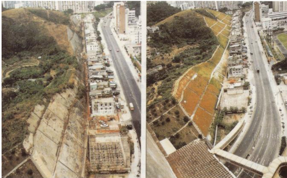
Figure 2.28 Slope before and after retrofitting (Ortigao and Sayao, 2004)
