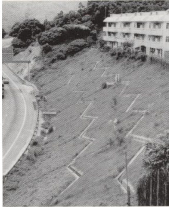
Figure 2.27 Surface drainage on a slope at Hong Kong (Source: Ortigao and Sayao, 2004)
