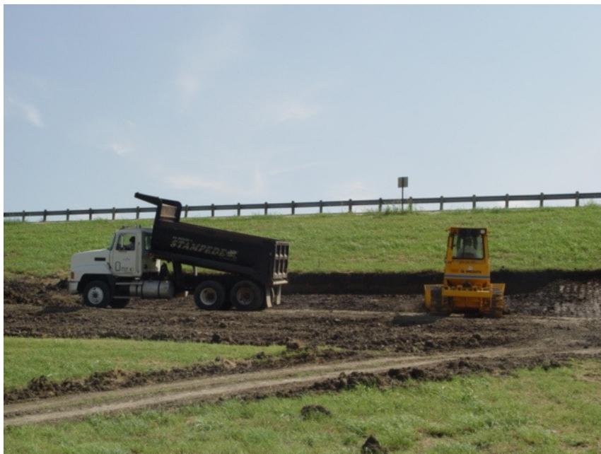
Figure 4.21 Unloading of treated soil on slope and leveling
