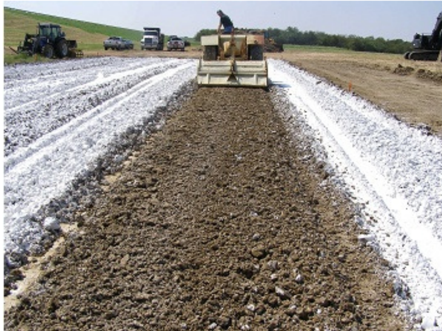
Figure 4.16 Mixing of lime with soil on level pad
