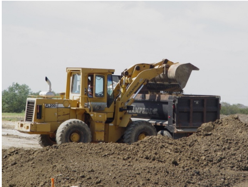
Figure 4.20 Loading of treated soil in to truck
