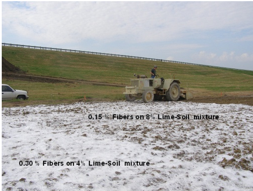
Figure 4.18 Polypropylene fibers spread on soil mixed with lime
