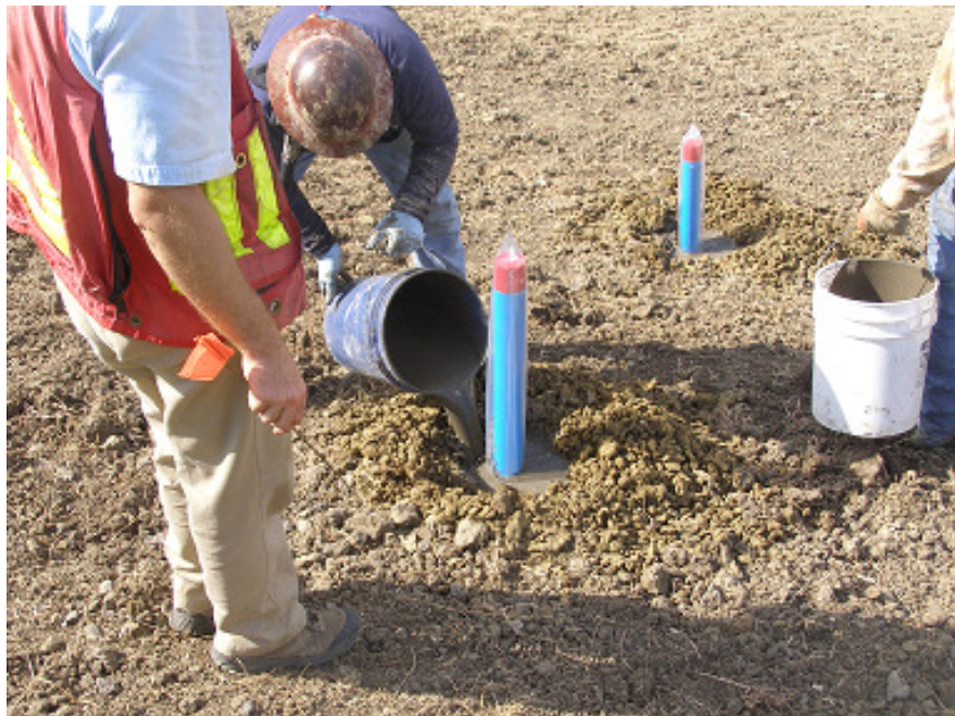
Figure 4.34 Grouting of inclinometer casing bore hole
