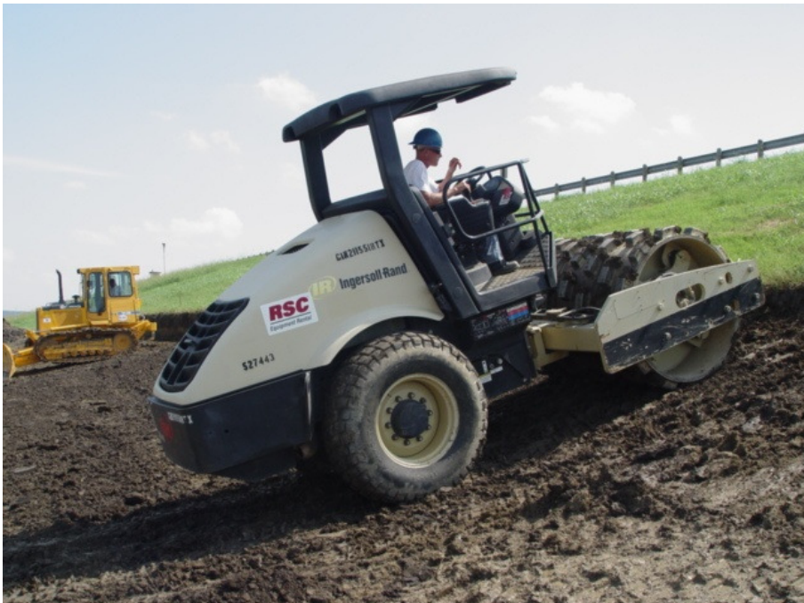
Figure 4.23 Compaction with sheep foot roller
