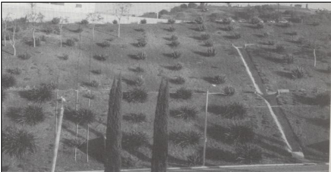
Figure 2.33 Landscaped slope with drainage and plantings (Source: Gray and Sotir, 1996)
