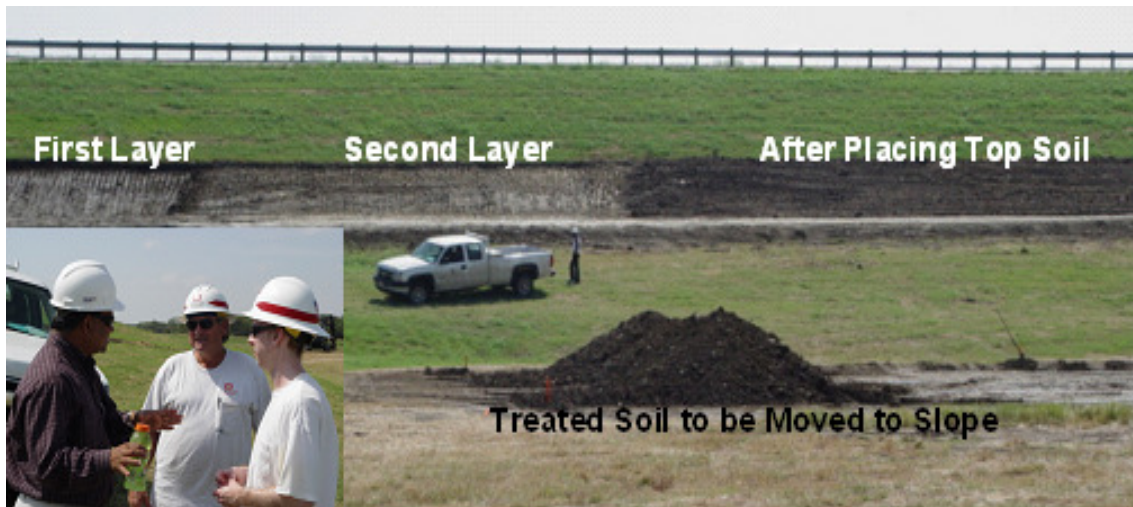
Figure 4.25 Placement of treated soil in the embankment (Inset: Planning of work)
