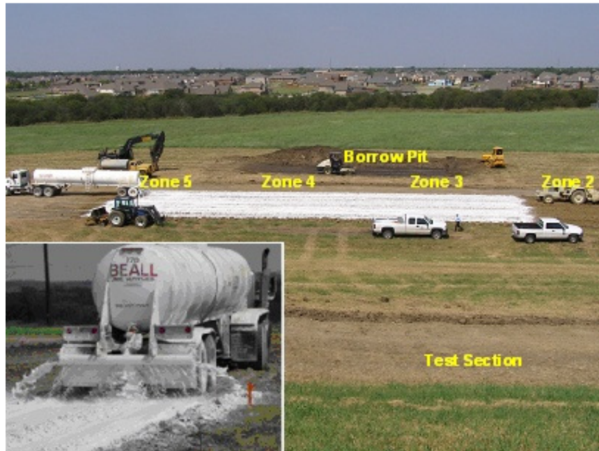
Figure 4.15 Spreading of lime slurry on the pulverized soil
