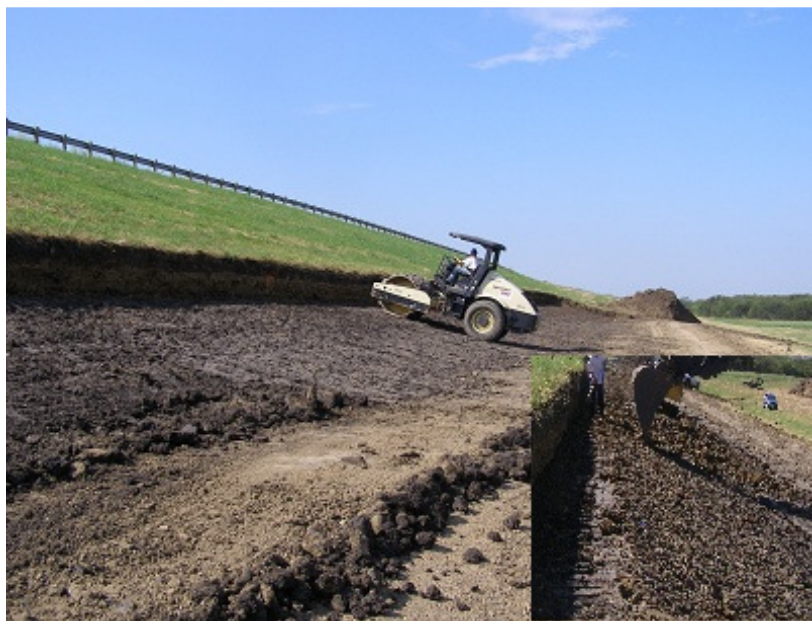
Figure 4.9 Preparation of bottom surface of excavation (Inset: preparation of berm)
