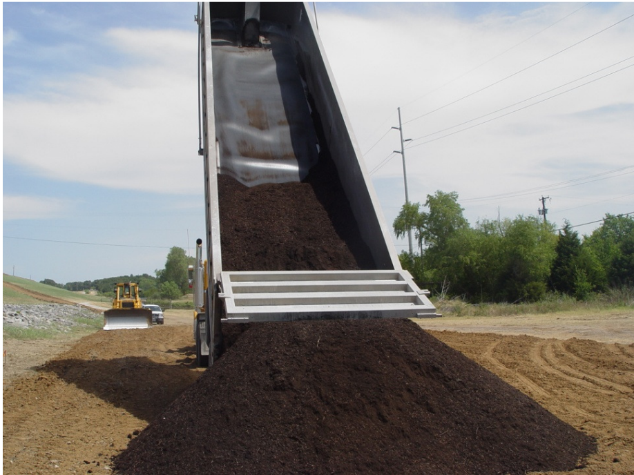
Figure 4.13 Unloading of compost in Zone 2 of level pad
