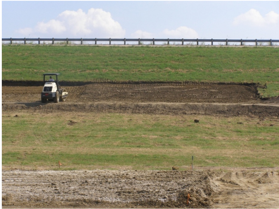
Figure 4.24 Compacted section with 8% lime
