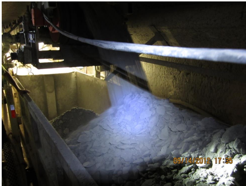
Figure 1.6. A muck car being filled during TBM operations.
