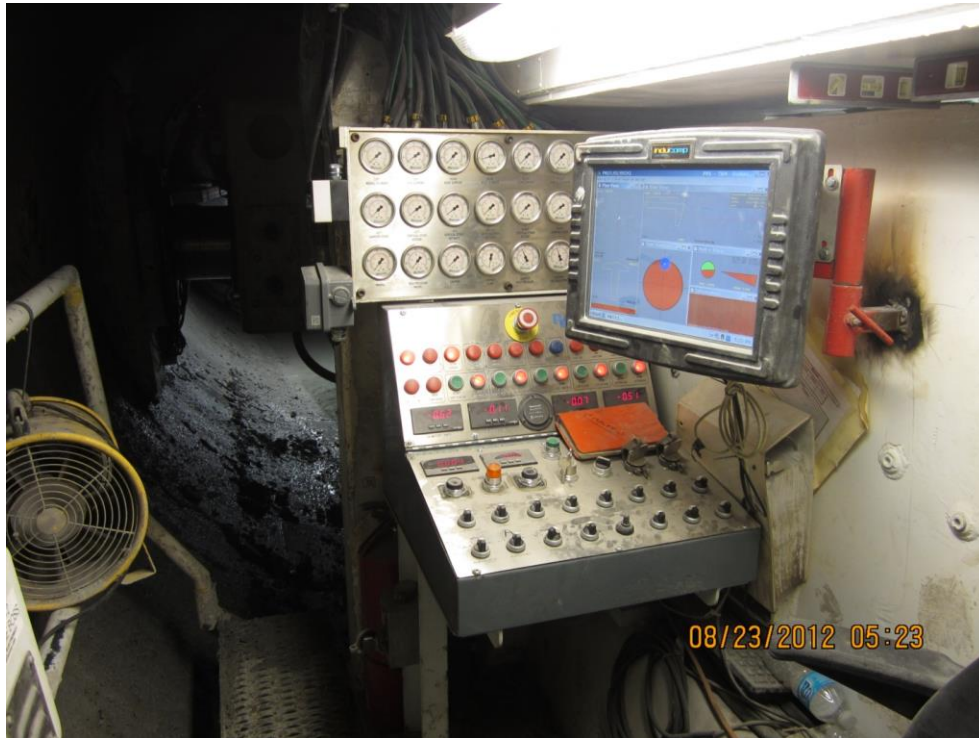
Operator's cab on the Reach #2 TBM.
