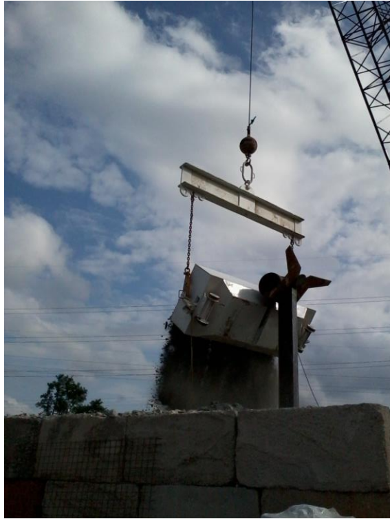
Dumping the muck on surface.
