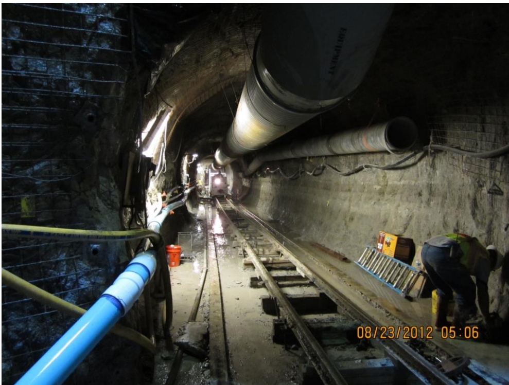
Full muck train arriving at the shaft.
