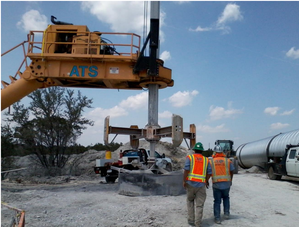
Figure 1.10. ATS Drilling beginning the drilling process at the WTP4 shaft location.
