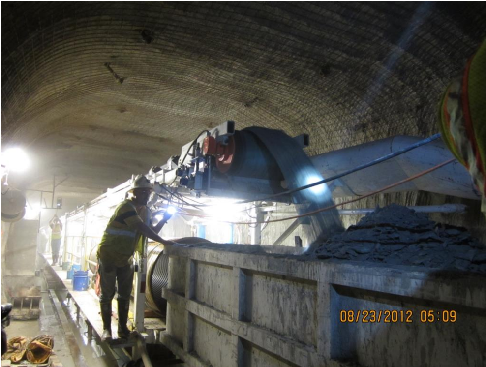
Filling up a muck car during TBM operations.
