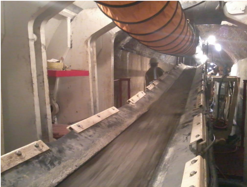
The conveyor belt inside the TBM can of Reach #1 during operations.
