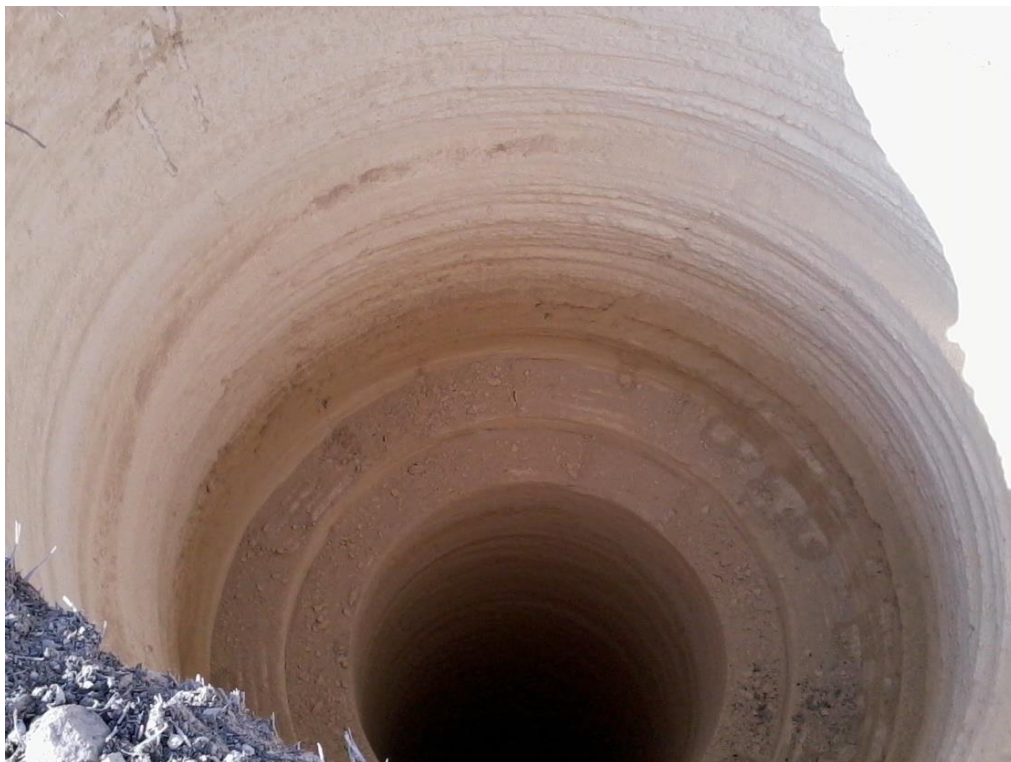
Figure 1.11. Drilled shaft at WTP4 shaft location.
