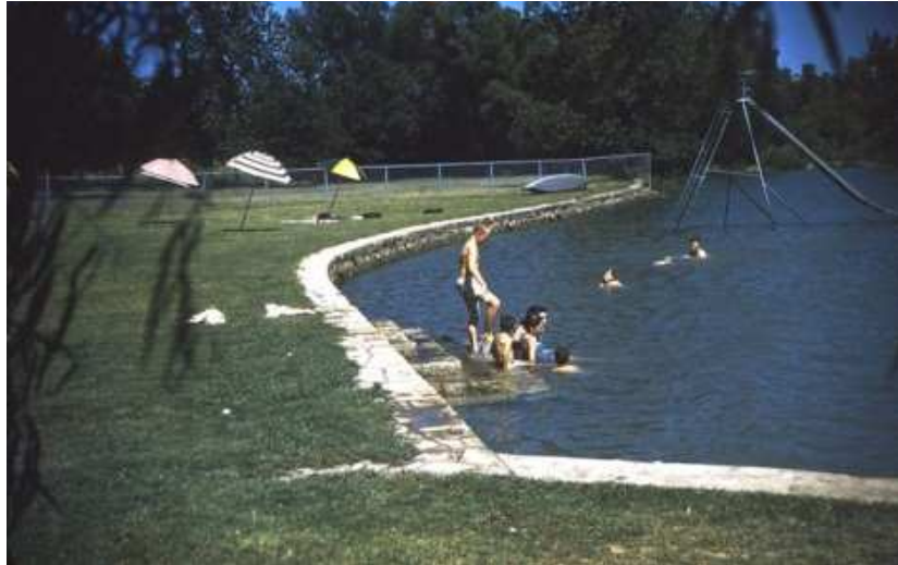
Figure 4.16 The original wall constructed by the CCC. This wall was constructed to prevent erosion and to maintain the lake's shore lines (Source: Dr. Pat Taylor @ UTA)
