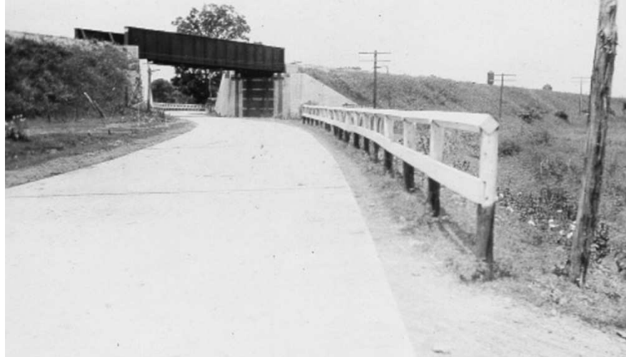
Figure 4.10 An earlier image of the Old Spanish Trail road. In this image the grass right-of-ways, tight curves, and lack of shoulders are evident. (Source: http://www.thc.state.tx.us/public/upload/preserve/national_register/final/Columbus%20OST%20NR.pdf )
