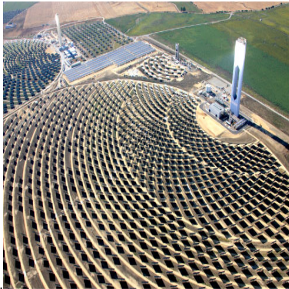
(a) Picture of a Power Tower[13]
