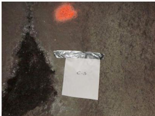
Figure 2.8 White Powder and Gel from Sulfate Reaction (Puppala 2010)
