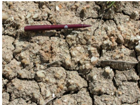
Figure 2.13 Gypsum Crystals Located in Drainage Wash Adjacent to the Roadway (Harris et al. 2006)
