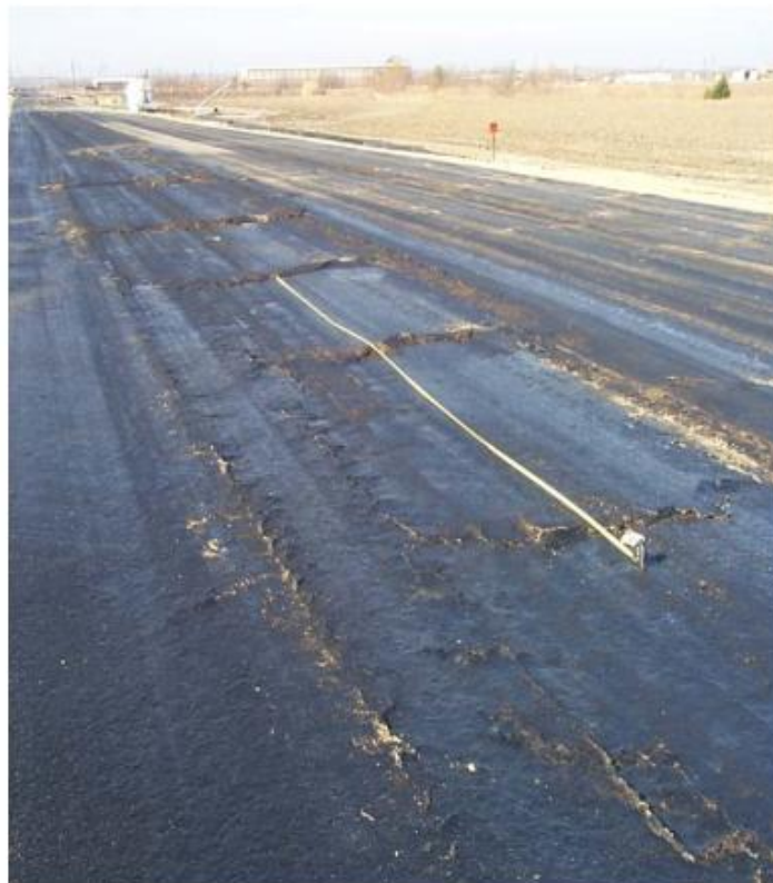
Figure 2.15 Heave Associated with US 67 near Midlothian, TX (Wimsatt 1999)
