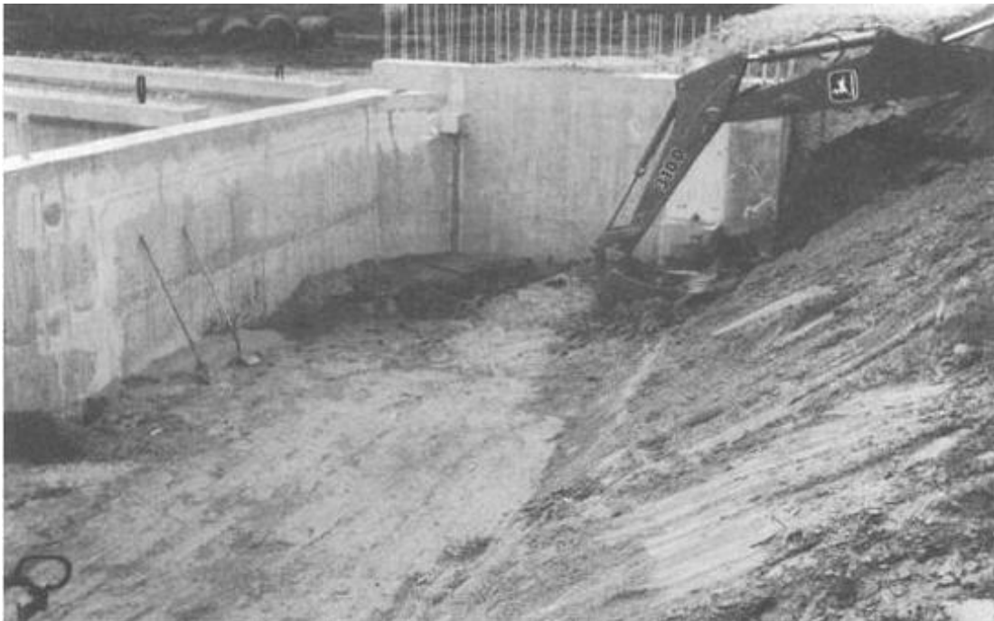
Figure 2.3 Excavation of backfill area at CLSM approach embankment (Snethen et al. 1998)
