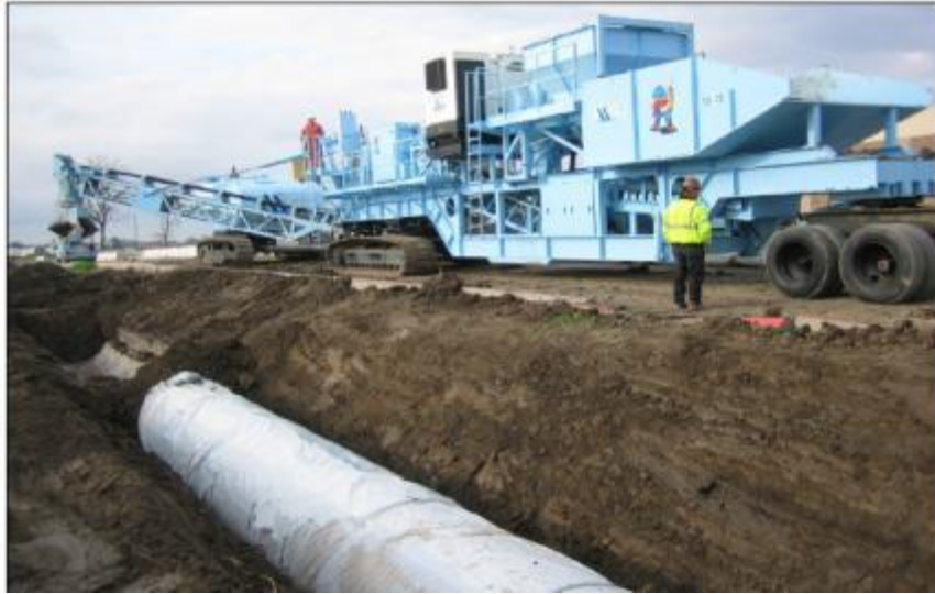
Figure 2.6 Placing of CLSM at test section (Finney et al. 2008)
