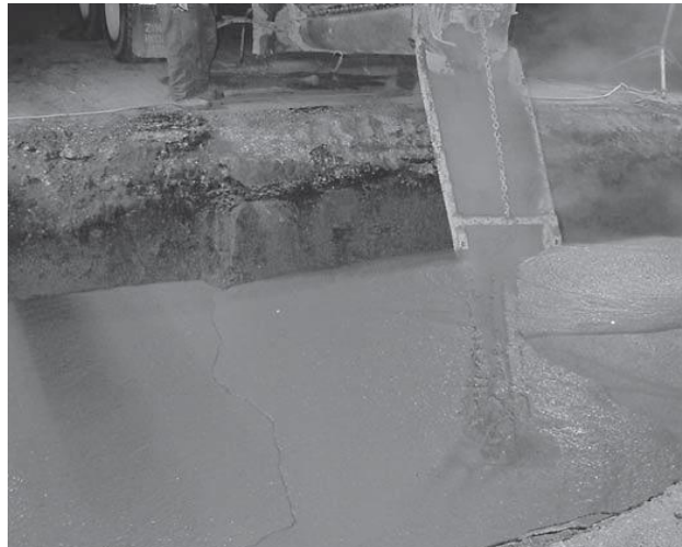
Figure 2.2 Placing rapid-setting CLSM for bridge approach (Du et al. 2006)
