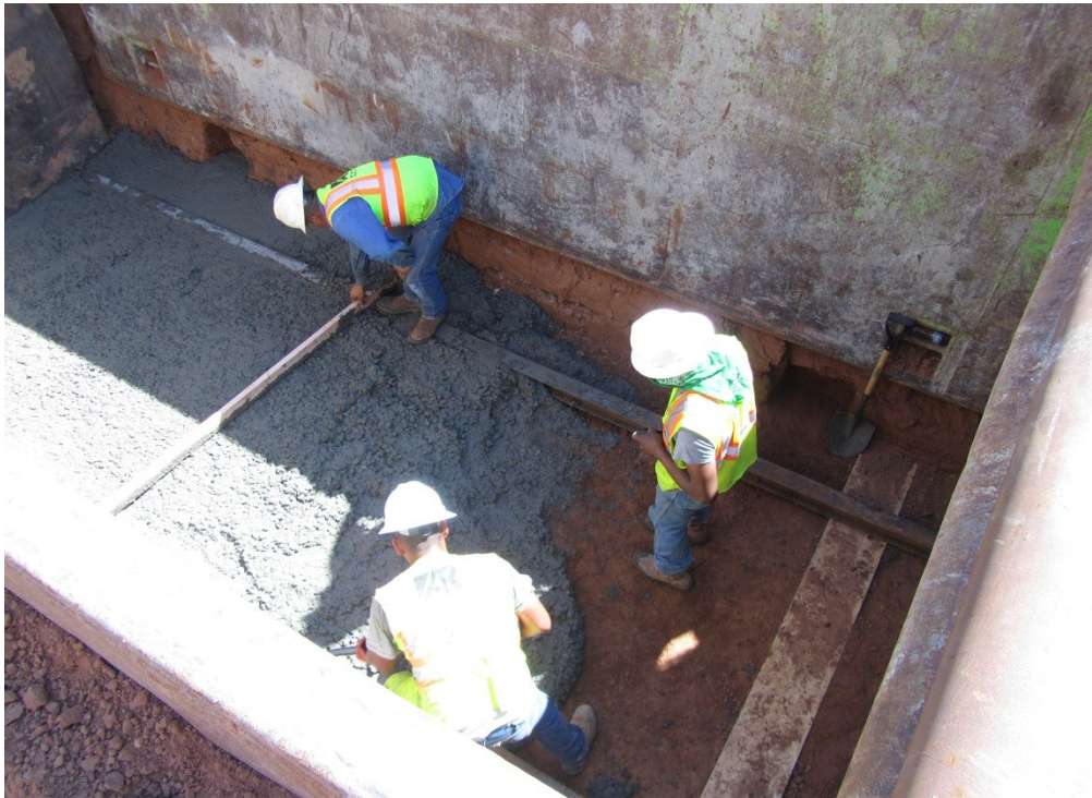
Pouring Concrete on Bottom of Jacking Pit
