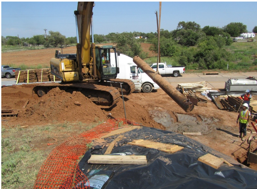
Setting up Jacking Frame
