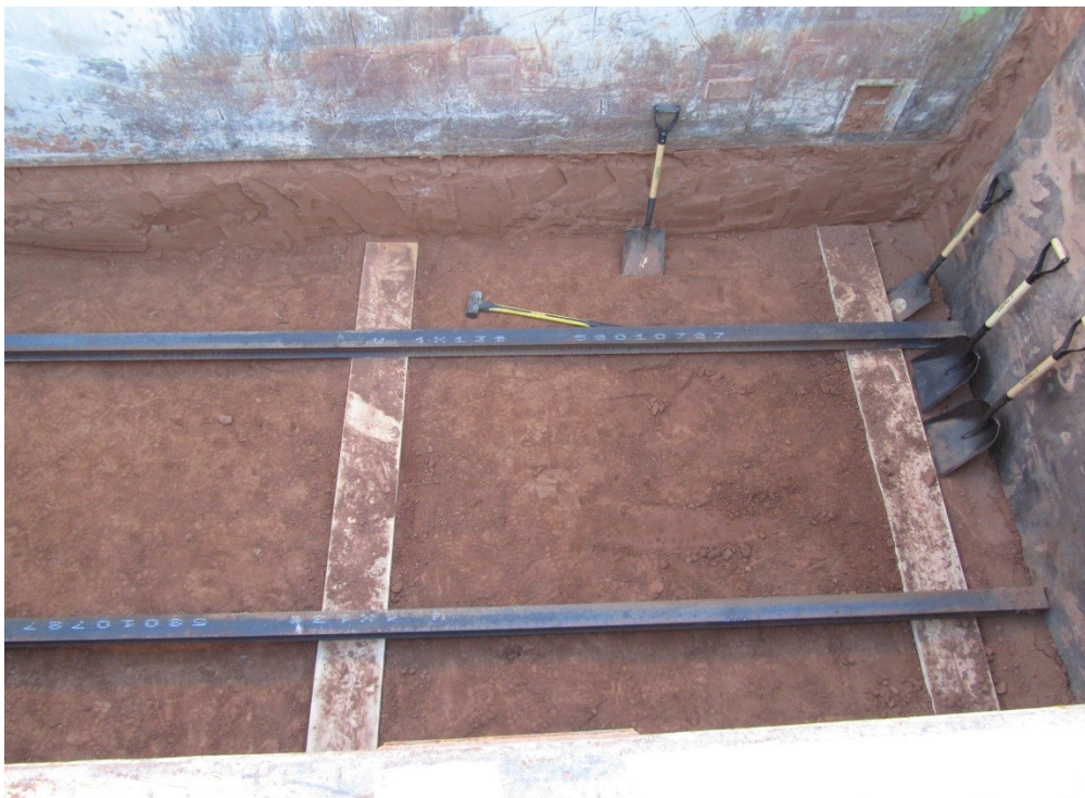
Leveling and Preparing Jacking Pit
