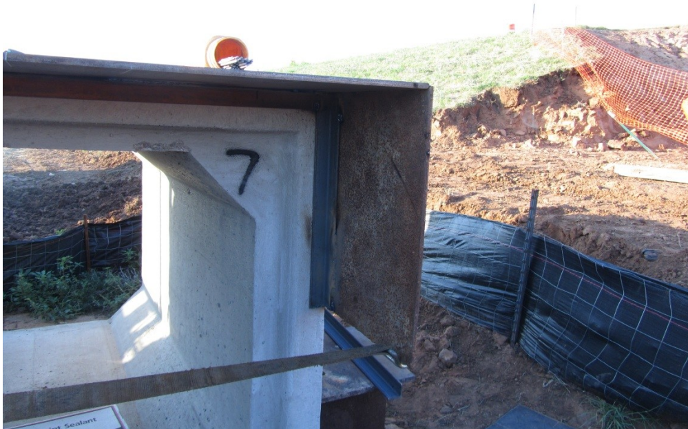
Preparing First Box and Shield
