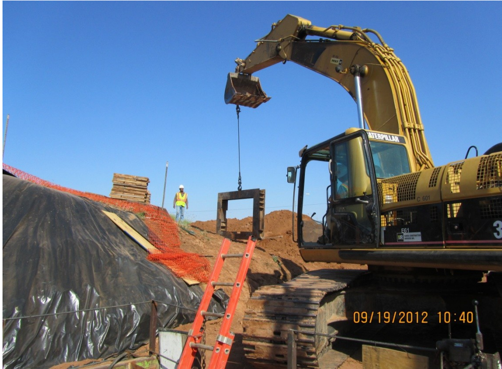
Setting up Jacking Frame
