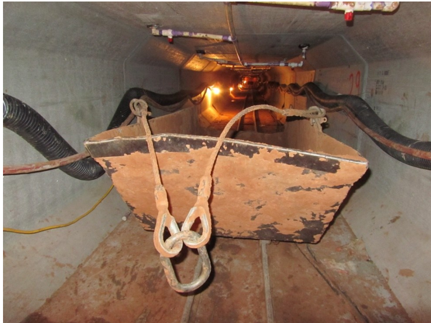
Figure 3.12 Empty Spoil Cart is Pulled Towards Face of the Tunnel
