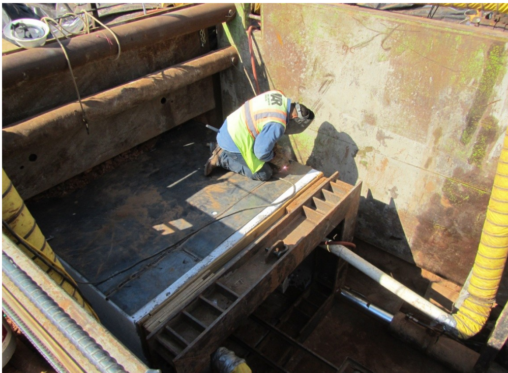
Start Jacking Boxes
