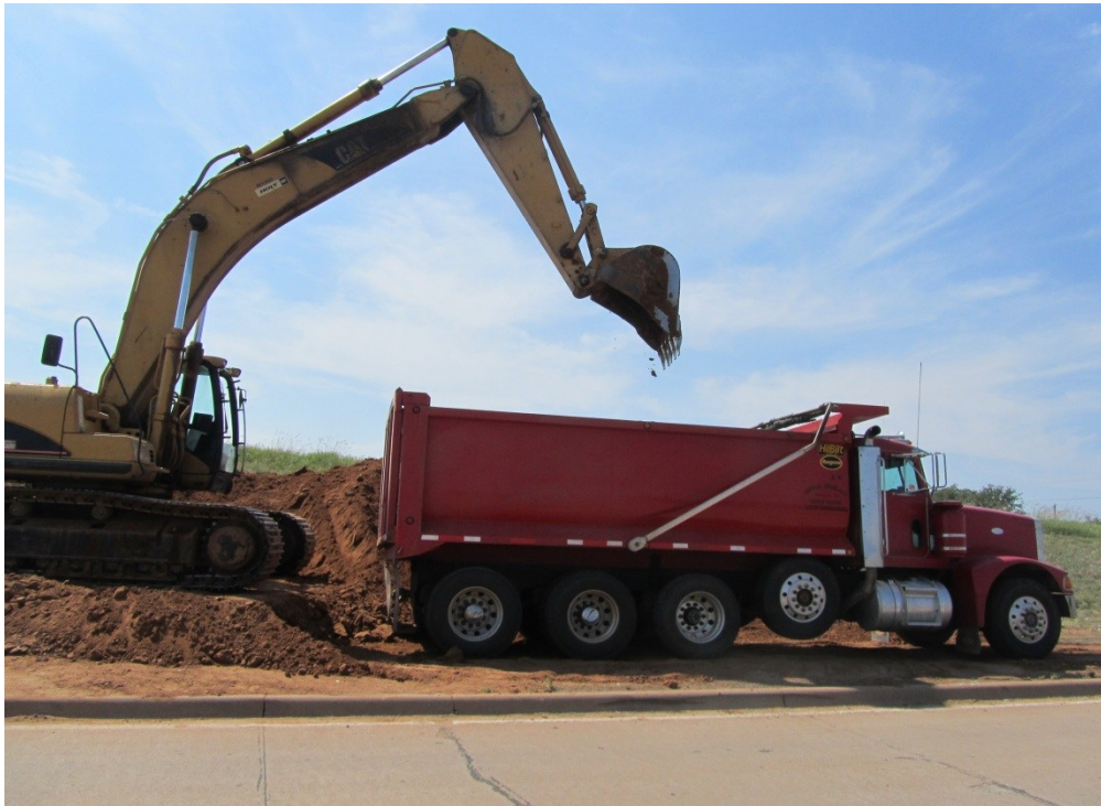
Truck Hauling Dirt from job Site
