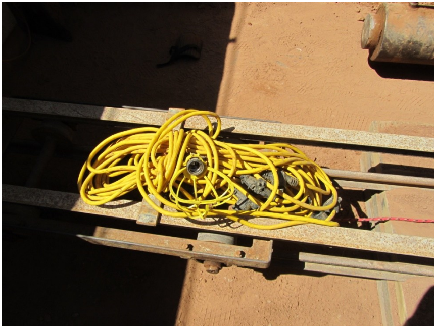
Figure 3.16 Cables and Rails Removed
