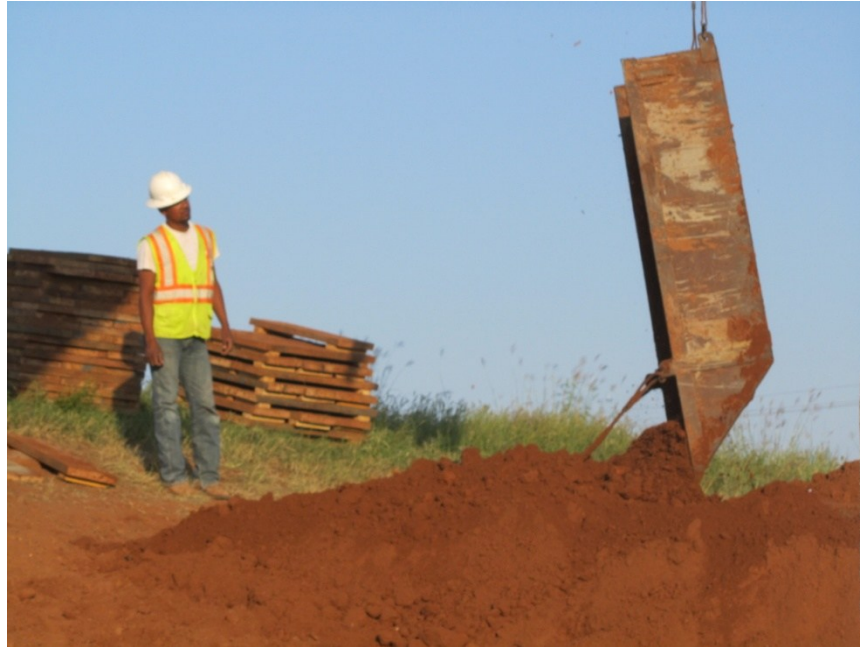
Figure 3.11 Crane Unloads Spoil Cart
