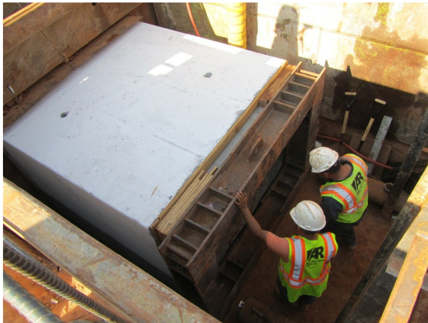
Figure 3.5 Labors Placing Jacking Frame
