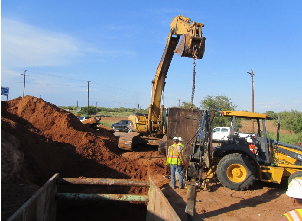
Placing Jacking Frame
