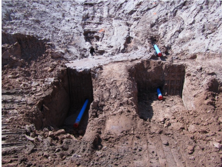
Figure 3.2119: Casings in Place
