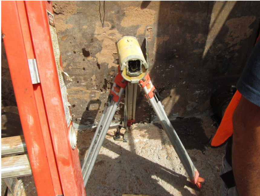
Figure 3.9 Laser for Grade and Alignment
