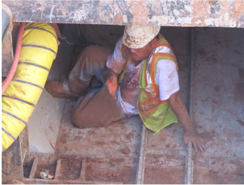
Figure 3.14 Labor Guides Jacking Operation
