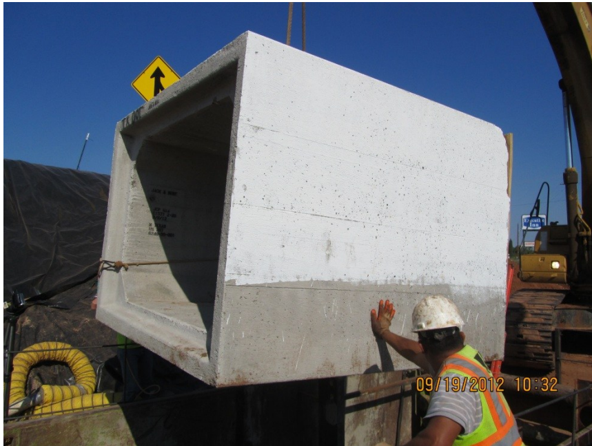
Figure 3.3 One Labor Helps to Place Culvert into the Launch Shaft
