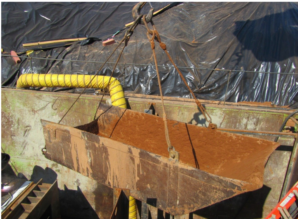
Rails and Dirt Removing Bucket
