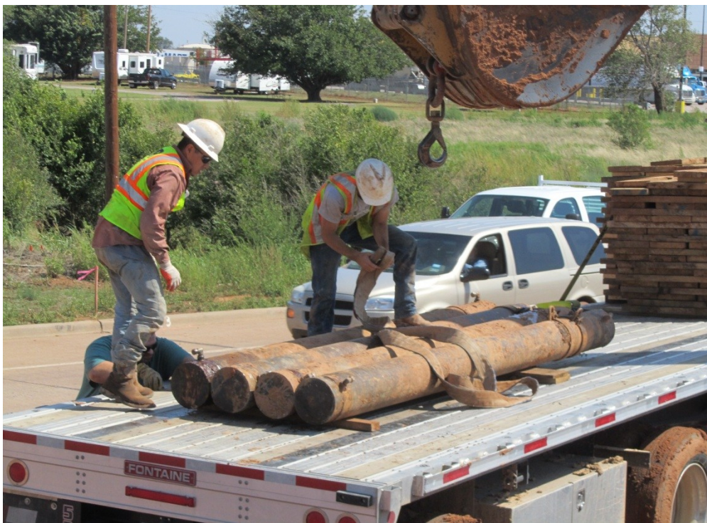
Loading Jacks in Truck
