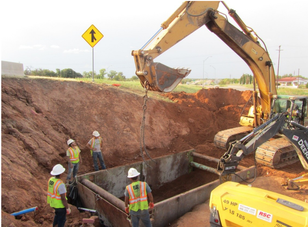
Demobilization, Removing Jacking Frame and Backfill
