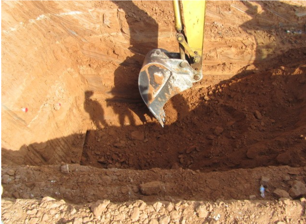
Excavation of Jacking Pit
