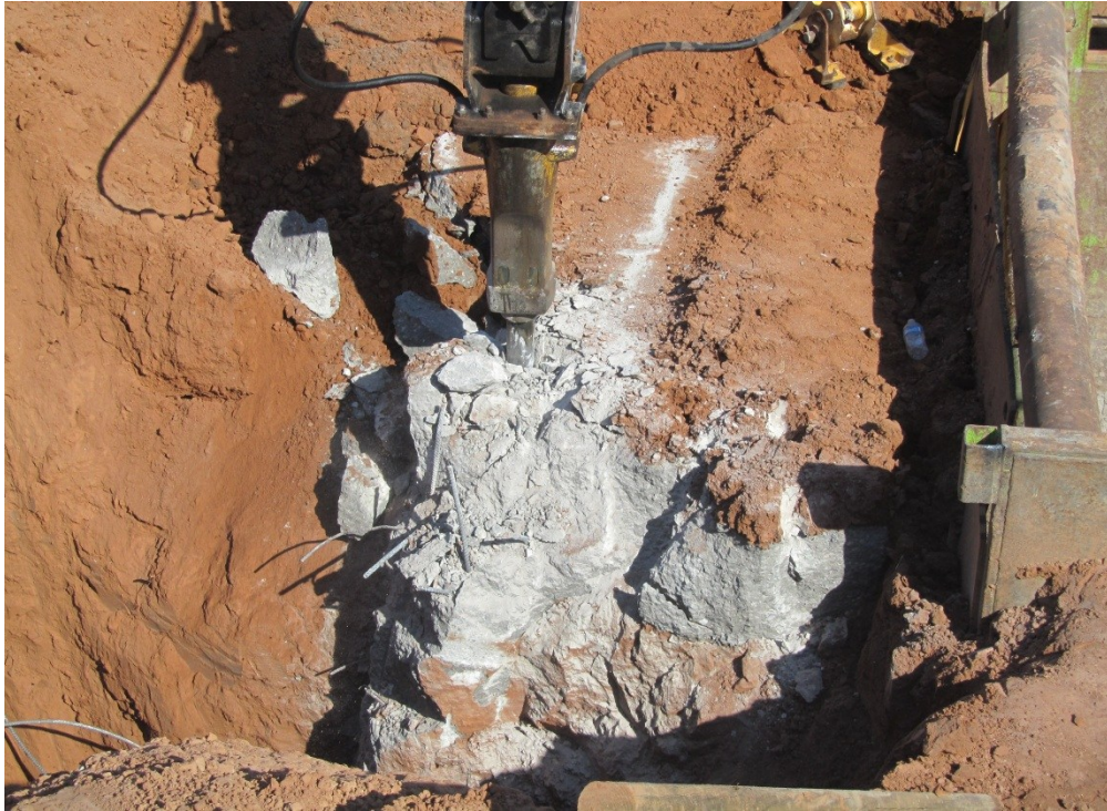
Demobilization, Removing Trust Wall
