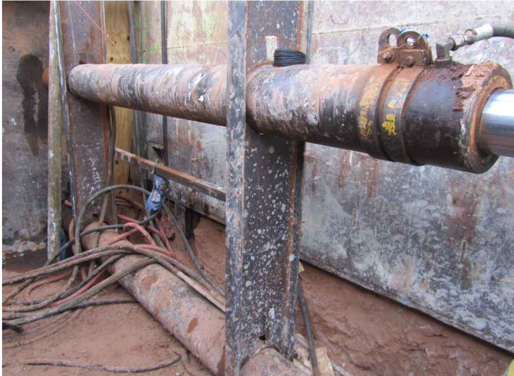
Jacks in Place
