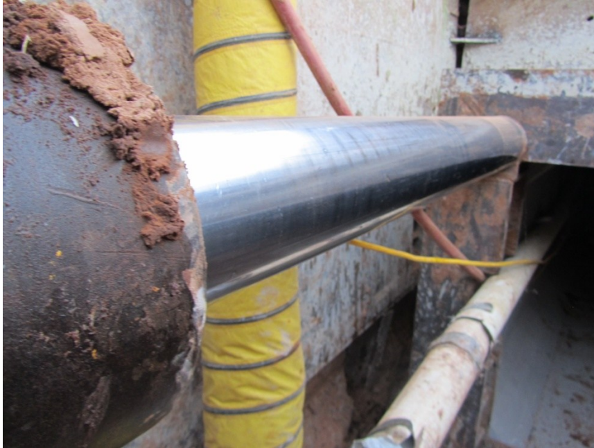
Figure 3.13 Four Jacks Pushing Box
