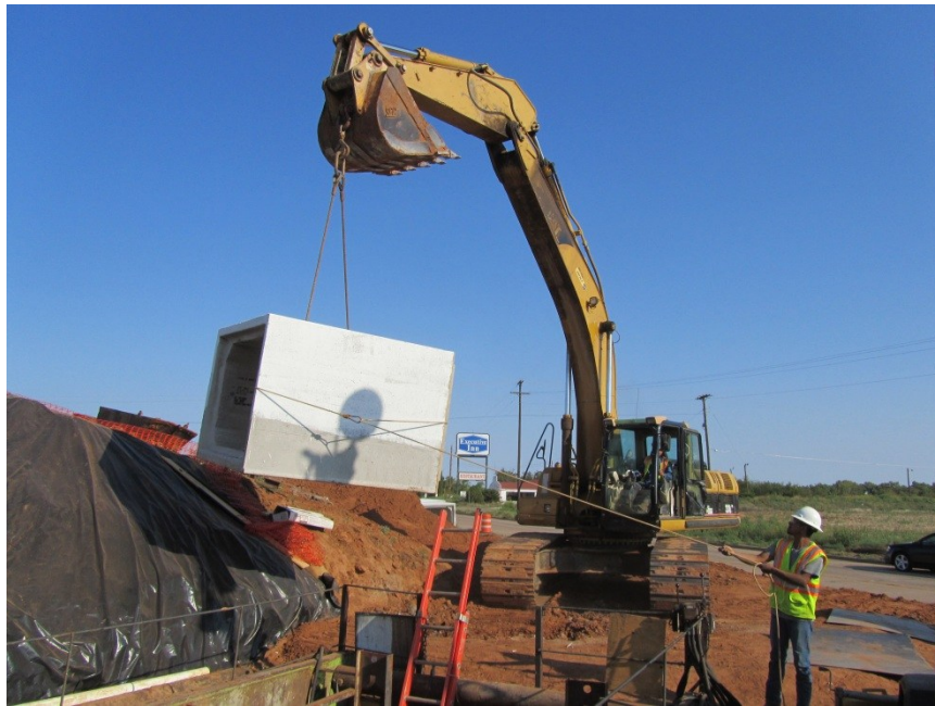
Figure 3.2 Crane Hoists a Culvert from Stockpile
