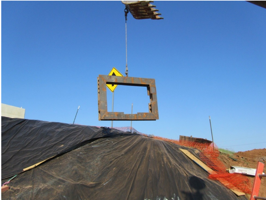
Figure 3.4 Crane Placing Jacking Frame into Launch Shaft
