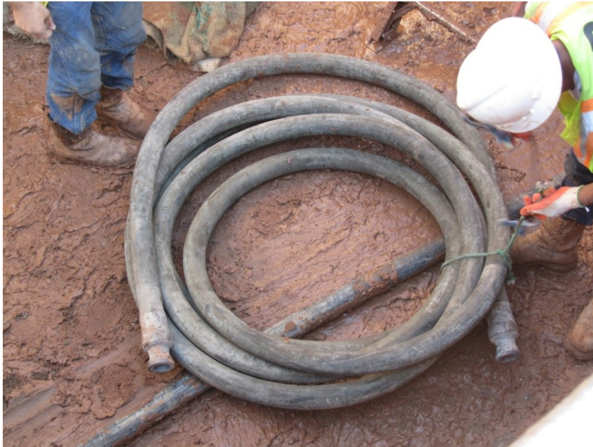
Figure 3.15 Labors Removing Bentonite Supply Hoses
