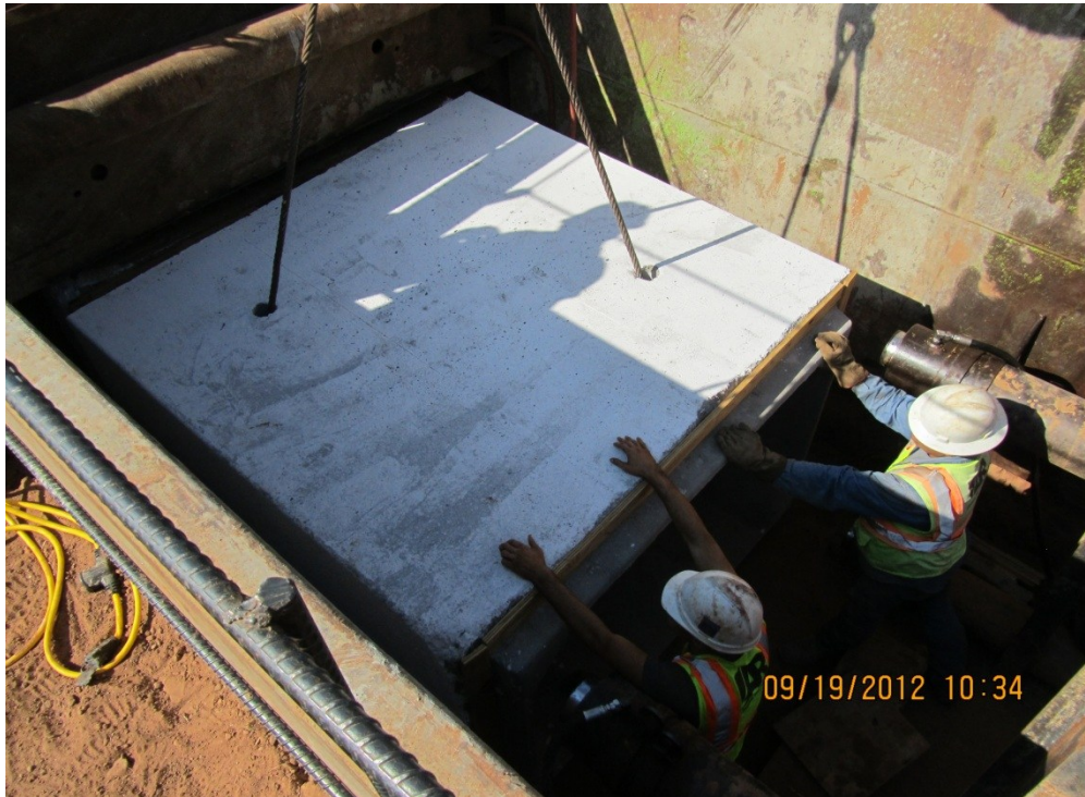
Installing Next Segment
