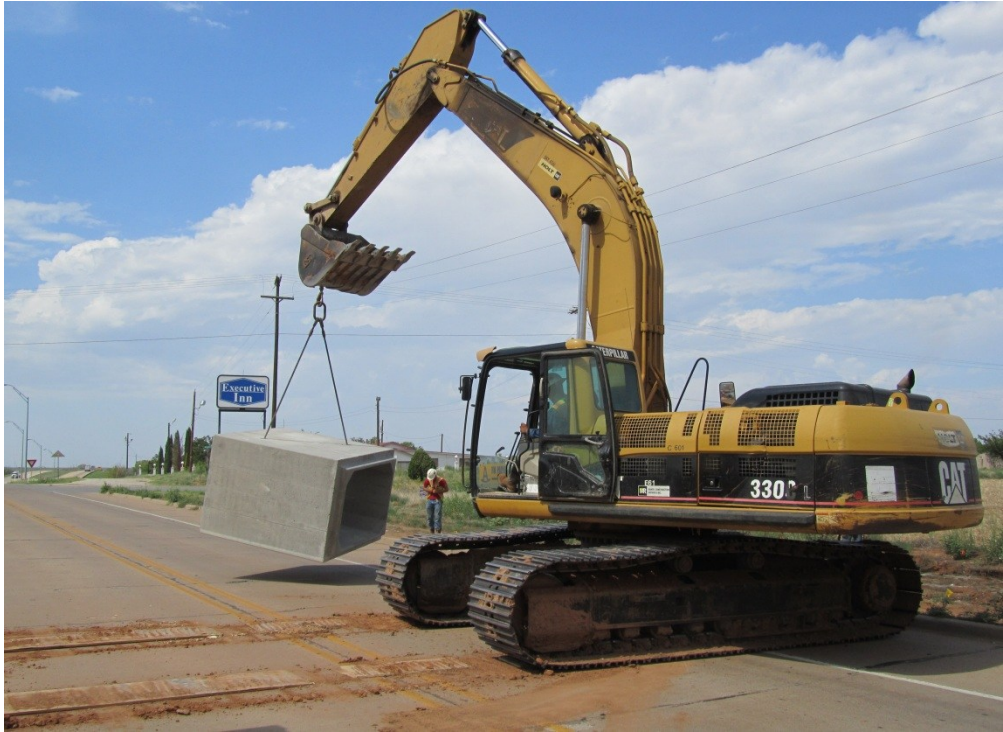
Bringing Culvert Box from Stockpile
