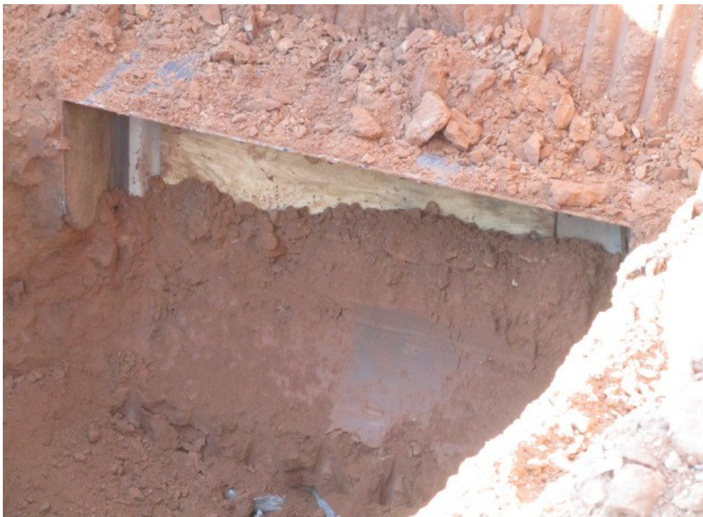
First Culvert Reaches the Other Side, End f Jacking Process
