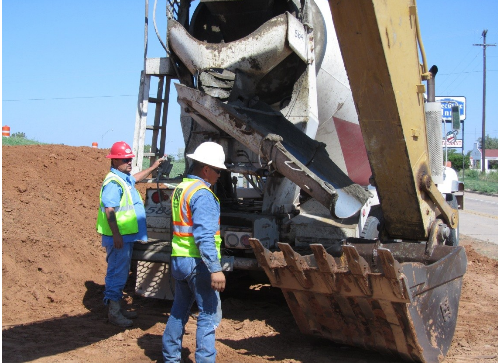
Pouring Concrete on Bottom of Jacking Pit
