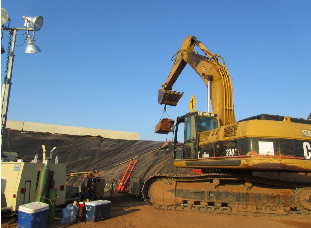
Removing Excavated Dirt
