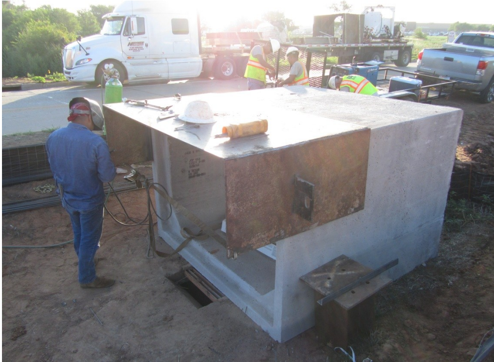
Preparing First Box and Shield
