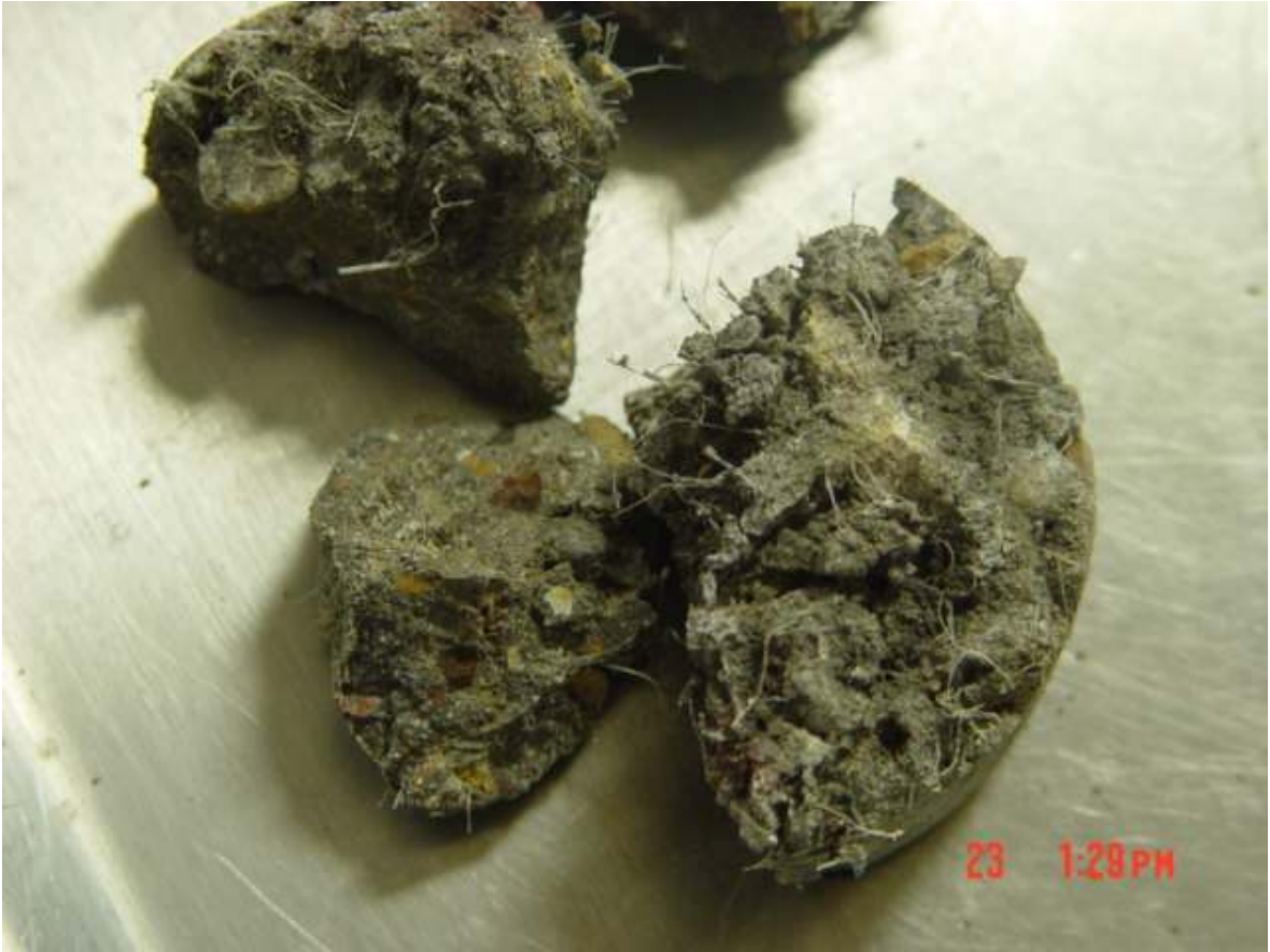
Figure A.2. Shotcrete Material from Tunnel Lining
