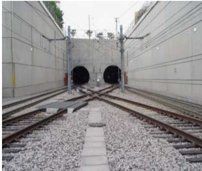
Figure 3.2 Picture of DART Tunnel Mined Portion
