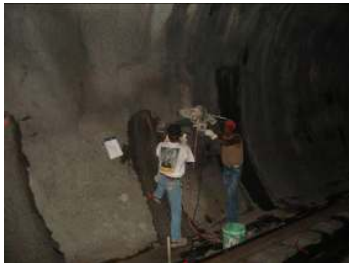
Figure 4.2 Coring of Rock Samples Using Carbide Rock Core Barrel
