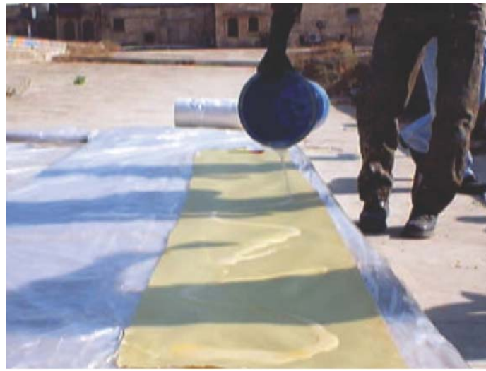
Figure 2.3 Application of Epoxy on FRP (Source: Verhulst et al, 2001)
