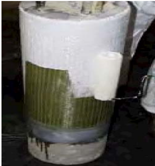
Figure 2.6 Painting FRP Wrapped Column (Source: Verhulst et al, 2001)
